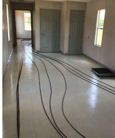
Field office interior
