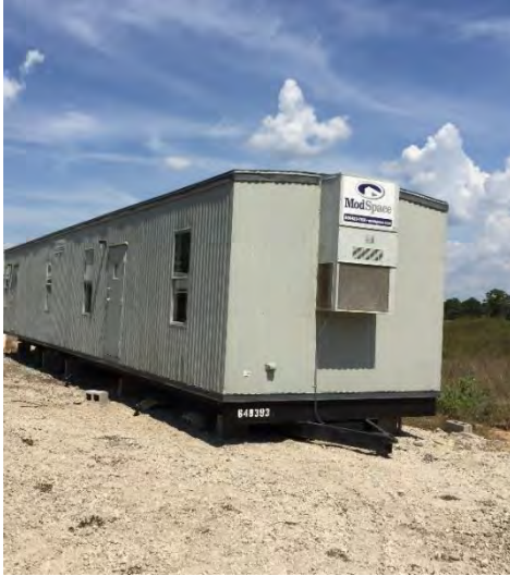
Field office exterior
