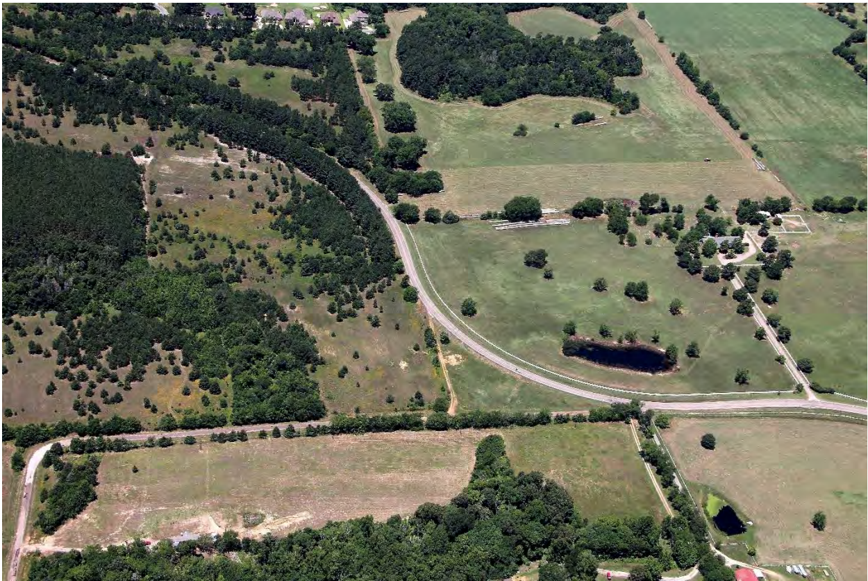
FIGURE 6: PROJECT AREA AT EXISTING FM 849
