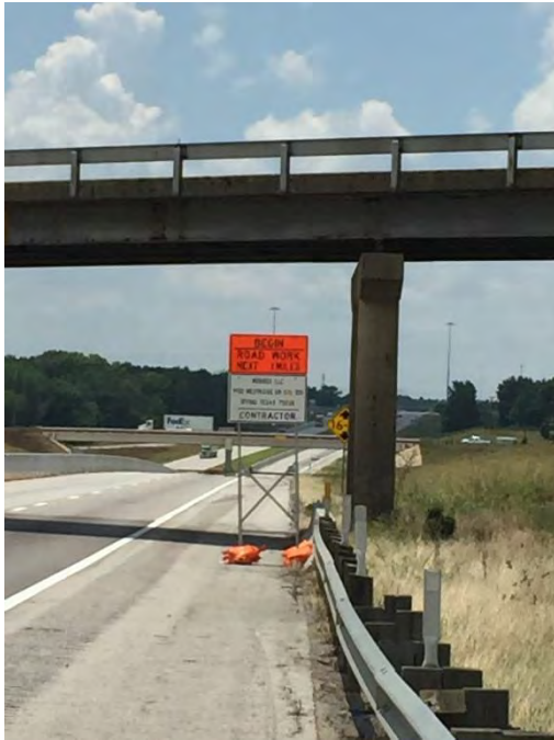
Work zone signage at I-20
