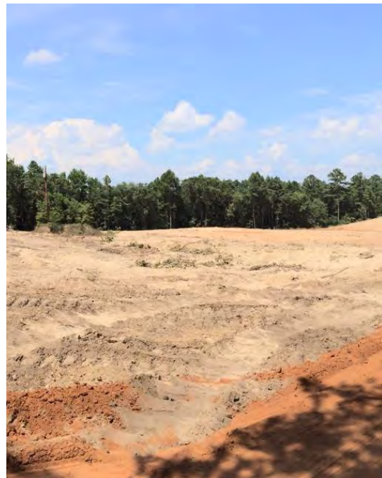
Clearing activities at sand pit
