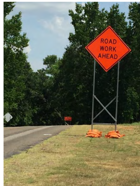
Work zone signage along CR 431
