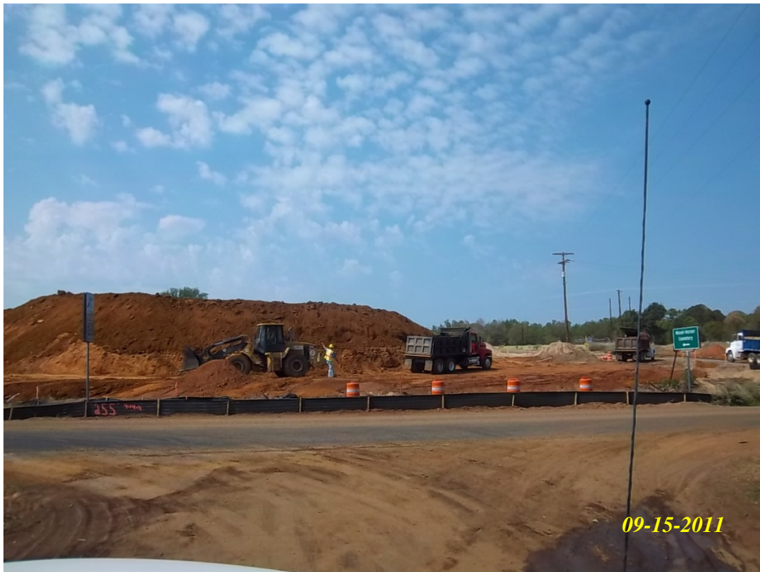
Toll 49 Segment 3B – FM 724 south embankment for Bridge abutment construction
