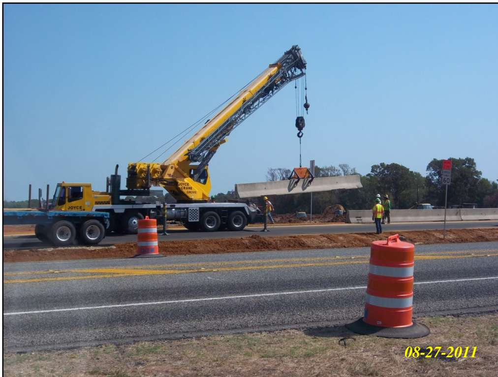
Toll 49 Segment 3B –SH 64 detour setting of the concrete traffic barriers
