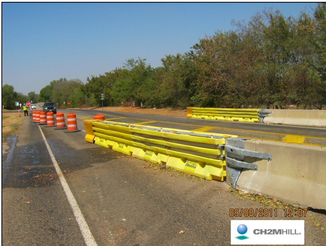
Toll 49 Segment 3B –SH 64 Crash Impact Attenuators
