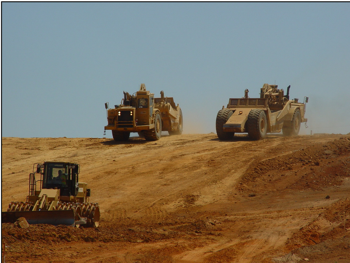
Scrapper Operations in Cut South of Indian Creek
