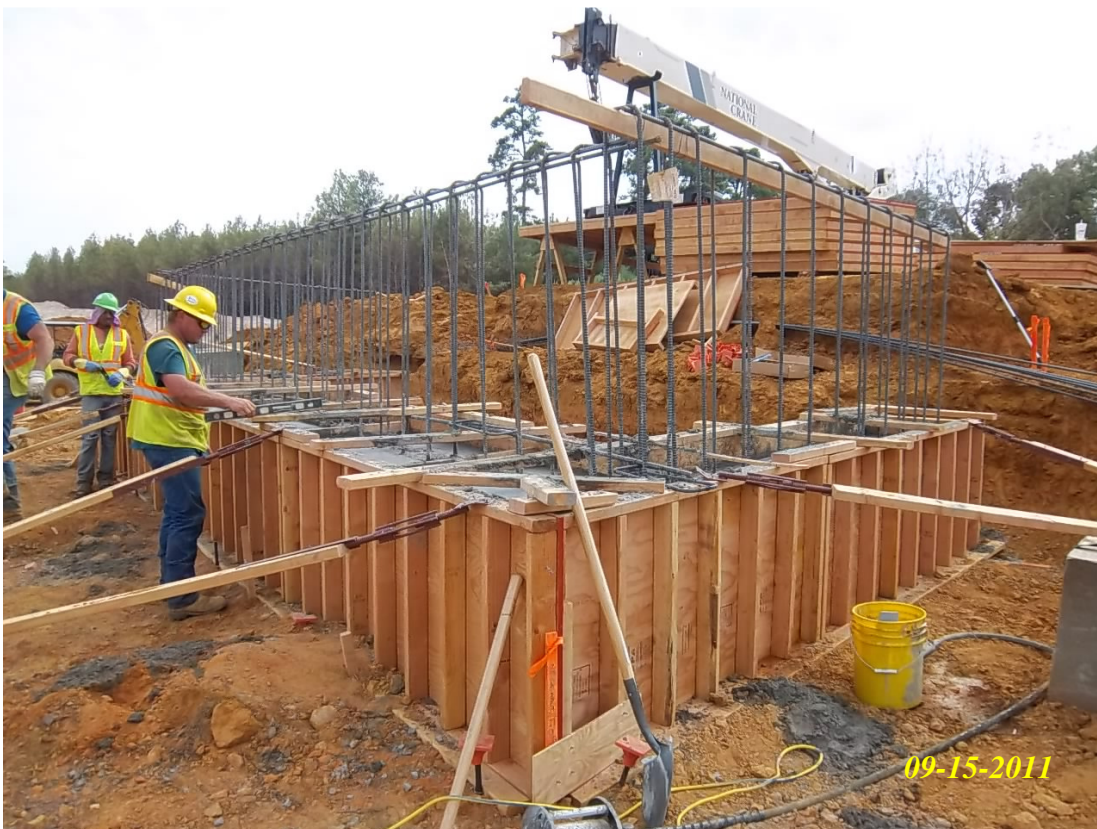
Toll 49 Segment 3B – Abutment cap concrete pour finishing up a leveling beaming seat
