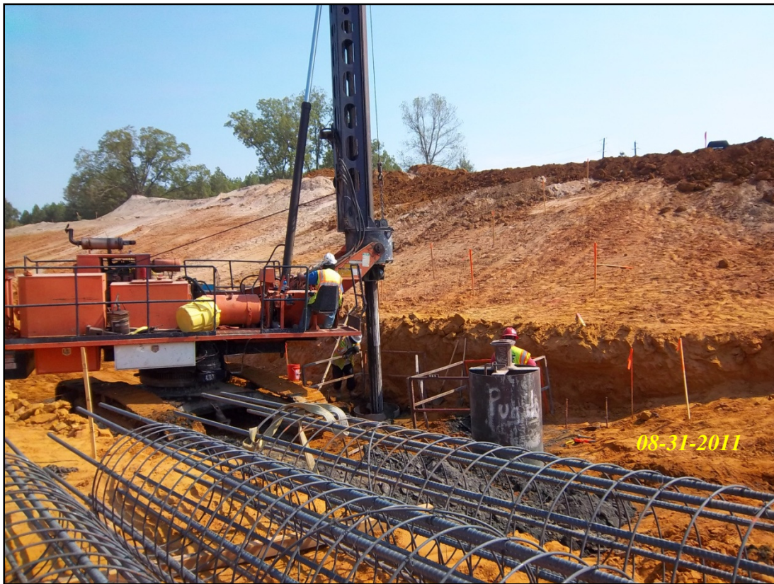
Toll 49 Segment 3B – Drilling for the foundation shaft at CR 1145 Bridge
