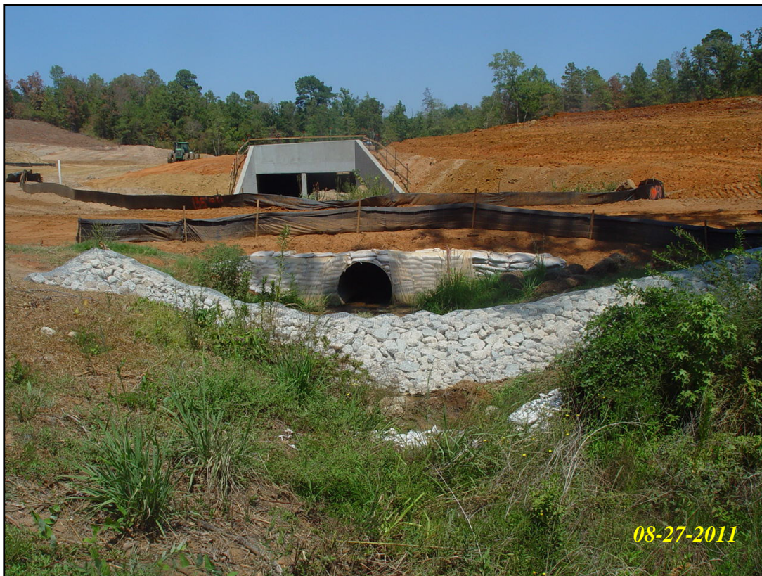
Toll 49 Segment 3B – Indian Creek downstream erosion control measures
