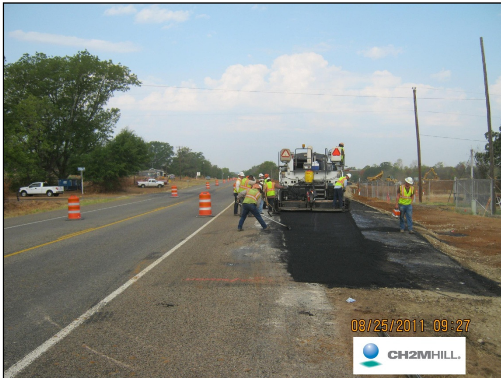
Toll 49 Segment 3B – Asphalt pavement lay down operations on SH 64 detour
