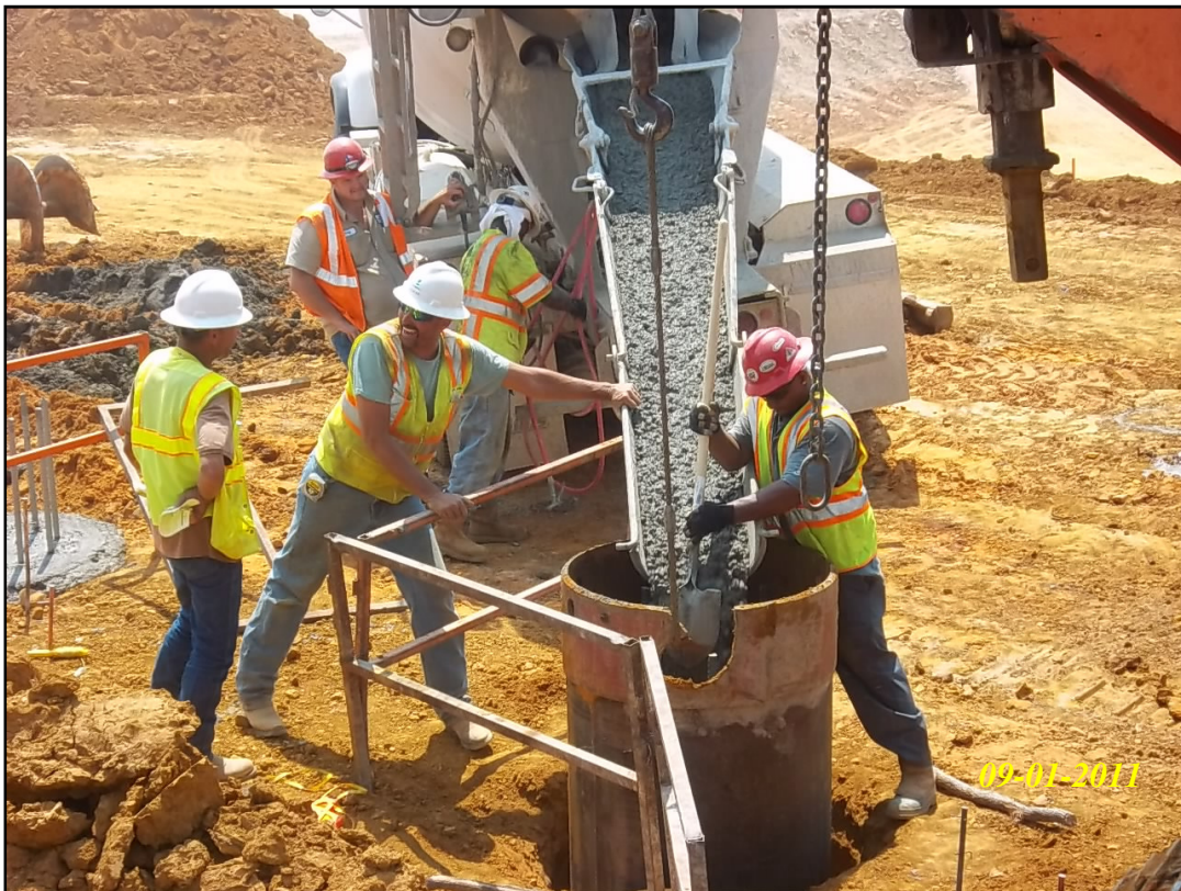
Toll 49 Segment 3B –Drilled shaft concrete pour for CR 1145 Bridge
