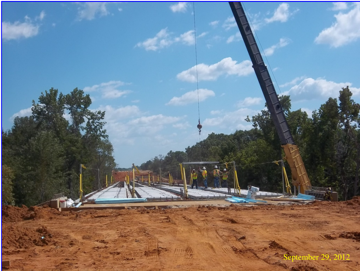
Setting Panels at Black Fork Creek Bridge
