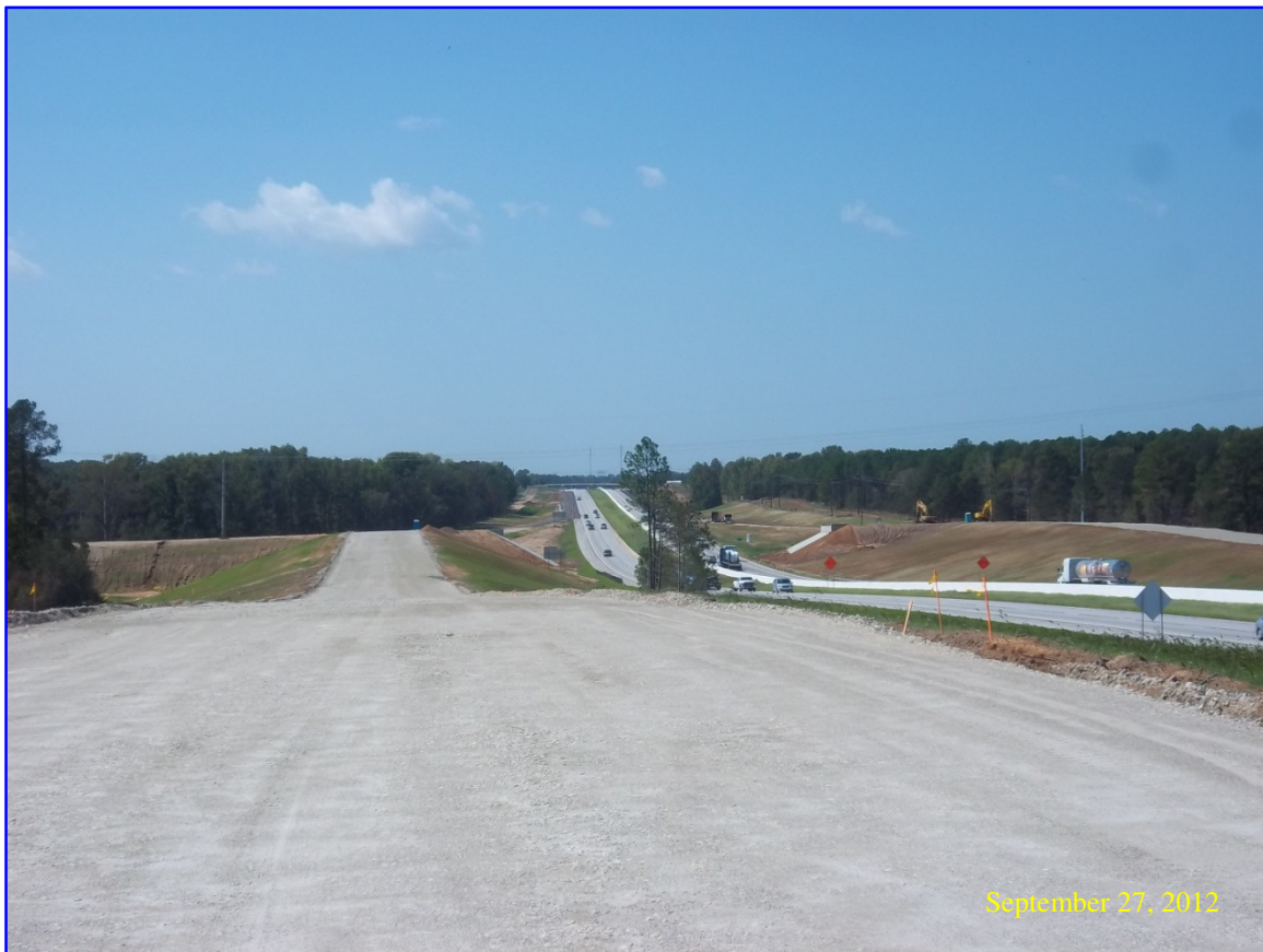
Flex Base Placement at CR 411 and I-20 Looking West
