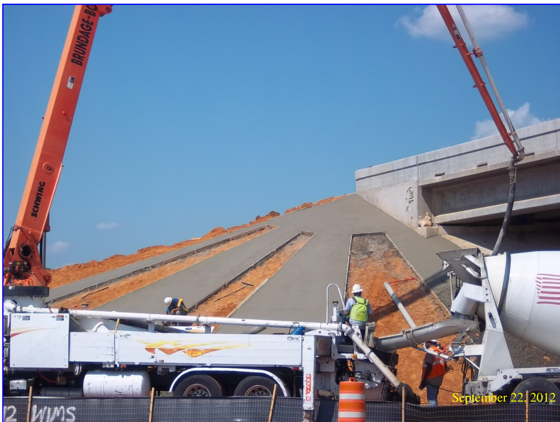
Concrete Rip Rap Construction
