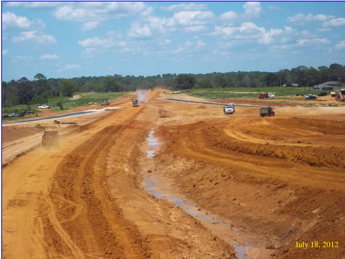
Roadway Grading North of SH 64
