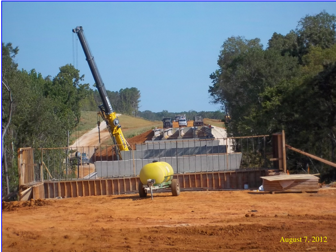
Setting Girders at Black Fork Creek Bridge
