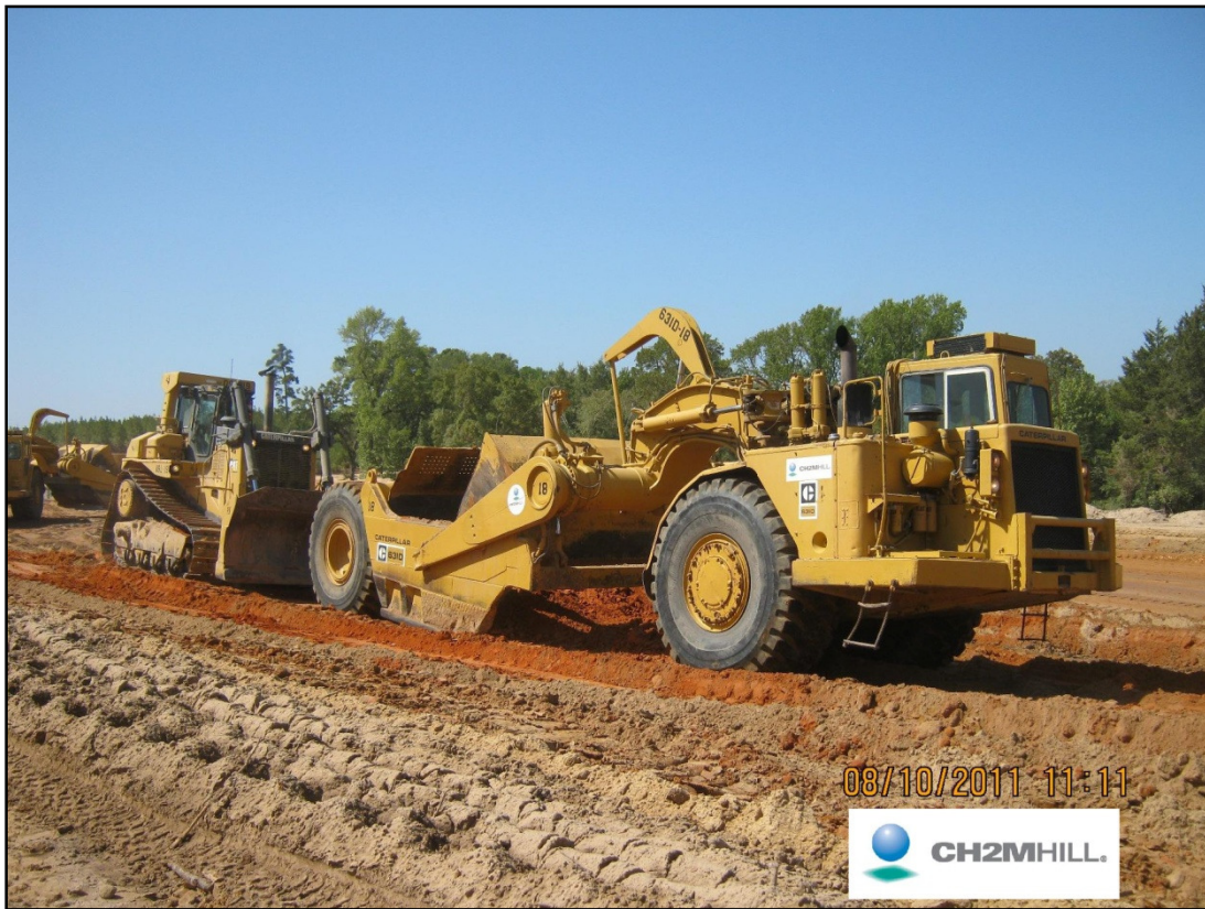
Toll 49 Segment 3B – Scraper Operation (picture courtesy of CH2M Hill)
