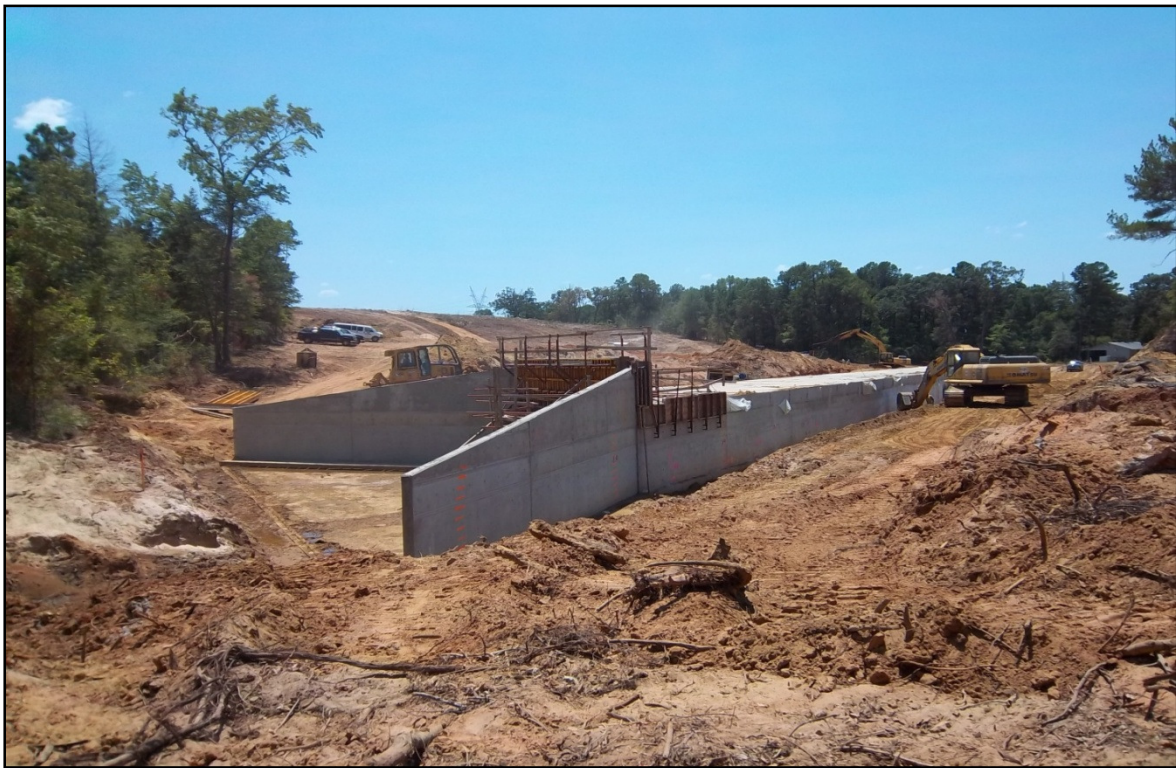
Toll 49 Segment 3B – Near Completion Preparing for Backfill of box Culvert at Indian Creek
