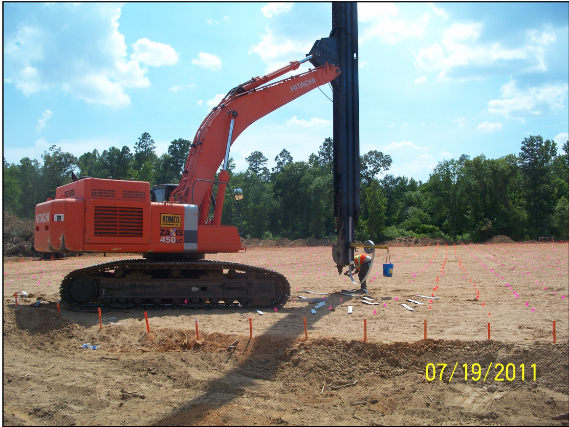
Installation of wick drains near Indian Creek.
