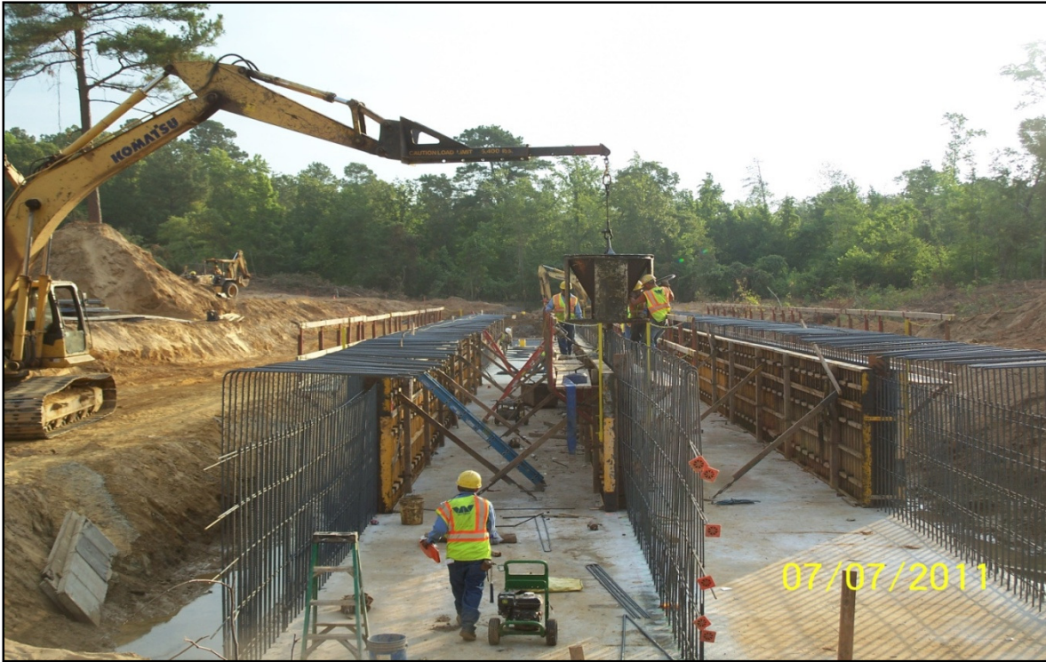
Toll 49 Segment 3B – Wall Pours for Box Culvert at Indian Creek
