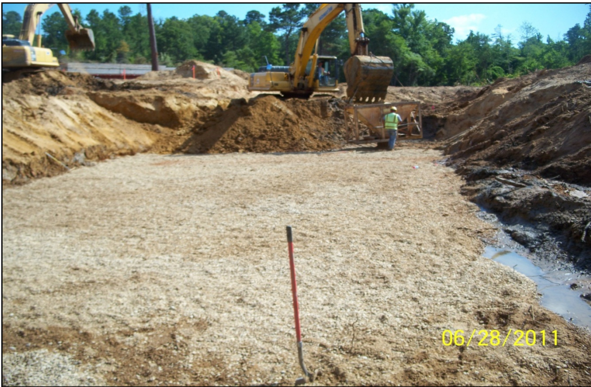
Toll 49 Segment 3B – Soil Preparation for Box Culvert at Indian Creek
