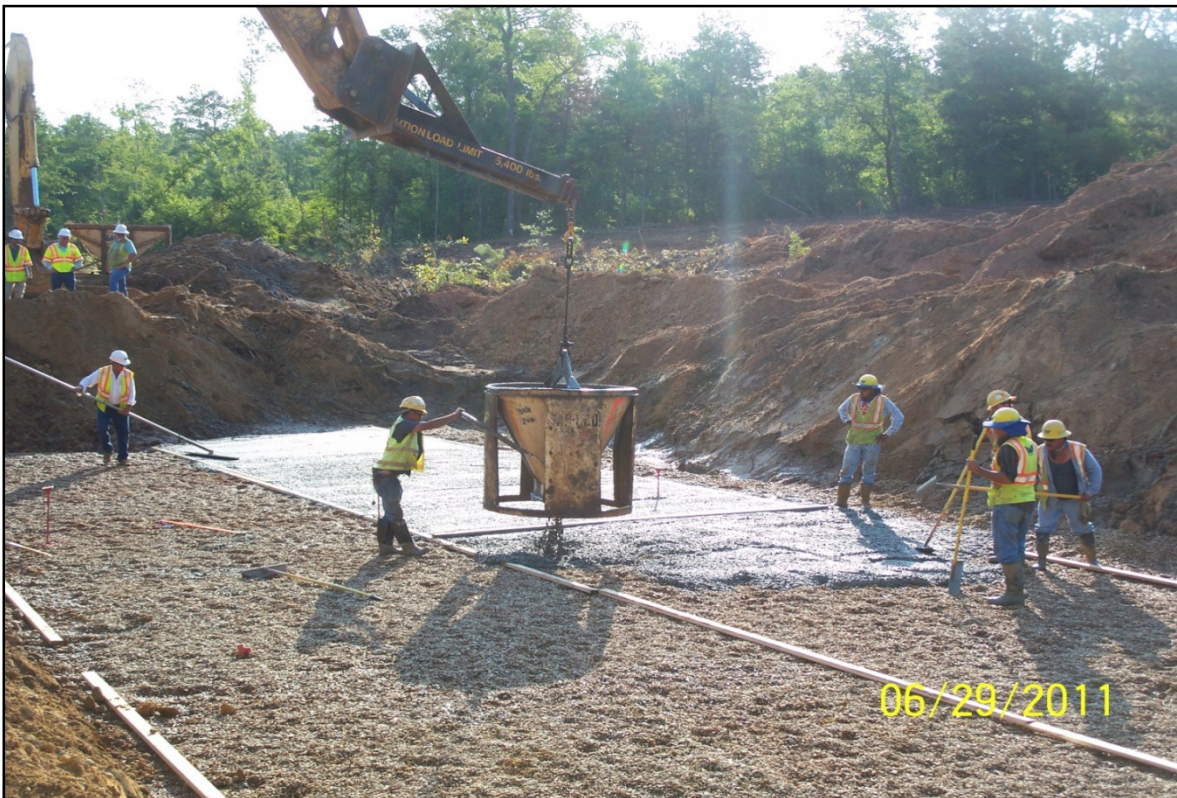
Toll 49 Segment 3B – Concrete Seal Slab Pour for Box Culvert at Indian Creek
