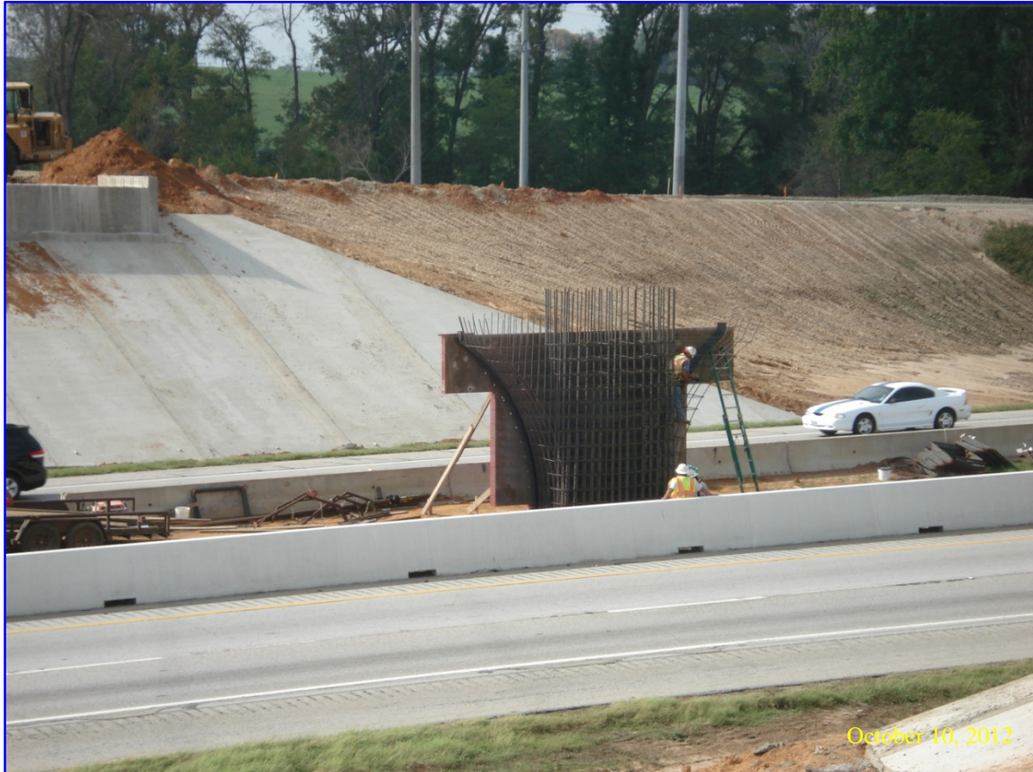
Toll 49 at I-20 Bridge Center Bent Cap Being Built
