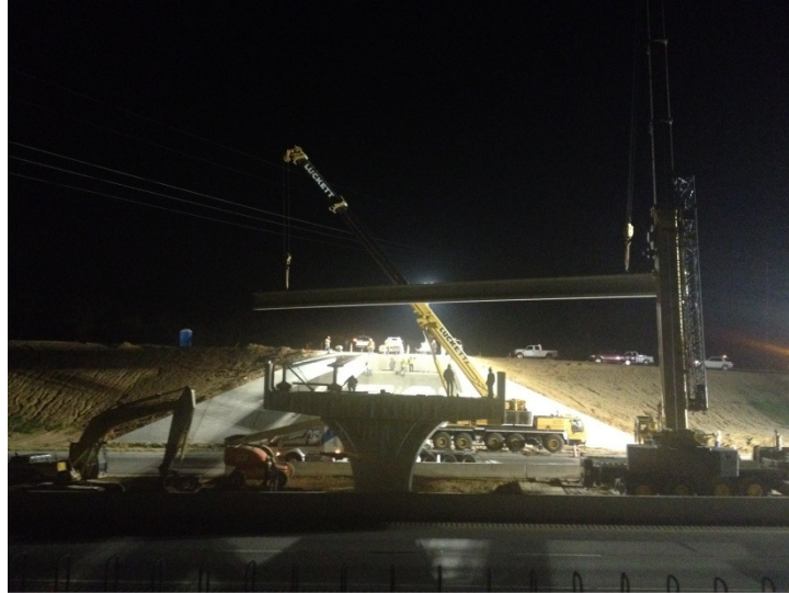
Figure 1 Looking South onto Toll 49 at I-20 Bridge Girder Set
