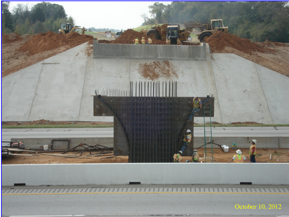
Looking South onto Toll 49 at I-20 Bridge Center Bent Cap Being Built
