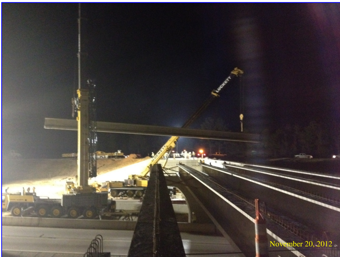
Looking North from Toll 49 at I-20 Bridge Girder Set
