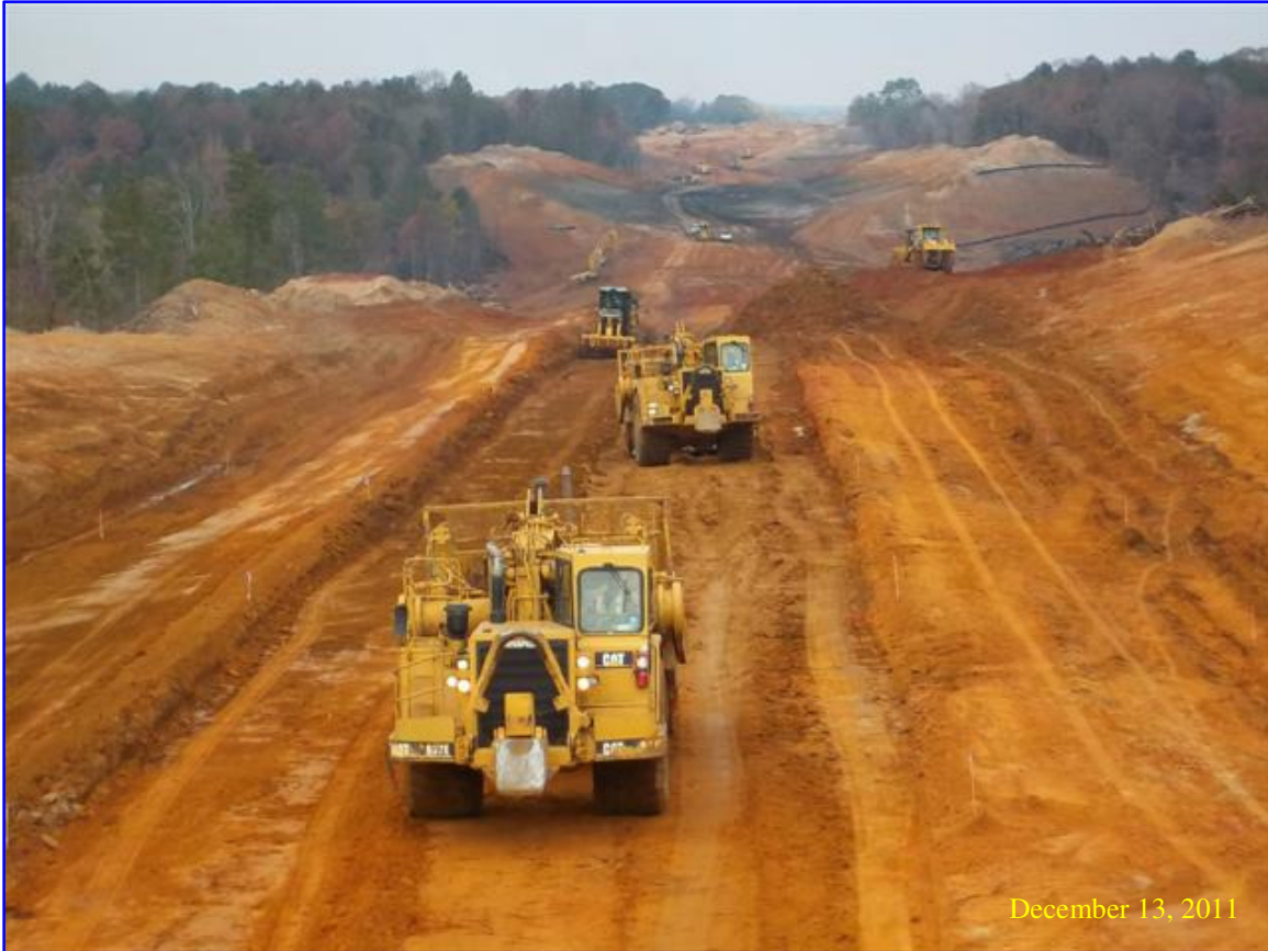
Finish grading operations looking north from CR 1145 Bridge.
