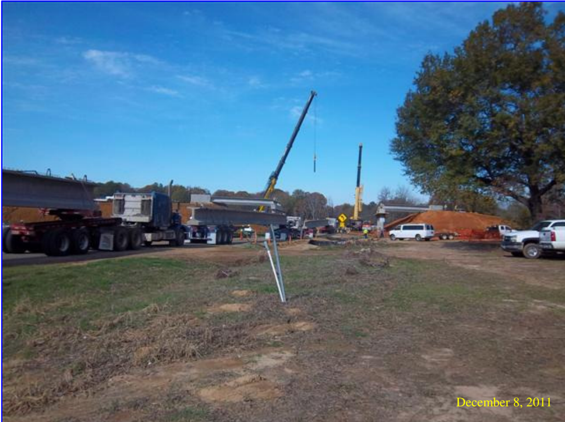
Pre-stressed Concrete Beams waiting placement at FM 724 bridge.
