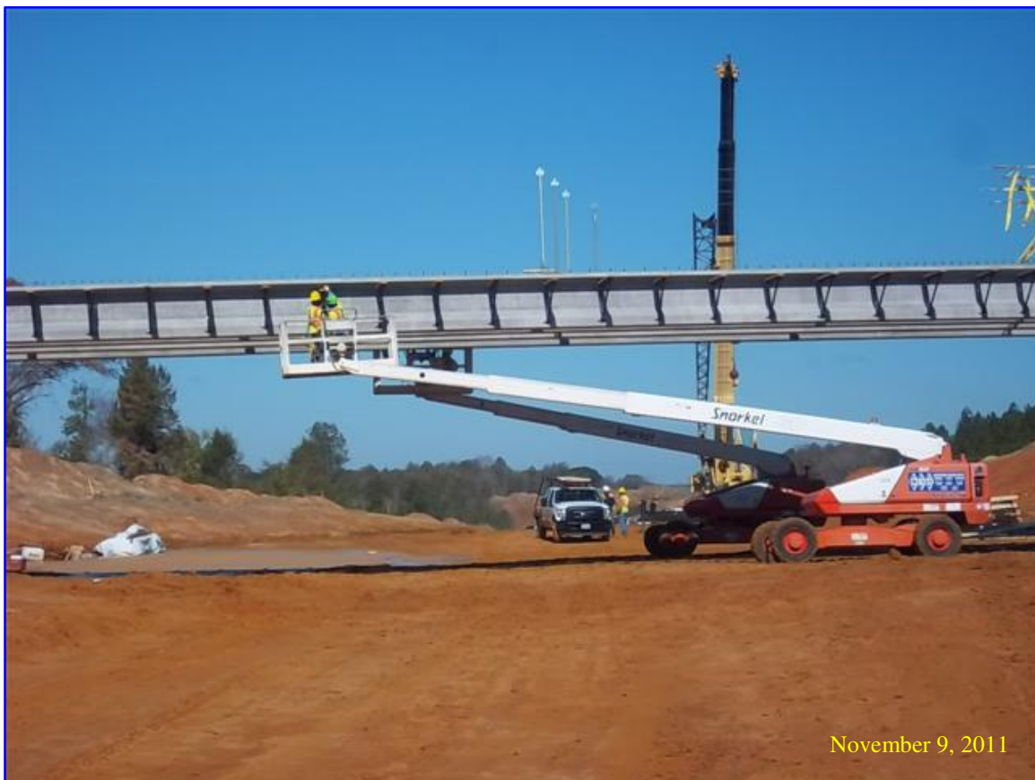
Installation of bridge slab overhang forms for CR 1145 bridge.
