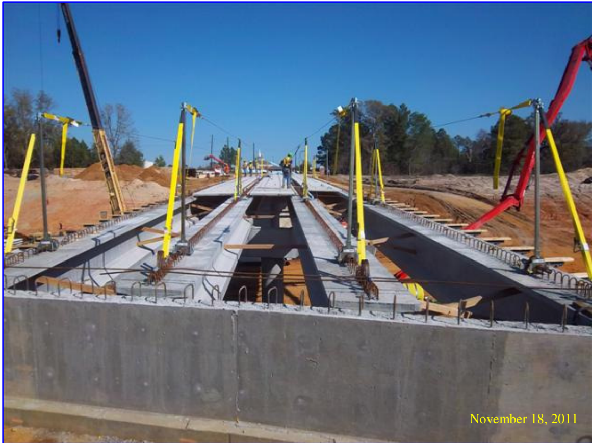
Placement of Pre-stressed Concrete Deck Panels on CR 1145 bridge.
