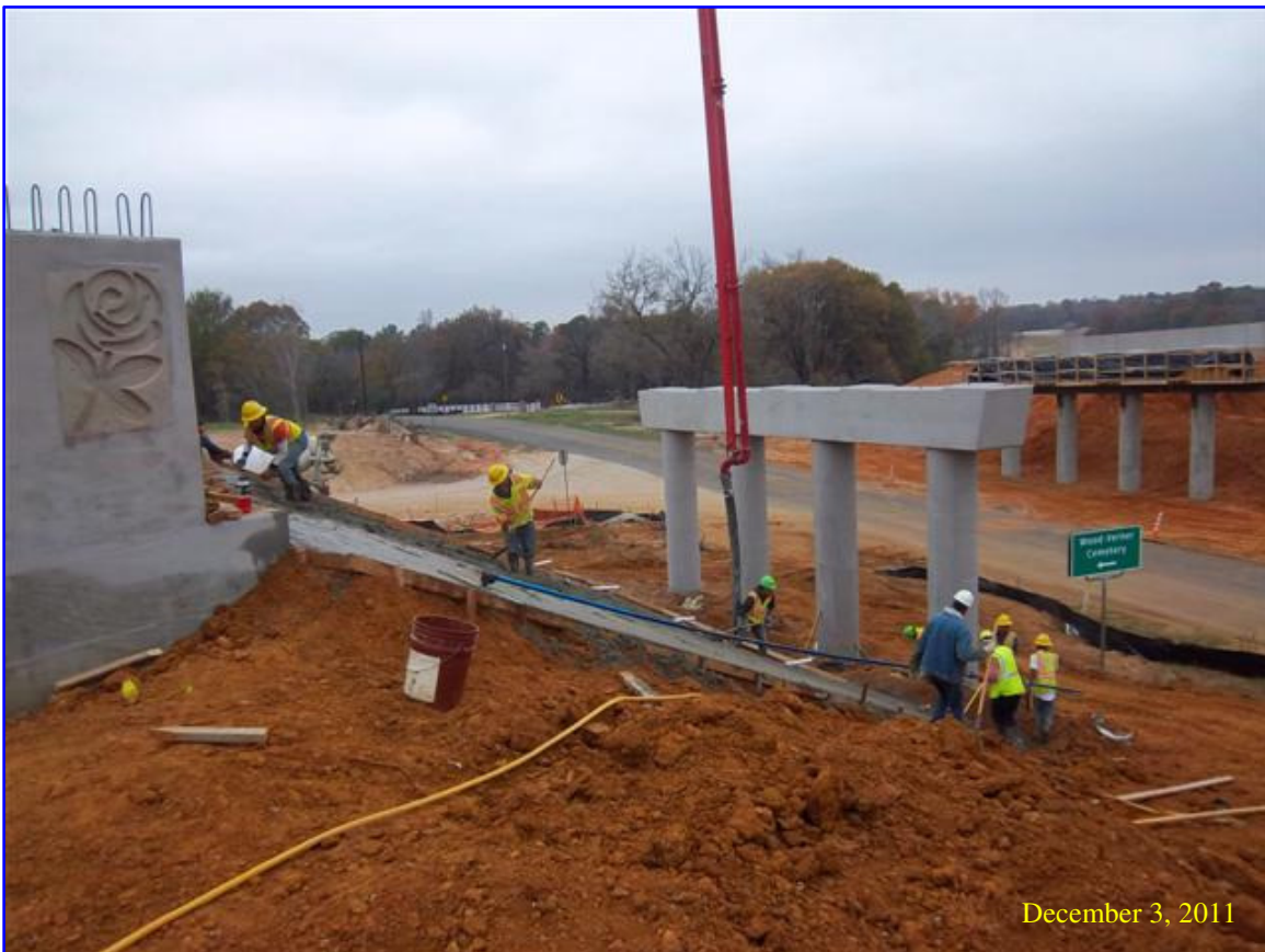
Construction of concrete riprap on east abutment of FM 724.
