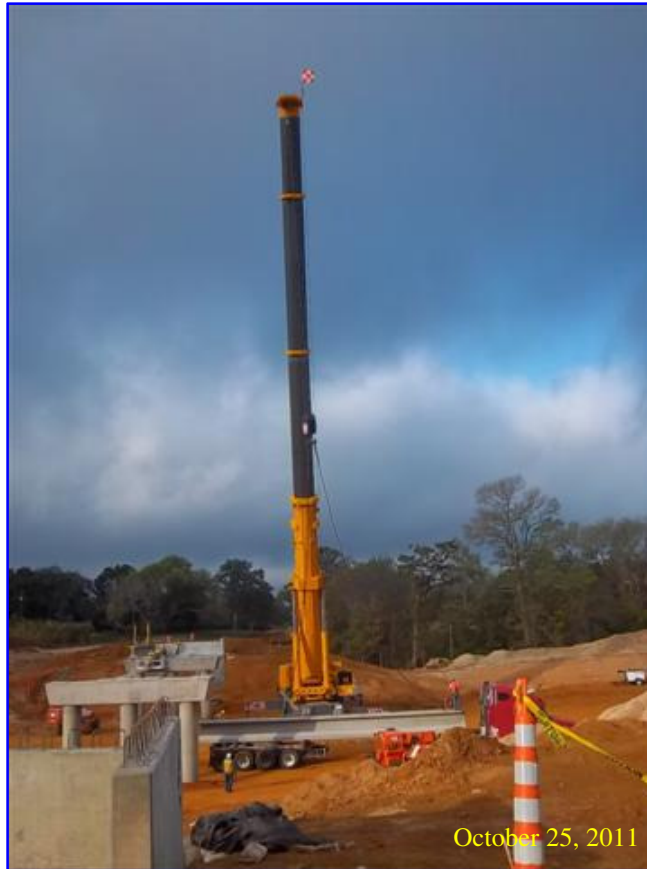
Pre-stressed Concrete Beam placement at CR 1145.
