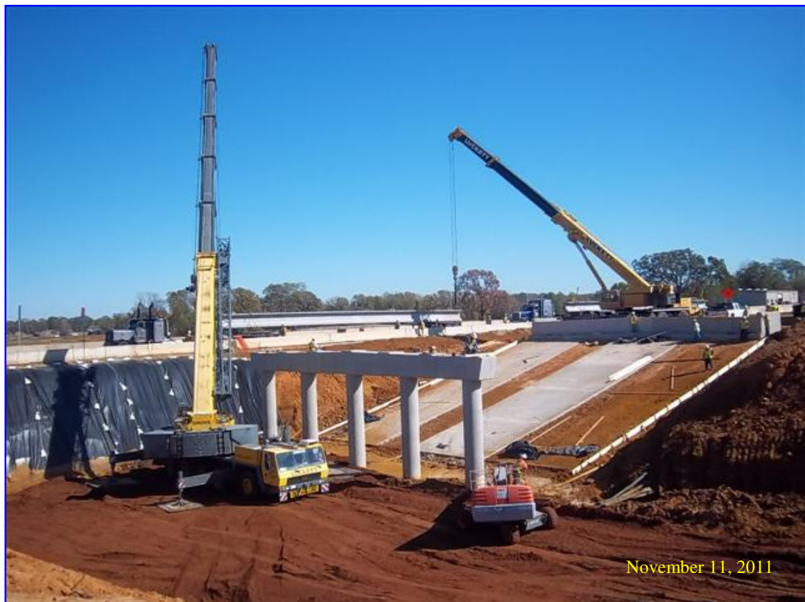
Installation of Pre-stressed Concrete Beams on SH 64.
