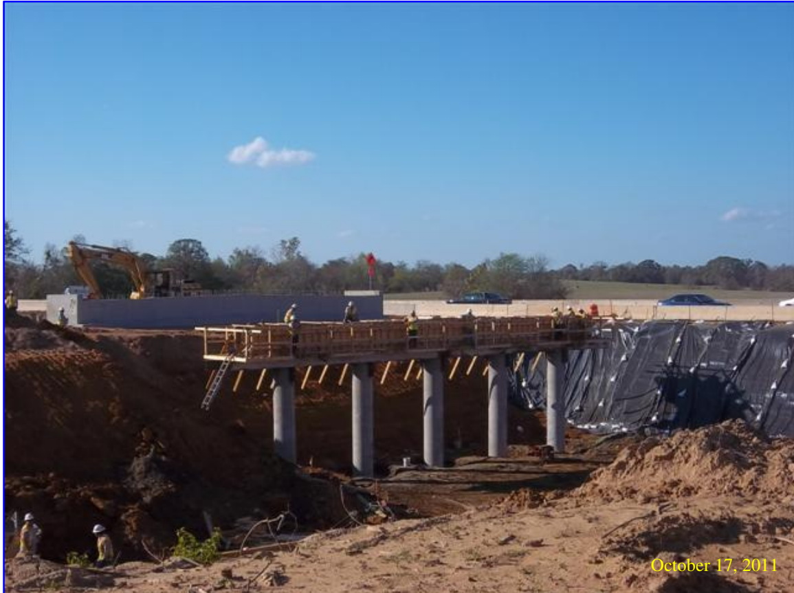
Construction of SH 64 bridge bent cap.
