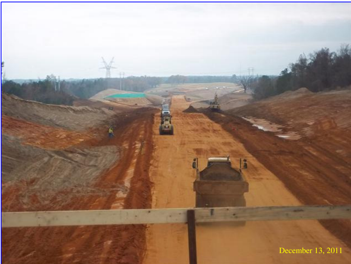
Finish grading operations looking south from CR 1145 Bridge.
