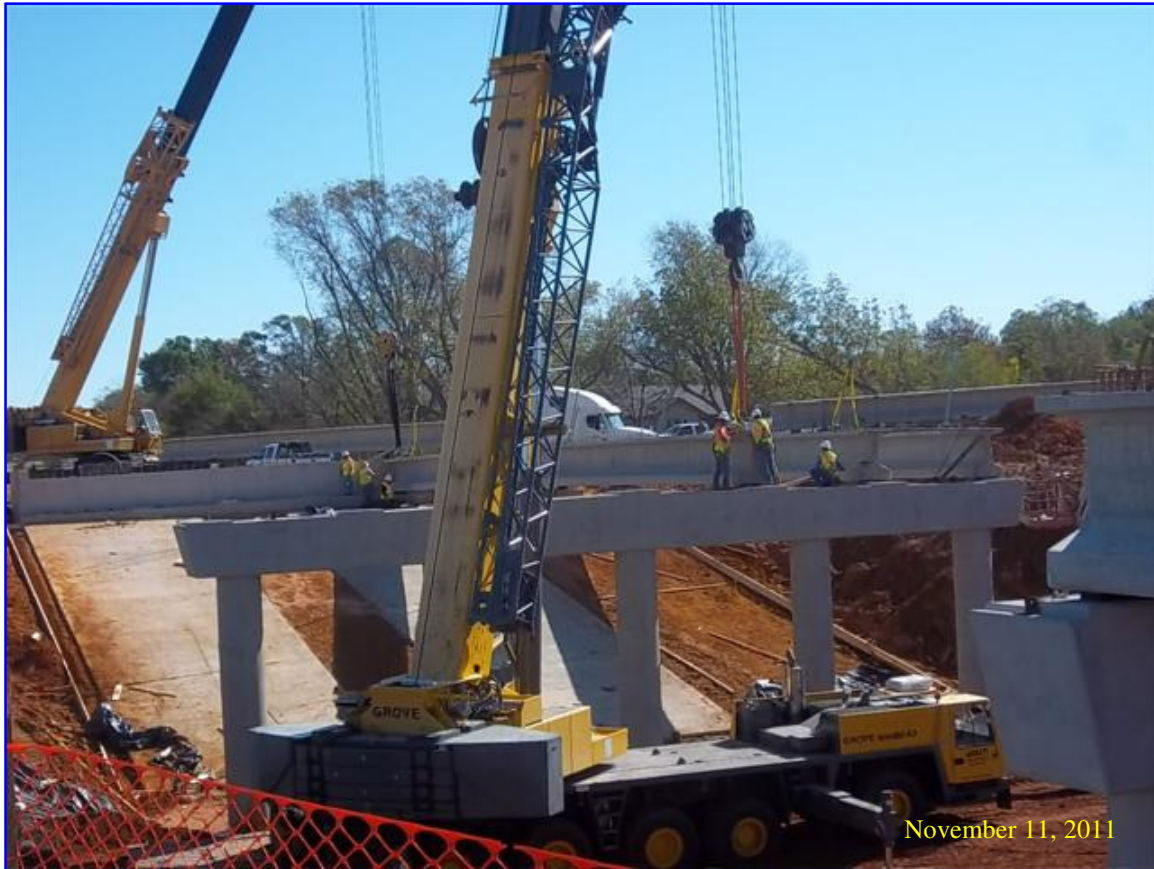
Placement of Pre-stressed Concrete Beams for SH 64 bridge.
