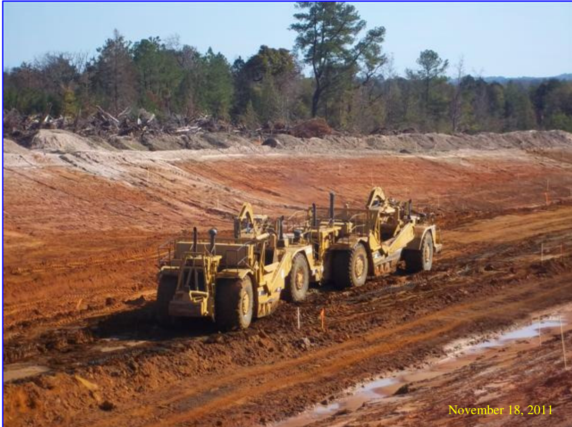
Scraper operations preparing rough cut finished subgrade.
