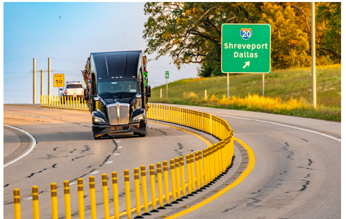
An average of 1300 delineators are replaced every year along the toll road.
