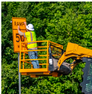
Installation & maintenance of signage.
