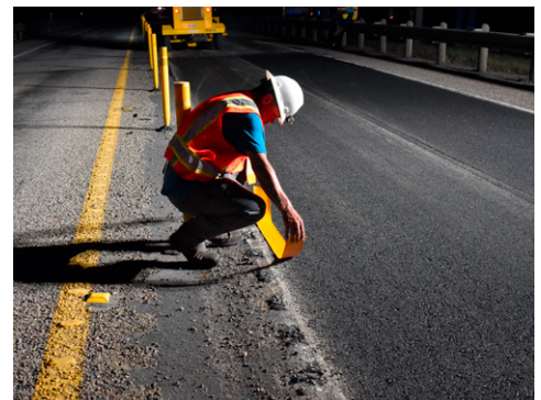
Applying striping after milling and overlay operations.
