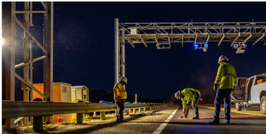
Replacing gantry sensor strips during nighttime road closure.
