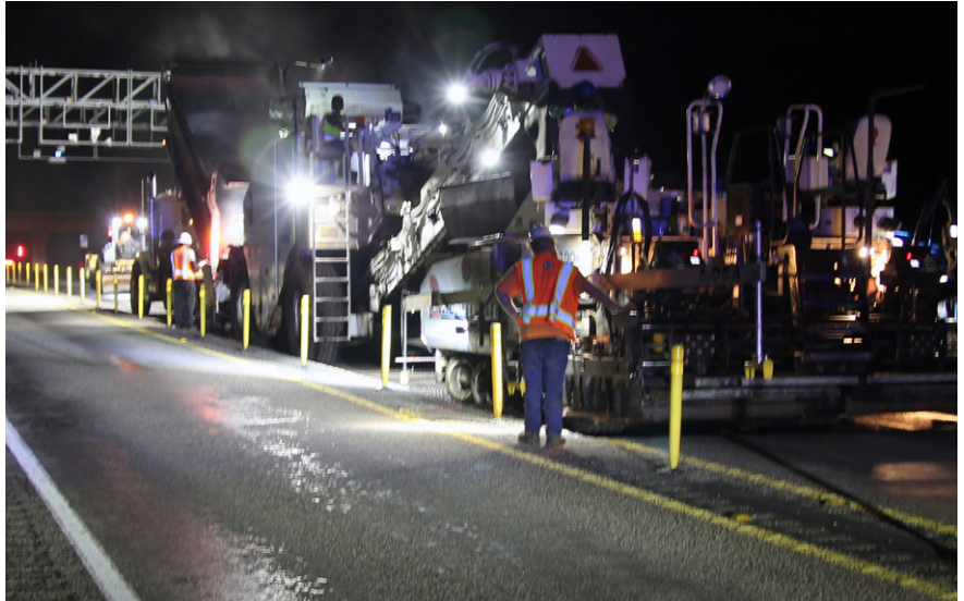
5-mile overlay using a Superpave asphaltic mixture.
