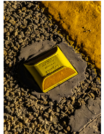
Raised pavement markers, (RPM's) are replaced every 2 years with additional replacement cycles every 6 months as needed.
