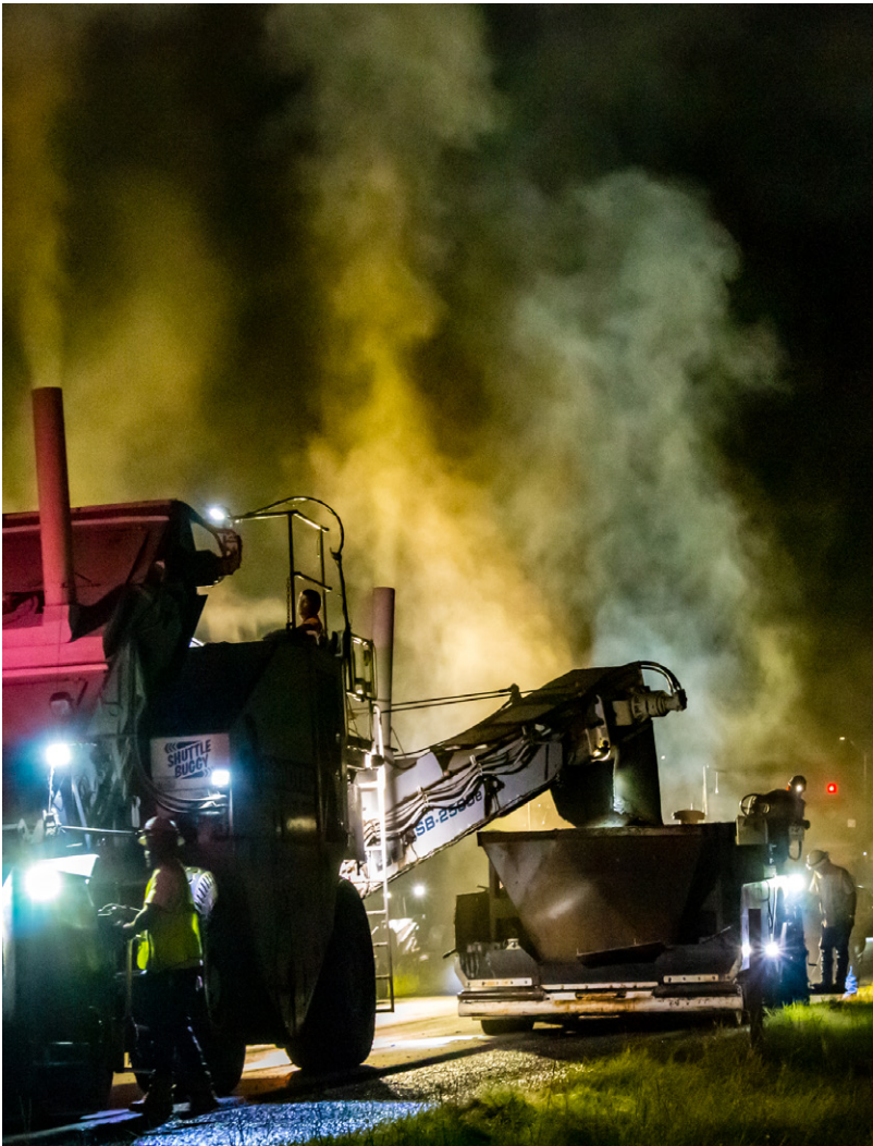
Hot mix resurface on Segment 1
