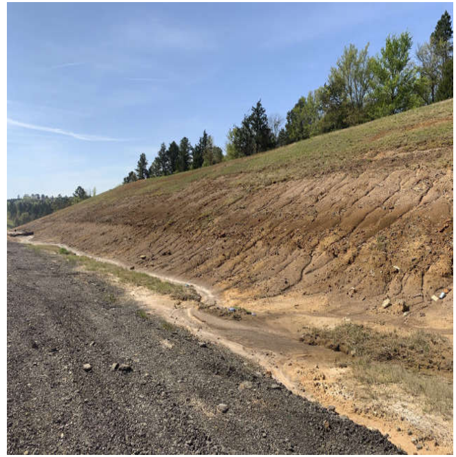
Figure 15: Slope Erosion
