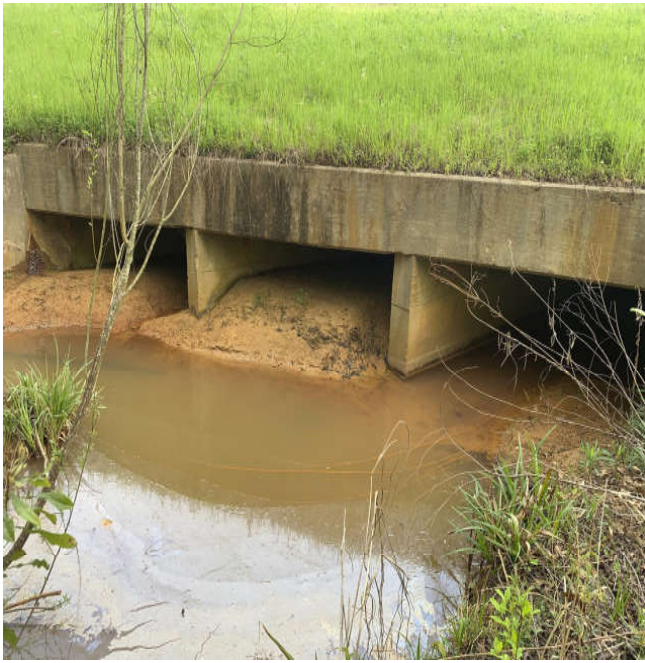
Figure 13: Box Culvert Silted Up
