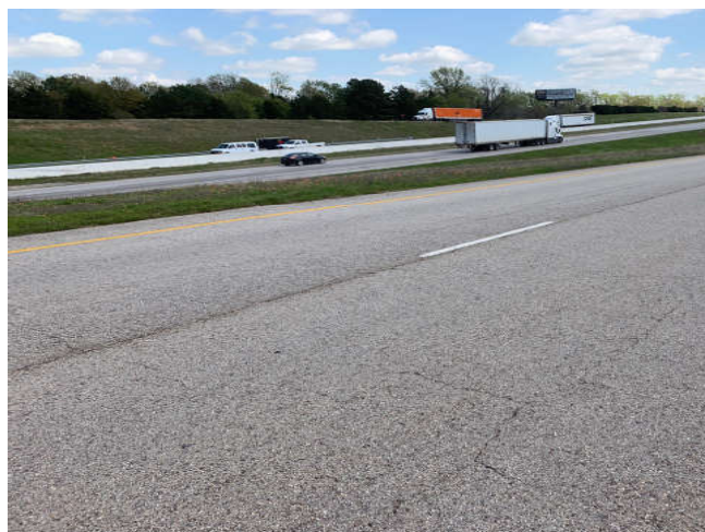
Figure 3: Pavement Cracking on Frontage Road
