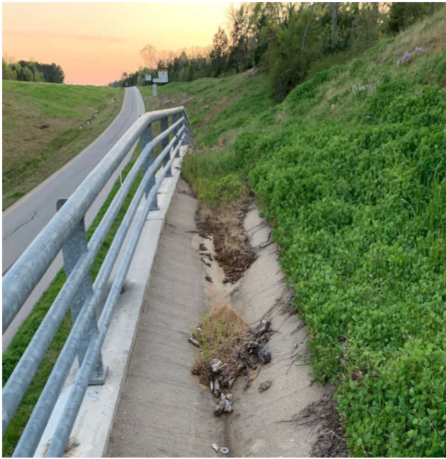
Figure 17: Debris in Retaining Wall Flume
