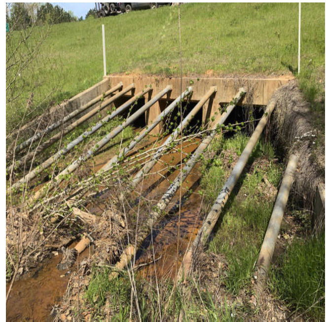
Figure 12: Structure Silted Up
