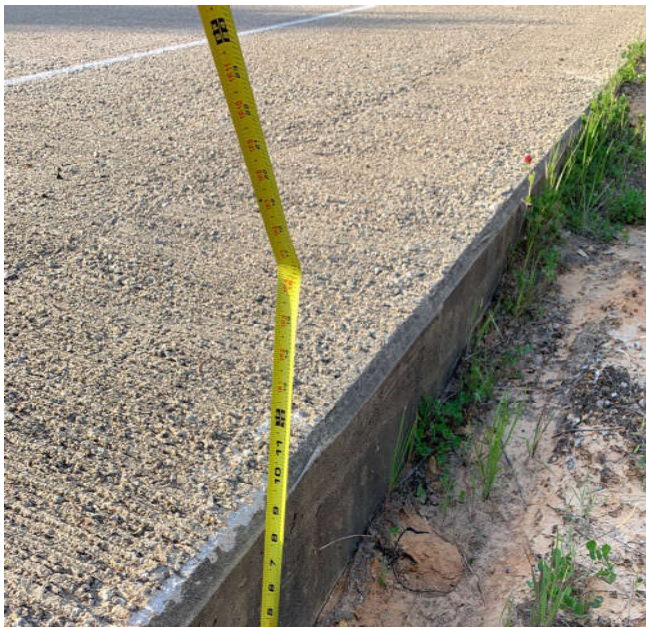
Figure 5: Pavement Drop-Off
