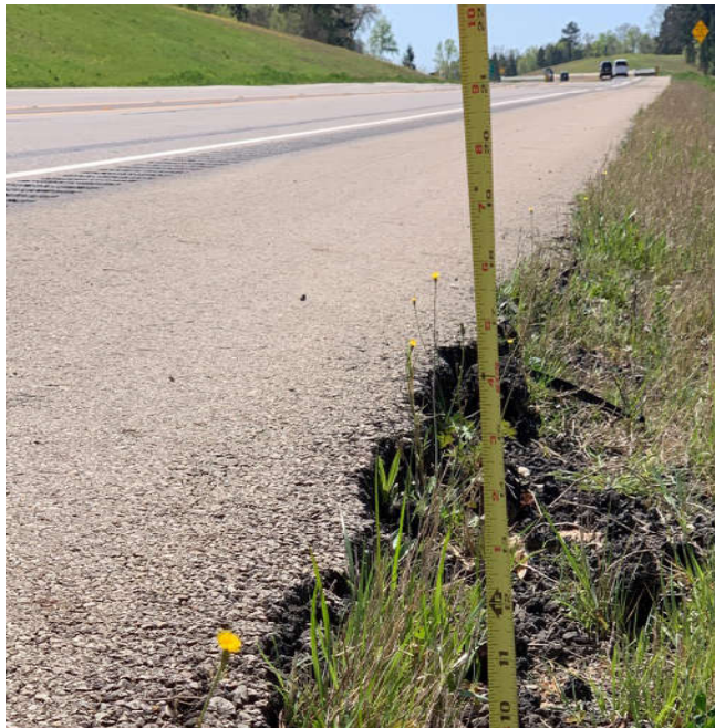
Figure 6: Pavement Drop-Off
