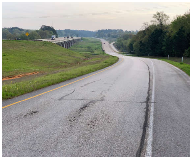
Figure 2: Pavement Cracking Frontage Road
