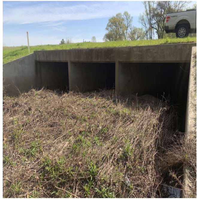
Figure 11: Box Culvert Partially Blocked
