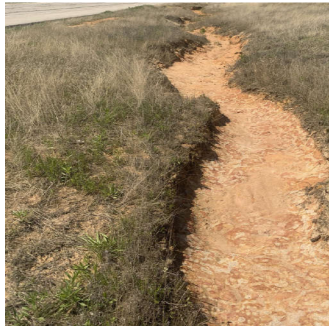
Figure 16: Ditch Erosion
