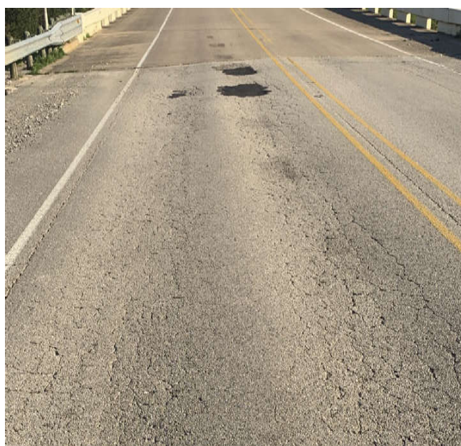
Figure 4: Pavement Cracking on Cross Street
