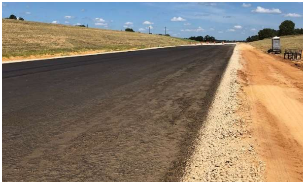
Placement of prime coat over the flexible base by FM 849
