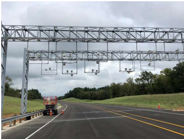
Cameras installed on mainlane toll gantry structure
