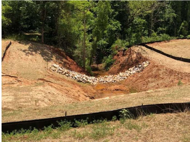
Installation of stone rip rap and silt fence at Culvert No. 7
