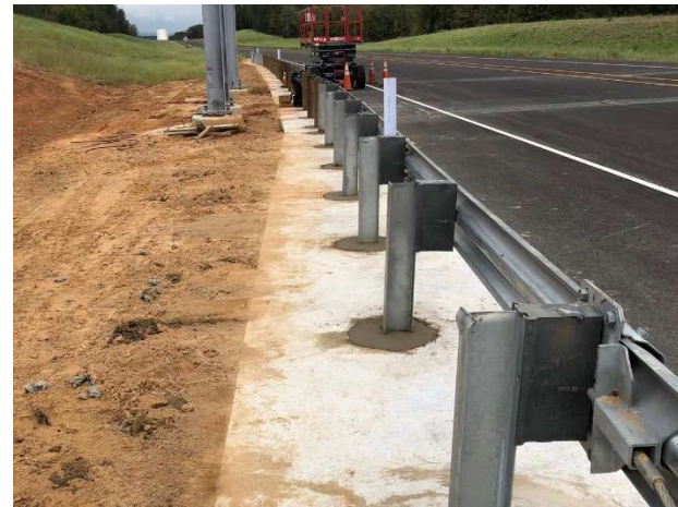
Flowable fill placed at guardrail supports at the main lane gantry
