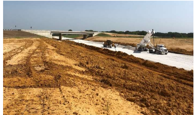
Placement of drainable pavement layer at FM 849
