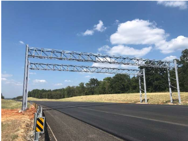
Columns and truss at mainlane gantry location
