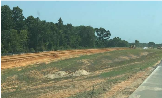
Cement treatment for northbound ramp
