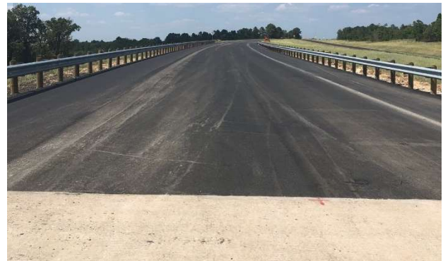
Progress on the laying of hot mix asphalt north of FM 16
