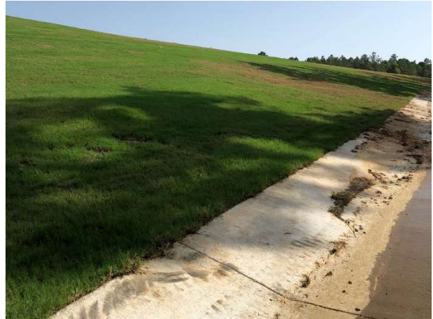
Installation of sod on the backslope north of CR 431
