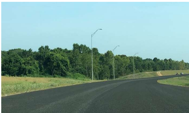
Completed One Course Surface Treatment from FM 849 to IH-20.
