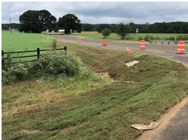
Installation of sod in drainage ditch near the southbound ramp at SH 110
