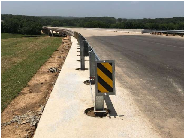
Guardrail and mow strip installed on CR 431 bridge
