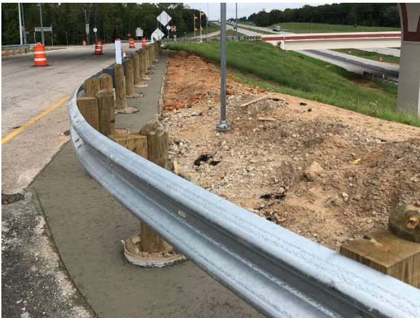
Guardrail installation and mow strip construction at the IH 20 frontage road
