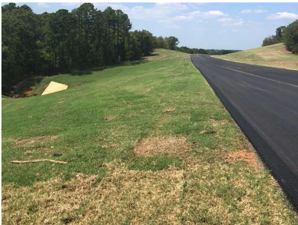
Installation of sod at Culvert No. 7 outfall
