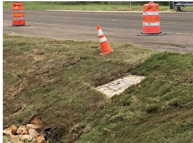
Ground box installation near southbound ramp at SH 110
