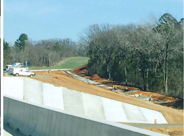
Completed concrete rip rap construction at CR 431 bridge
