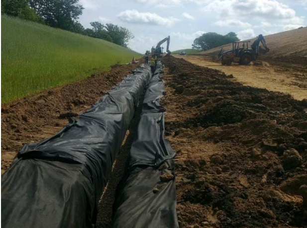
Construction of underdrains between CR 4118 and CR 431
