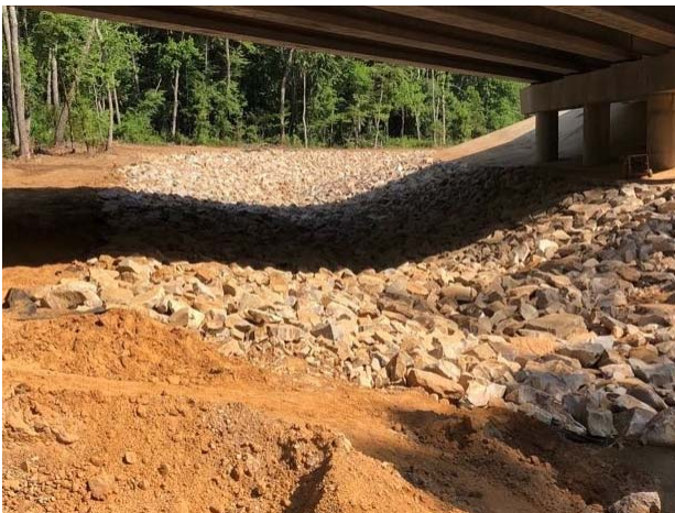
Rock rip rap installation at Davis Branch Tributary Bridge
