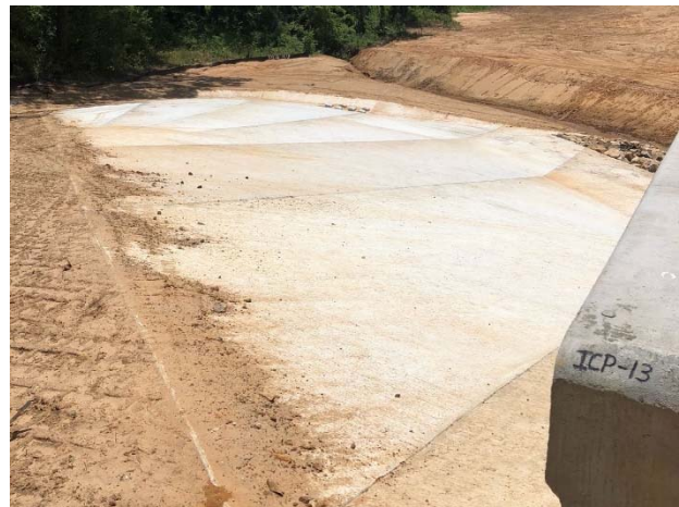
Concrete rip rap construction at Davis Branch Tributary outfall
