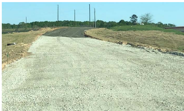
Flexible base installation for the SH 110 southbound ramp
