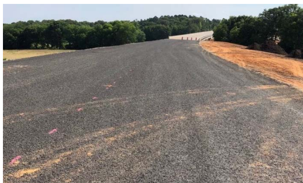
One Course Surface Treatment placed from US 69 to Stevenson Branch bridge
