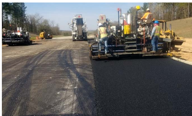
Asphalt placement North of FM 16
