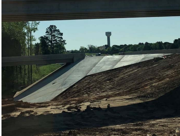
Completed concrete rip rap construction at Long Brake Tributary bridge
