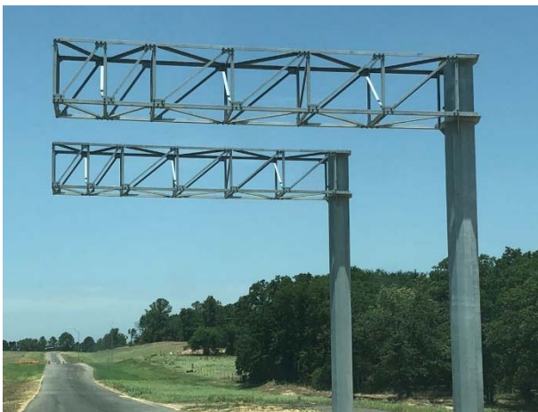
Columns and cantilever trusses on northbound ramp at FM 16
