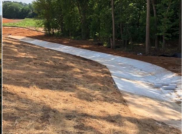
Concrete rip rap construction for ditches south of Stevenson Branch
