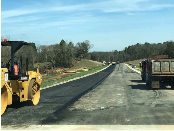
Asphalt paving south of Davis Branch Bridge
