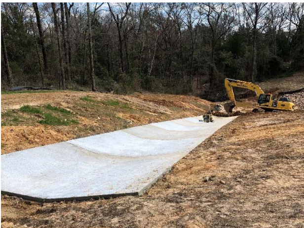
Concrete rip rap for drainage near Culvert No. 16, south of FM 849
