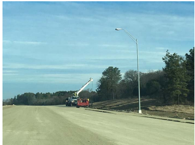
Installation of luminaire poles for the exit ramp south of FM 16
