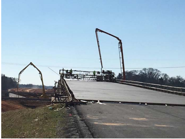
IH 20 main lane overpass bridge deck construction
