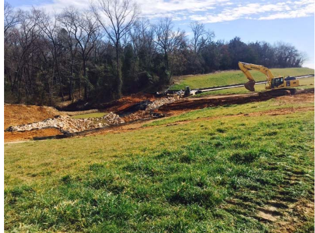
Rock rip rap and silt fence at Culvert No. 16, south of FM 849
