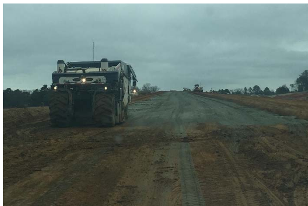
Cement treatment of the pavement subgrade south of FM 16
