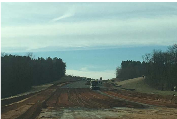
Cement treatment of the pavement subgrade north of FM 16
