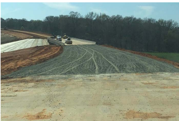
Flexible base installation between the CR 431 and Stevenson Branch bridges
