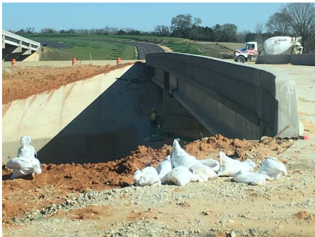
Superstructure patching and sealing at the northbound ramp bridge at IH 20
