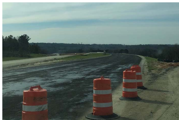
Primed flexible base for the main lanes north of FM 16 at the ramp tie-ins
