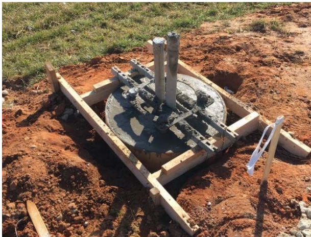
Construction of drilled shafts for main lane gantry north of FM 16
