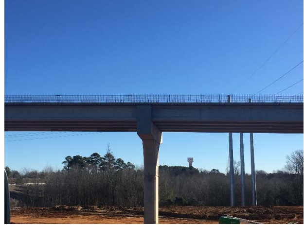
Construction of the concrete bridge rail of the IH 20 main lane overpass
