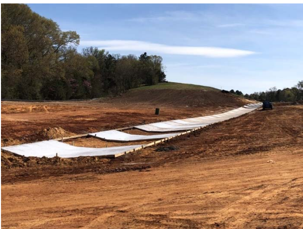
Concrete rip rap for drainage south of Stevenson Branch
