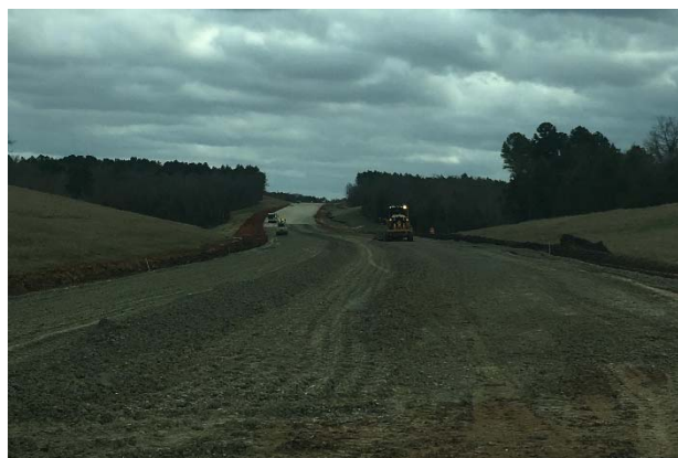
Flexible base installation north of FM 16
