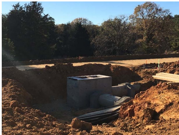
Drop inlet construction just south of FM 16
