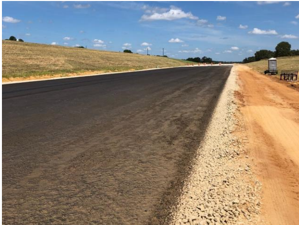
Placement of prime coat over the flexible base by FM 849
