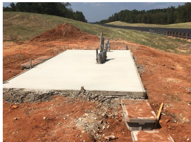
Completed equipment pad for the Gantry Structure north of FM 16
