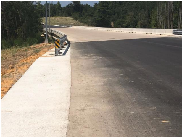
Completed mow strip at Davis Branch bridge
