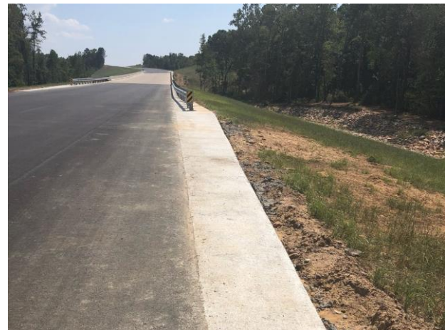
Completed mow strip at Davis Branch Tributary bridge
