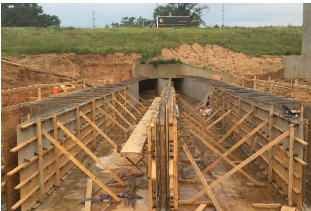
Culvert No. 19 wall forms south of IH 20
