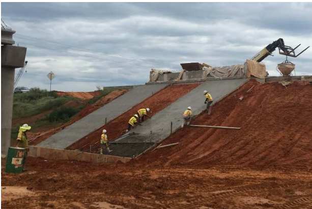
Construction of riprap at Long Brake Tributary bridge abutment
