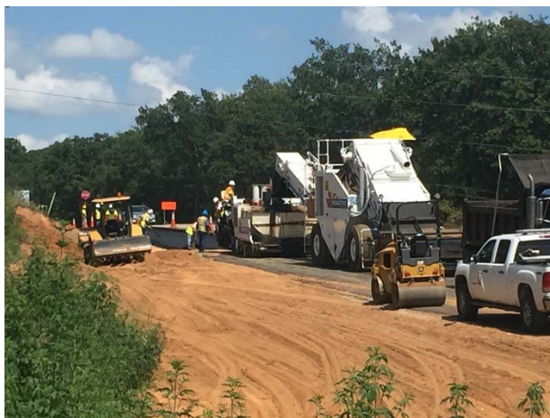
Tie in pavement construction in preparation for FM 16 traffic switch
