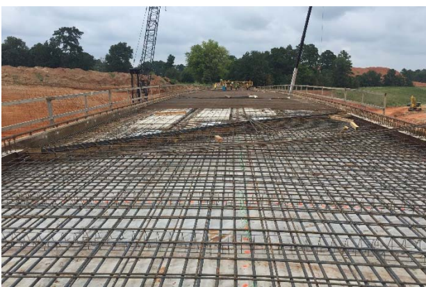
Steel reinforcing bars for CR 4118 bridge deck
