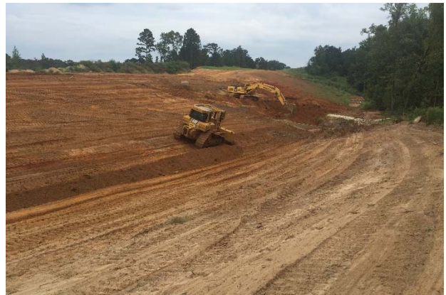
Shaping of side slopes at Davis Branch
