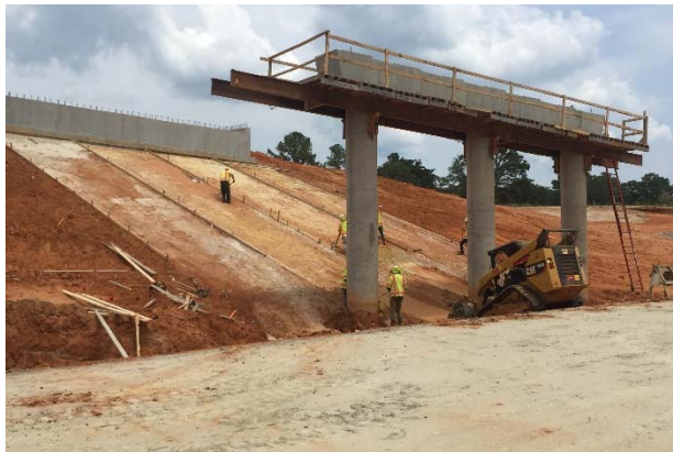
Cap construction and riprap forms on the north end of FM 16 bridge
