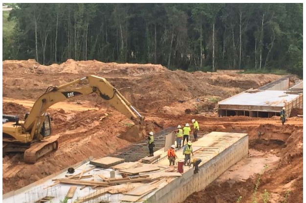
Construction of deck for Culvert No. 19 south of IH 20
