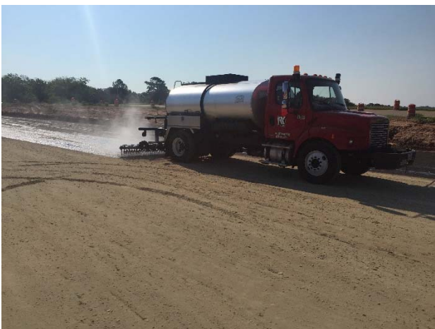
Placement of seal coat on FM 16 pavement
