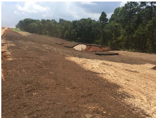
Seeding and silt fence south of Stevenson Branch near Culvert No. 7
