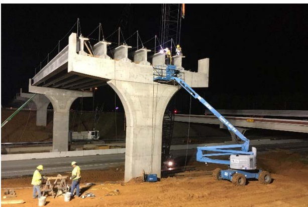
Nighttime placement of main lane bridge beams over IH 20
