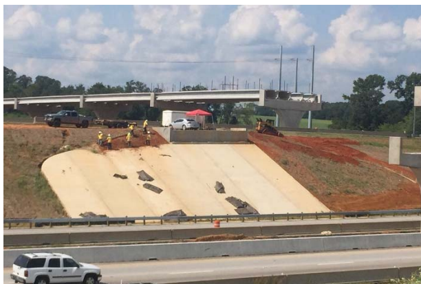
Placement of concrete riprap IH 20 northbound ramp bridge abutment
