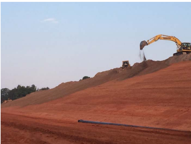
Installation of topsoil on side slopes just south of CR 4118
