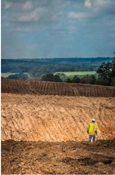
Clearing and grubbing north of IH 20
