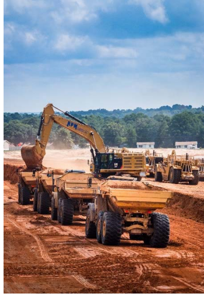
Excavation activities near US 69
