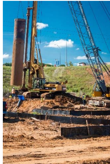
Drilled shaft work at the future IH 20 overpass
