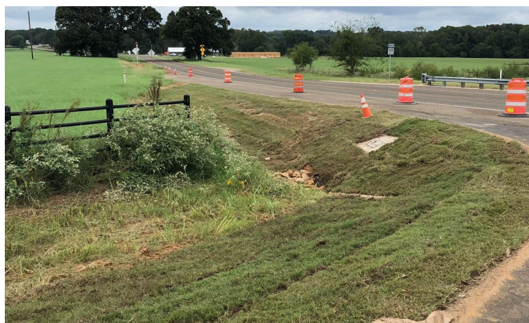
Installation of sod at ditch near southbound ramp at SH 110
