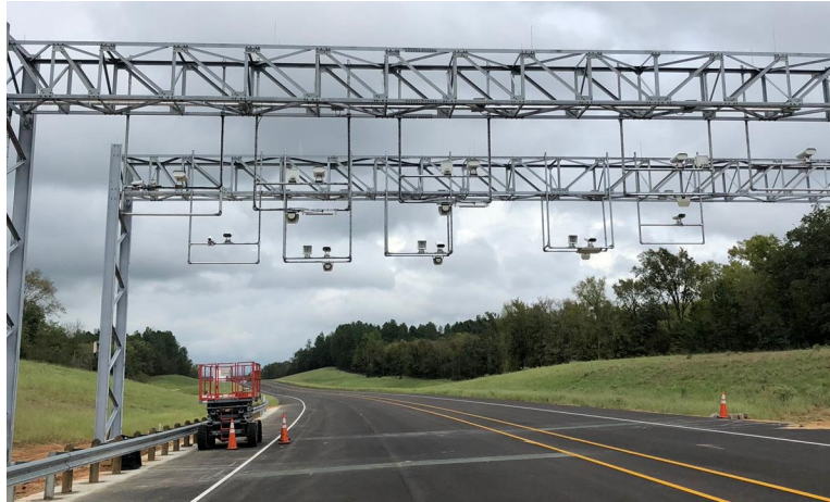
Cameras installed at Mainlane Toll Gantry Station
