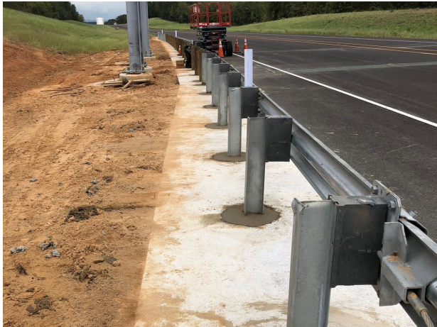
Guardrail installation at mainlane north of FM 16
