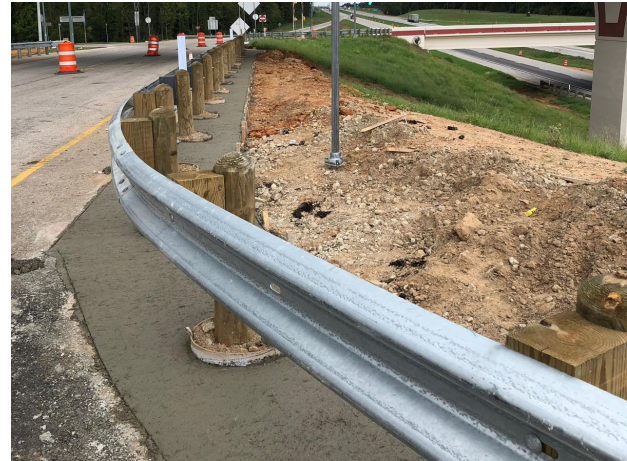
Guardrail installed at the northbound ramp bridge on IH 20
