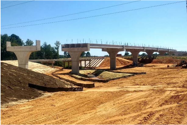
IH 20 main lane overpass beams and deck panels
