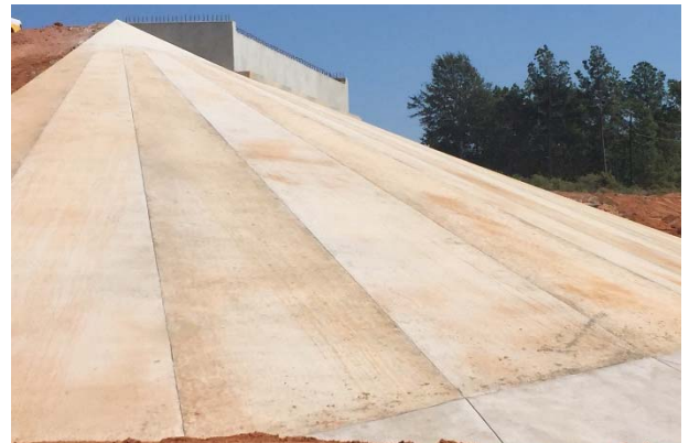
Concrete rip rap at FM 16 bridge abutment
