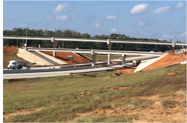
Beams installed over IH 20 for the main lane and northbound ramp bridges
