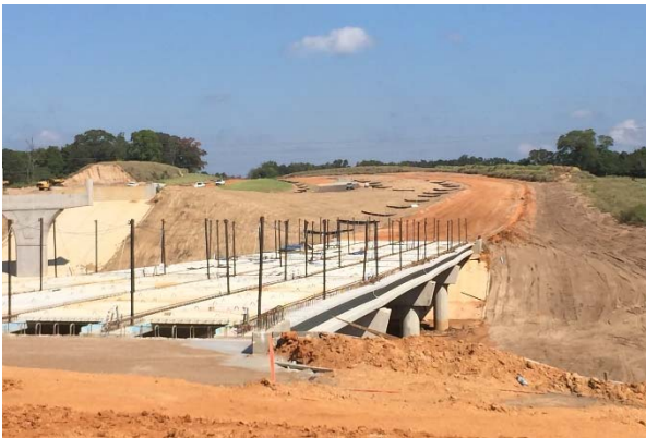
Deck pannels at Long Brake Tributary Bidge
