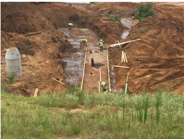
Footing construction for Culvert No. 18 north of IH 20
