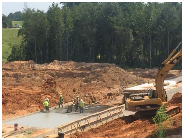
Construction of deck for Culvert No. 19 south of IH 20
