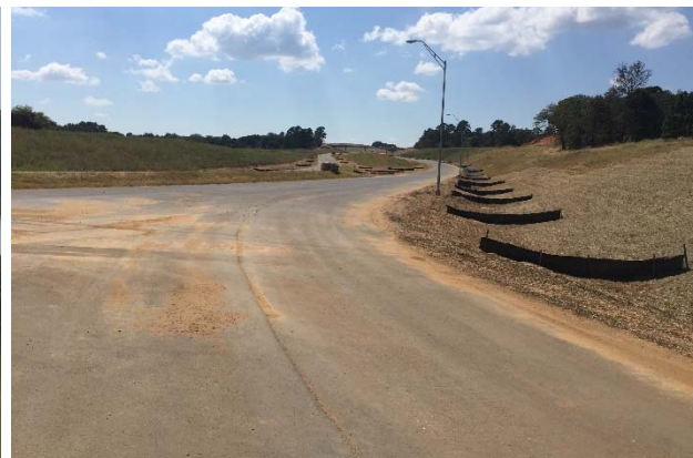
Silt fence south of US 69 at the Toll 49 entrance ramp
