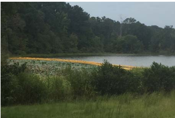
Floating turbidity barrier at Davis Branch
