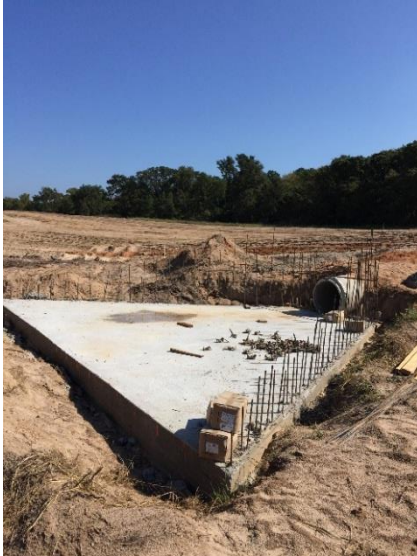
Culvert #11 footing construction (north of FM 16)
