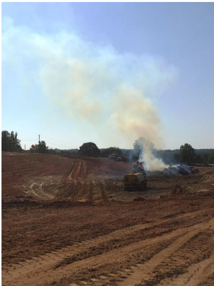
Clearing and grubbing (controlled burn north of FM 16)
