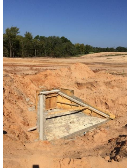
Culvert #11 wingwall installation (north of FM 16)
