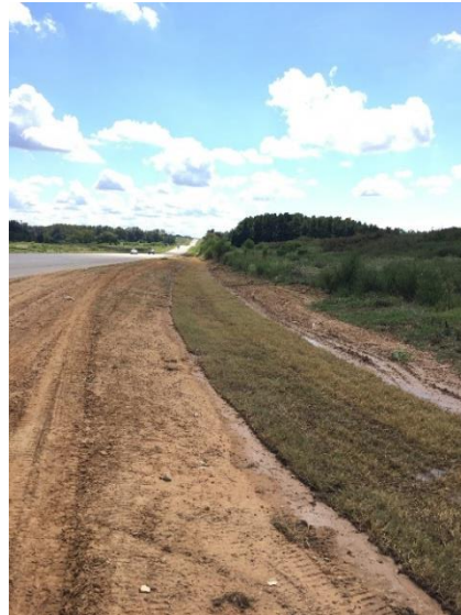
Sod over underdrain installation south of IH 20 (southbound side facing south)
