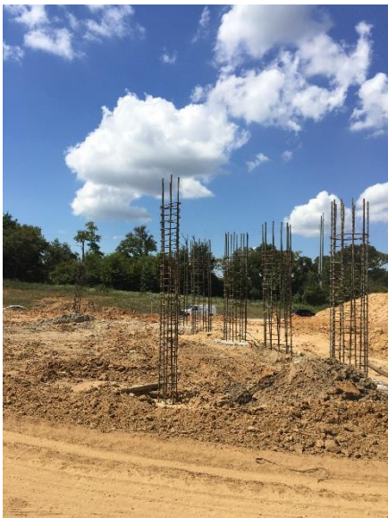
Drilled shaft work at IH 20 overpass (Abutment No. 17)
