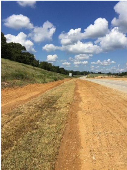
Sod over underdrain installation south of IH 20 (southbound side facing north)
