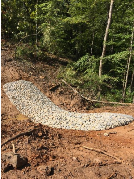
Rock filter dam at proposed culvert No. 8 location south of Stevenson Branch
