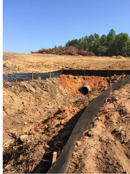
Silt fence at culvert No. 9 between Stevenson Branch and FM 16
