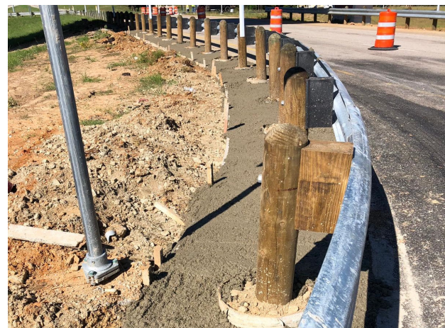
Placement of concrete mow strips at northbound ramp at I-20
