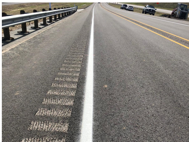
Pavement markings and rumble strips placed throughout the project
