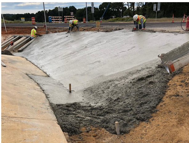
Concrete rip rap placement at FM-16
