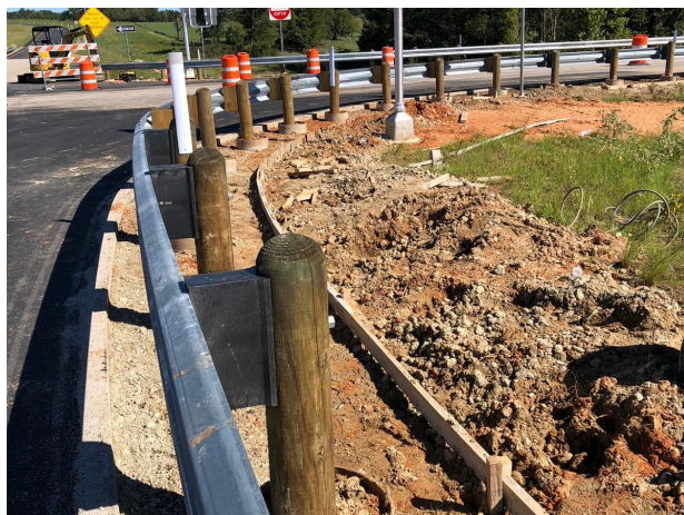
Concrete mow strip forms at northbound ramp at I-20
