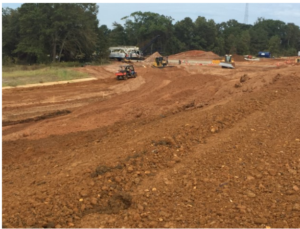
Side slope grading south of FM 16
