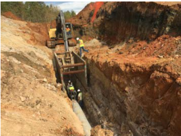
Installation of reinforced concrete pipe near CR 431
