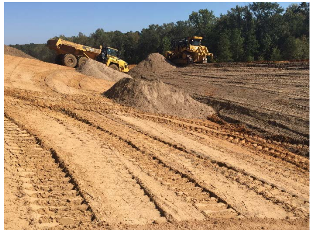
Placement of topsoil and seeding on side slope south of CR 4118
