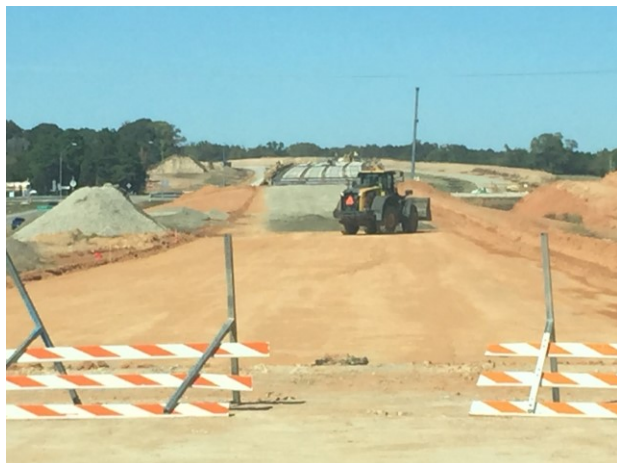
Flex base installation at IH 20 main lane overpass abutment
