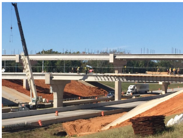
Installing overhangs for the IH 20 northbound ramp bridge
