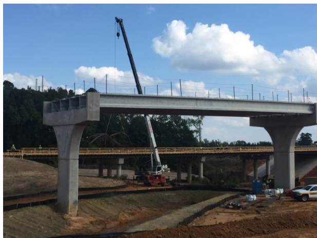
Tying steel prior to the concrete deck placement at Long Break bridge
