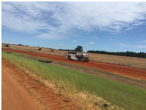
Cement treating subgrade north of the IH 20 main lane overpass
