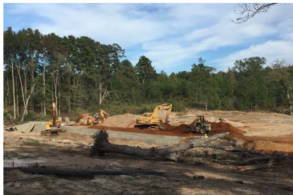
Backfilling at Culvert No. 12
