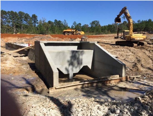
Culvert #12 wingwall construction (south of FM 16)
