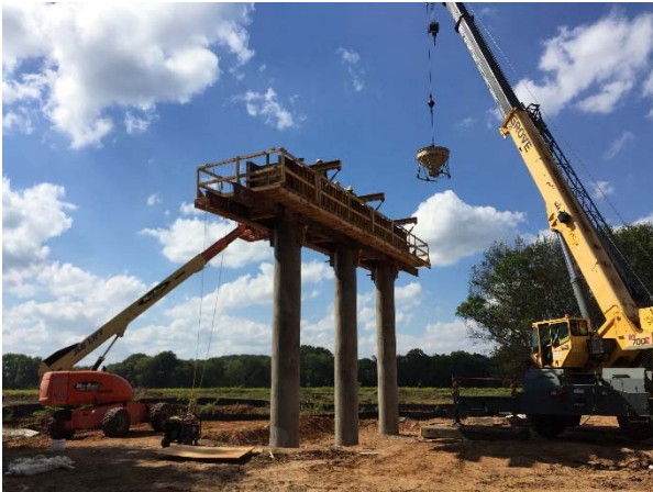
Cap placement at CR 431 bridge
