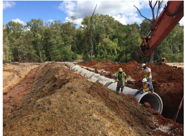
Culvert #15 reinforced concrete pipe installation (north of FM 849)
