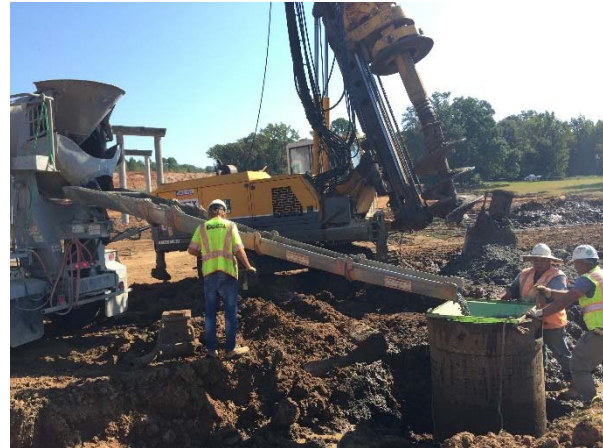
Drill shaft work at CR 431
