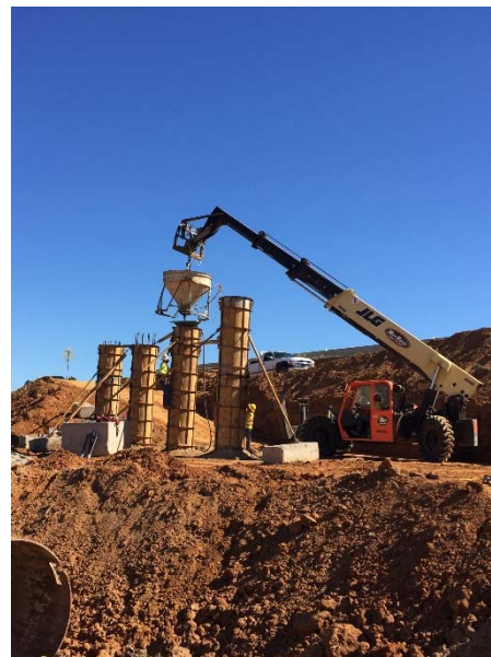
Column construction at Long Brake Tributary north of IH 20
