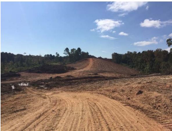
Clearing and grubbing between IH 20 and FM 849
