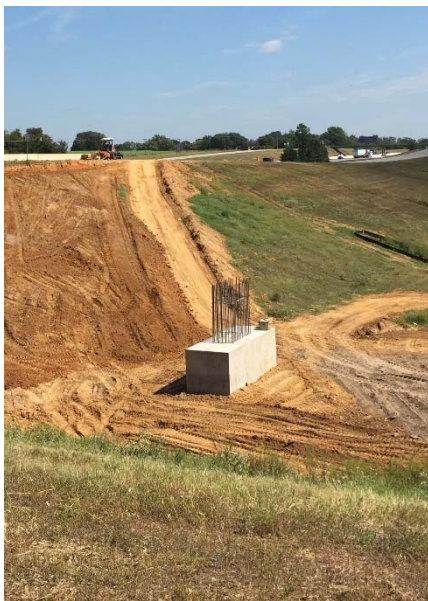
Footing at future main lane overpass at IH 20
