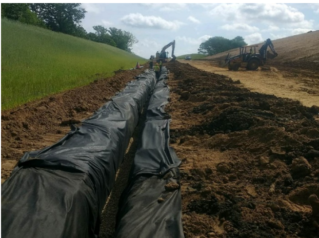
Construction of underdrains between CR 4118 and CR 431
