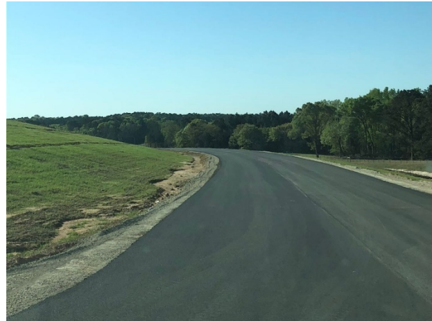
Completed 4 inch base layer of asphalt south of FM 16
