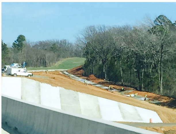
Completed concrete rip rap construction at CR 431 bridge
