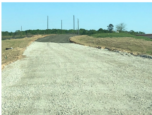
Flexible base installation for the SH 110 southbound ramp
