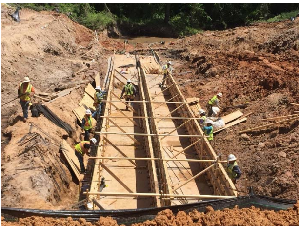
Forms in preparation of Culvert No. 16 concrete
