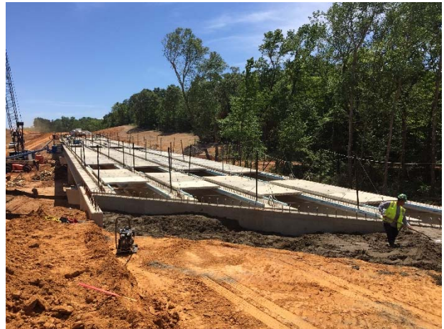
Backfilling/embankment at the Stevenson Branch abutment
