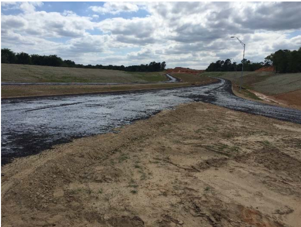
Fresh prime coat prior to asphalt paving just south of US 69
