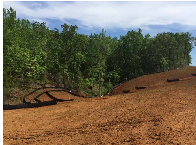
Silt fence south of Stevenson Branch near Culvert No. 8
