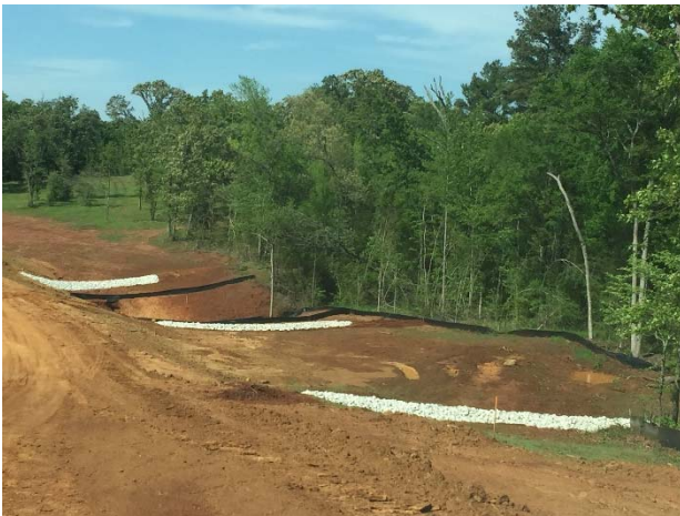
Rock filter dams south of Stevenson Branch near Culvert No. 7
