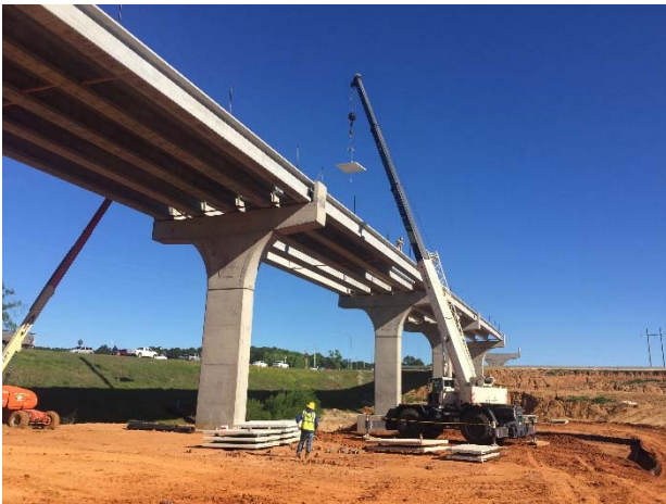
Deck panels at the IH 20 main lane overpass bridge
