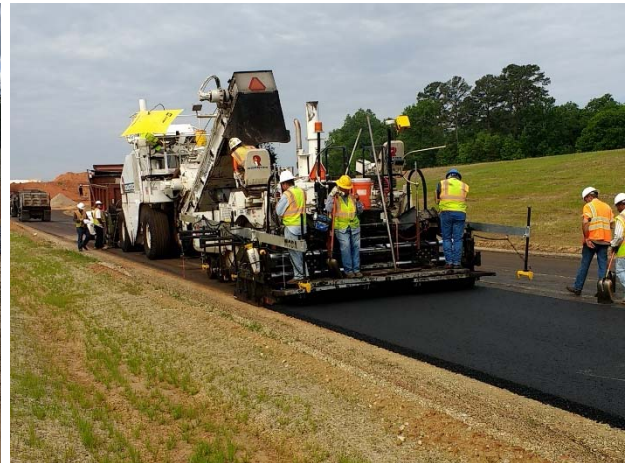
Hot mix asphalt paving from south of US 69 to just north of CR 4118
