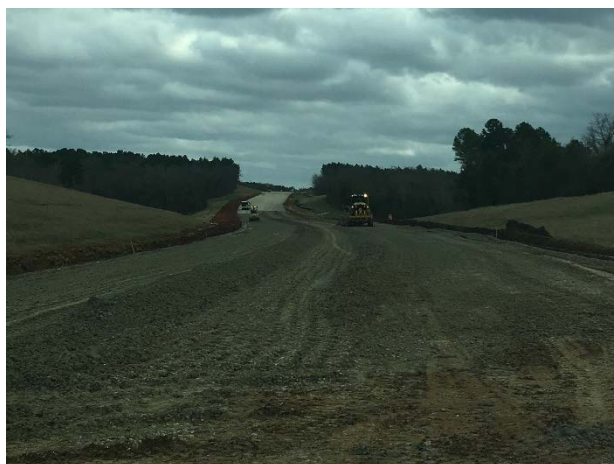
Flexible base installation north of FM 16
