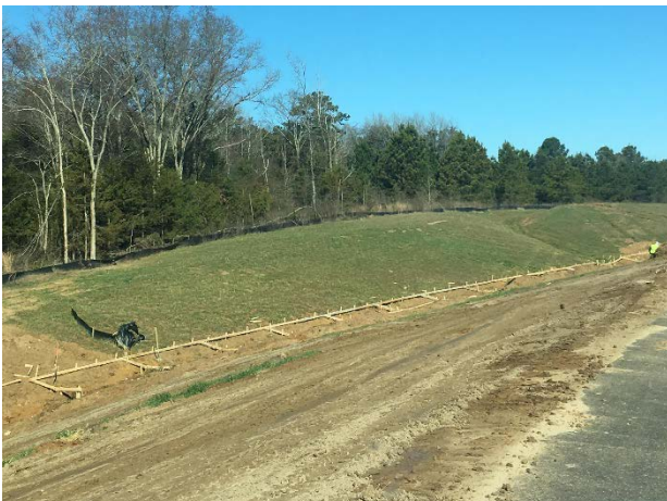
Forms for concrete rip rap near Culvert No.16, south of FM 849
