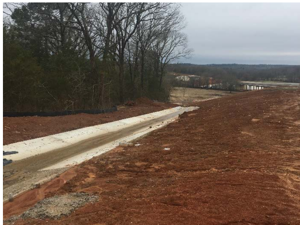
Concrete rip rap near Culvert No. 16, south of FM 849
