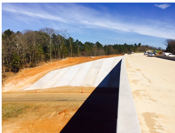
Concrete rip rap at the CR 431 bridge abutment
