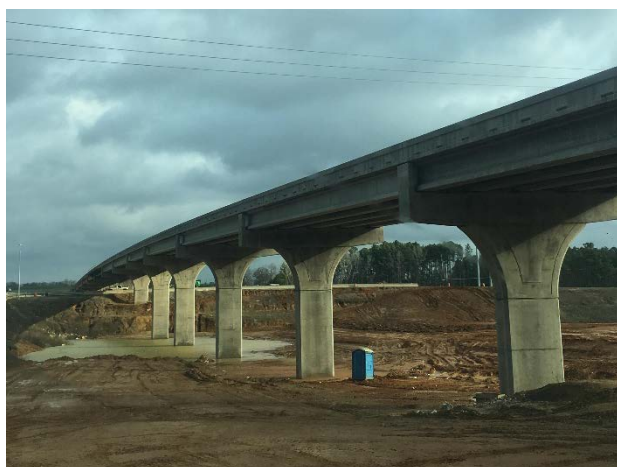
Completed bridge rail construction on IH 20 main lane overpass
