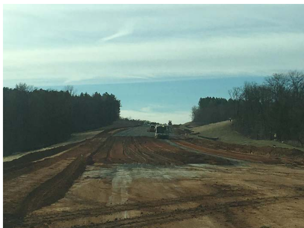
Cement subgrade treatment north of FM 16
