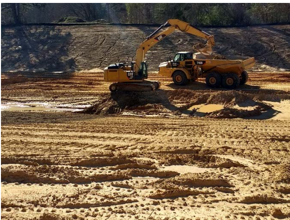
Remove/replace unstable subgrade material (Change Order No. 4)
