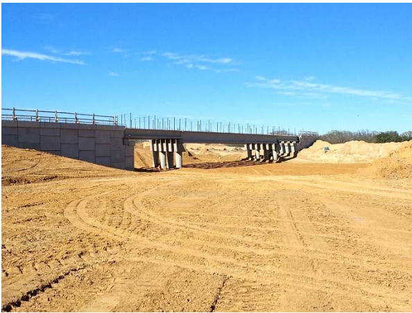
Completed columns, girders, and abutment MSE walls at FM 849 Bridge
