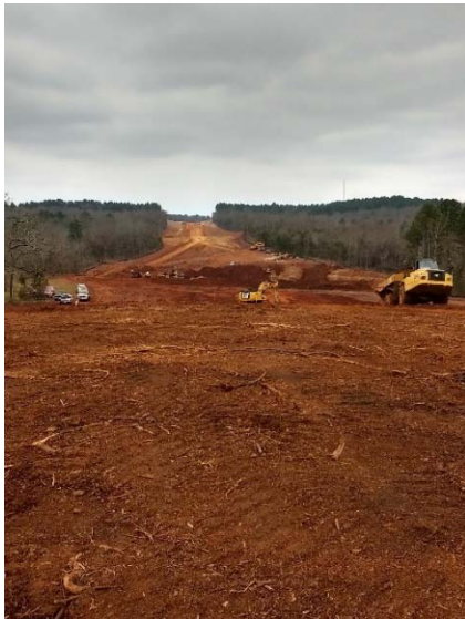
Clearing/grubbing, excavation, and embankment in expanded access area near archeological site
