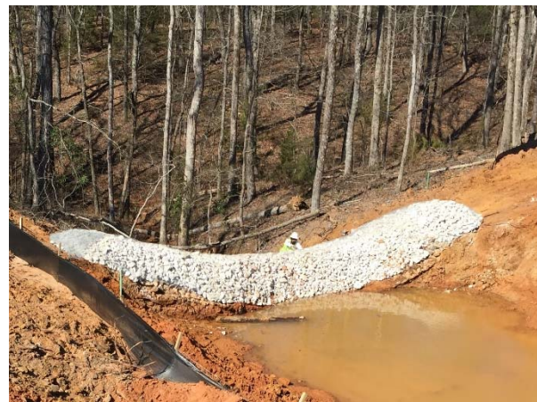
Rock filter dam at major cross Culvert No. 10 (Change Order No. 4)
