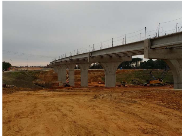
Girder placement for IH 20 main lane overpass, southern side of IH 20
