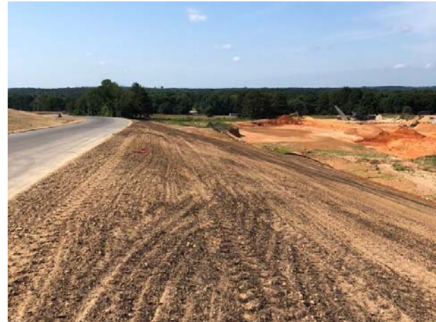
Top soil, seed compost, hay mulch installation north of FM 16
