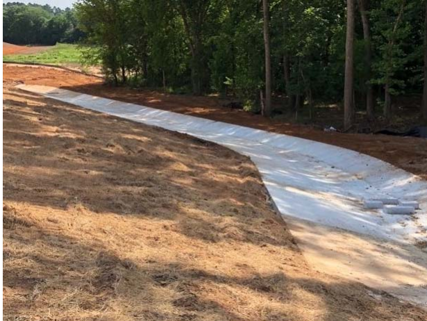
Concrete rip rap construction south of Stevenson Branch
