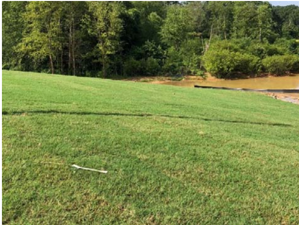
Sod installation on side slopes north of Davis Branch
