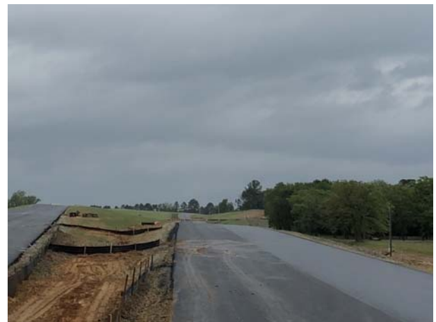
Paving Northbound ramp at FM 16
