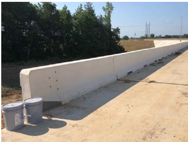
Concrete bridge rail painting at Long Break Tributary Bridge
