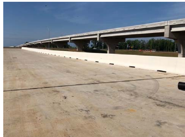
Concrete bridge rail painting at Northbound Ramp Bridge at IH 20
