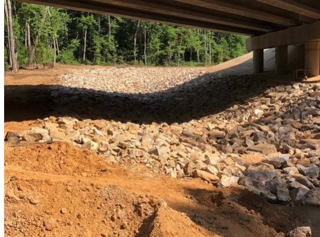
Rock rip rap construction at Davis Branch Tributary Bridge
