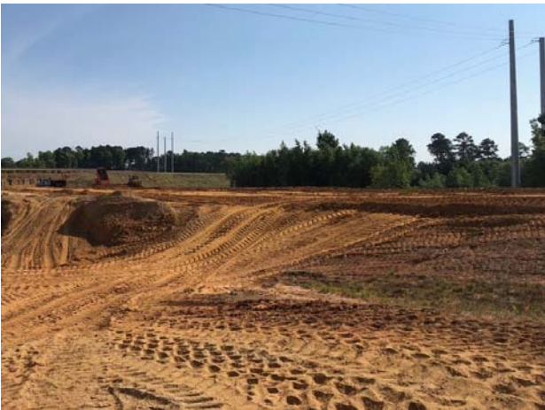
Embankment for the northbound ramp South of IH 20
