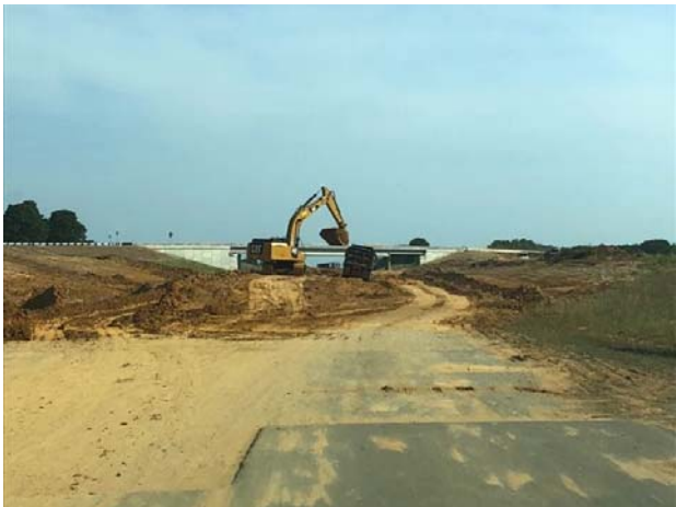
Excavation for the Toll 49 main lanes at FM 849
