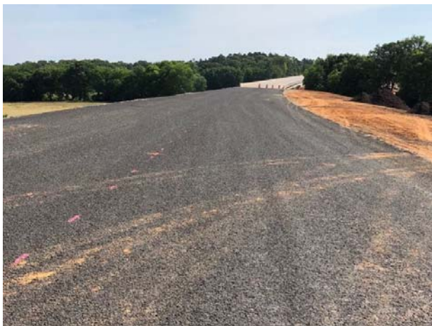
One Course Surface Treatment placed from US 69 to Stevenson Branch bridge
