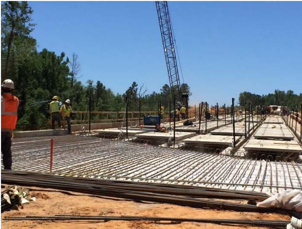
Davis Branch Tributary bridge deck panel installation
