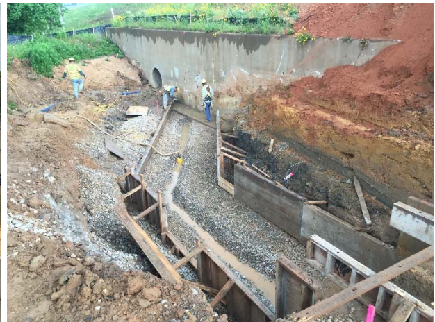
Footing forms for Retaining Wall No. 4 just south of IH 20
