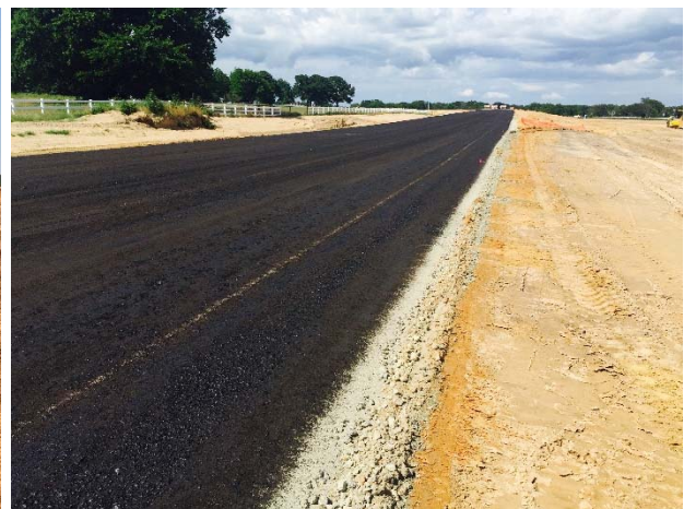
Prime coat placement on eastern portion of FM 849 future pavement
