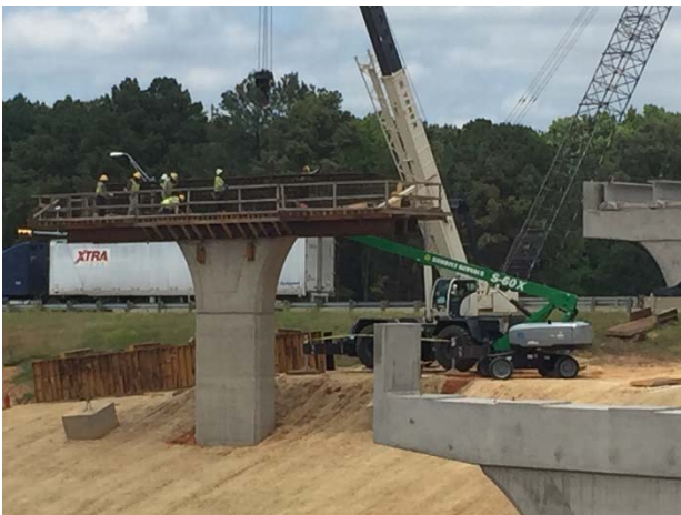
Cap construction at IH 20 main lane overpass
