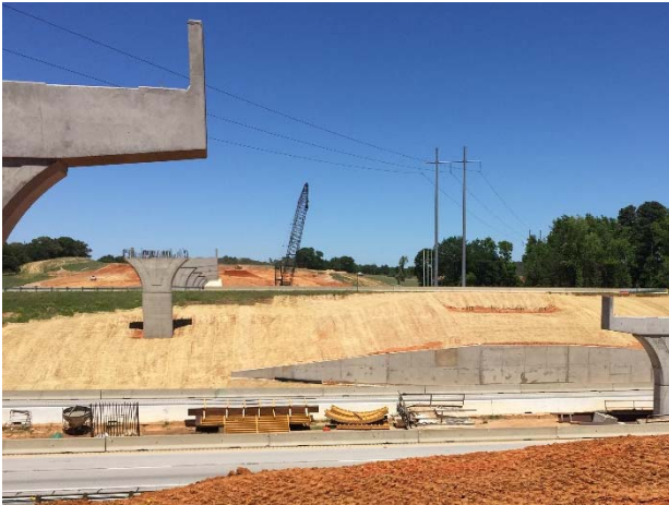
Erosion control blankets along IH 20 northern side slopes
