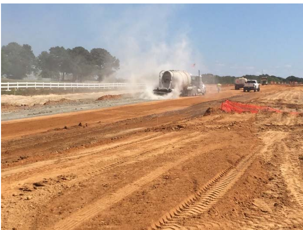
Cement treatment of subgrade on eastern portion of FM 849 future pavement
