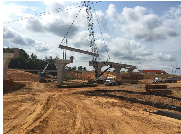
IH 20 main lane overpass beam placement (north of IH 20)
