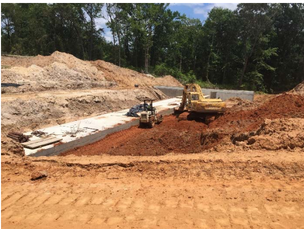
Backfilling at complete portions of Culvert No. 16 south of CR 849
