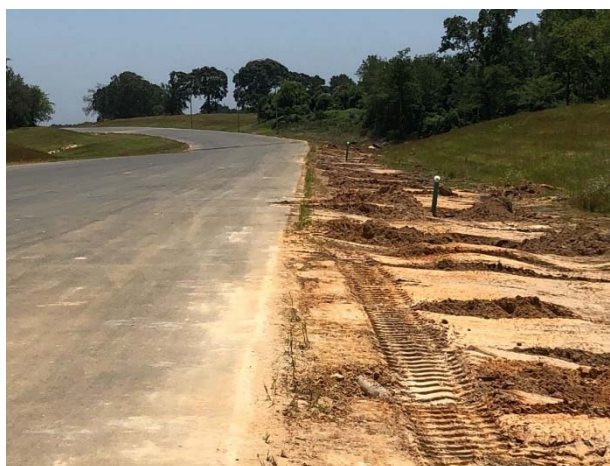
Completed construction of underdrain along the drainable pavement sections near FM 89
