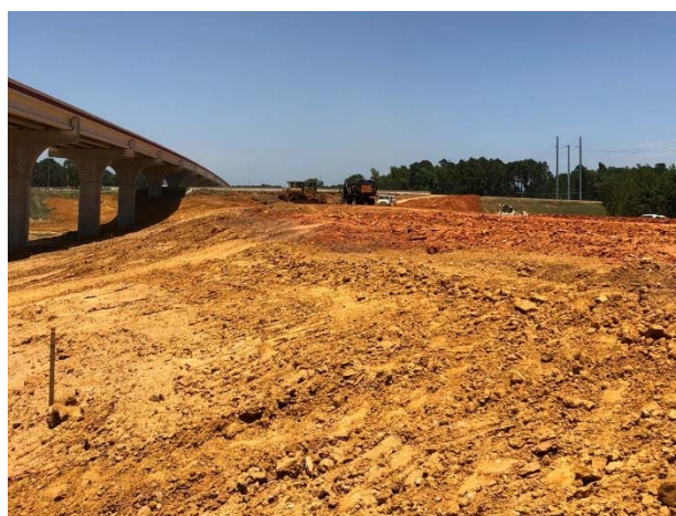
Embankment south of IH 20 for the northbound exit ramp
