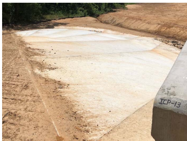
Concrete rip rap construction at Davis Branch Tributary
