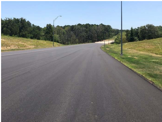
Final asphalt layer north of the Davis Branch bridge
