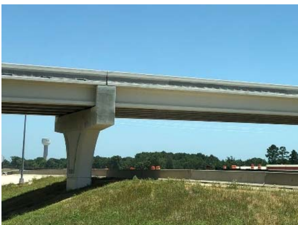
Concrete column partial painting at IH 20 main lane bridge
