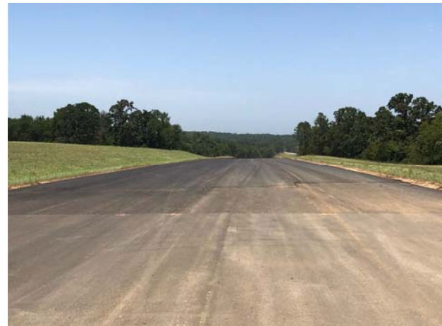
Final asphalt layer north of the FM 849 bridge
