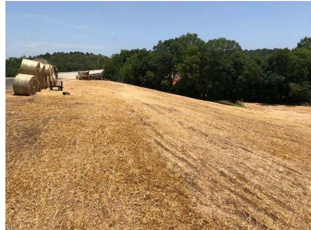
Fertilized, seeded and hay mulched side slopes between CR 431 and Stevenson Branch bridges
