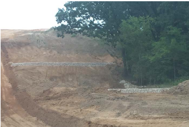
Rock Filter Dams between CR 4118 and CR 431 near culvert No. 5
