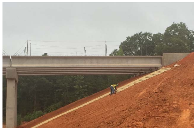
Hay mat installation at CR 431 bridge abutment
