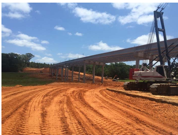
Completed beam placement at the CR 431 bridge
