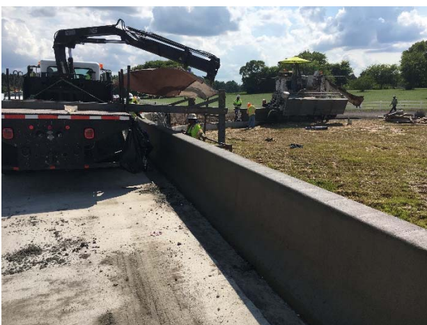
Installation of concrete traffic barrier at the approach of the FM 849 bridge
