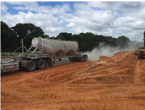
Cement treatment of subgrade at FM 16
