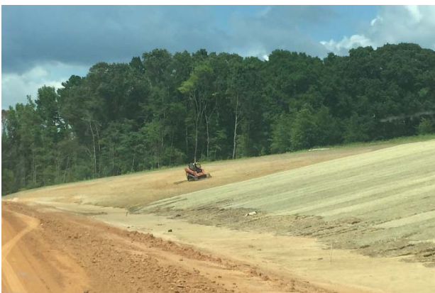
Topsoil and compost on backslopes between Davis Branch and Davis Branch Tributary
