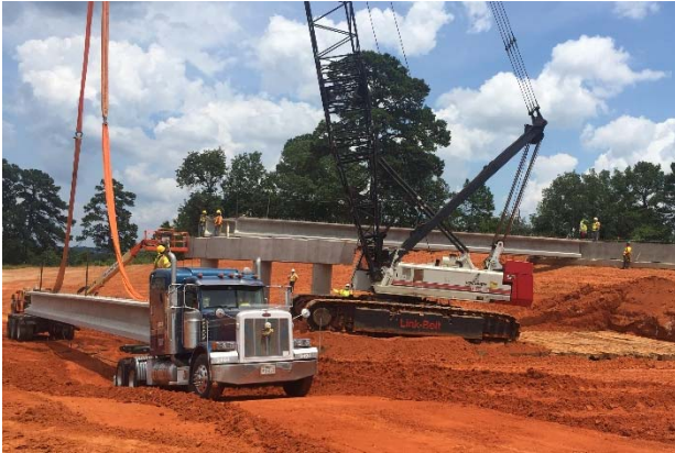
Beam placement at the CR 4118 bridge
