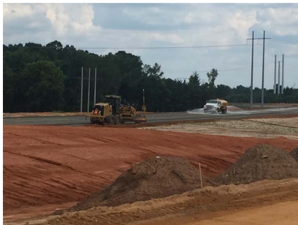
Placement of flex base for Toll 49 main lanes north of IH 20
