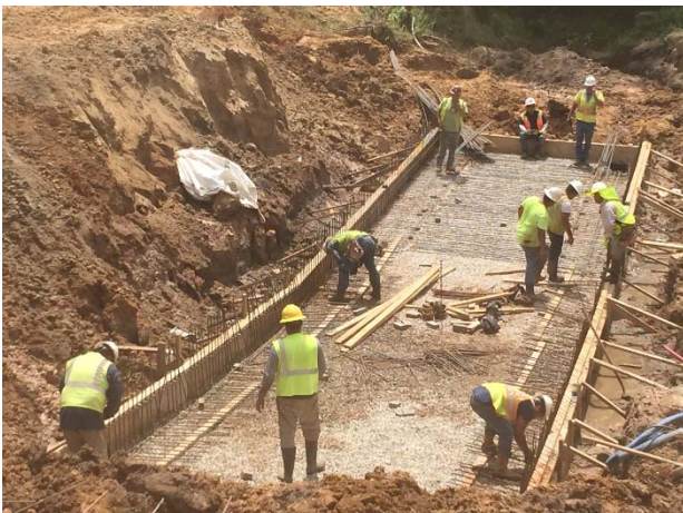
Culvert No. 16 construction south of FM 849
