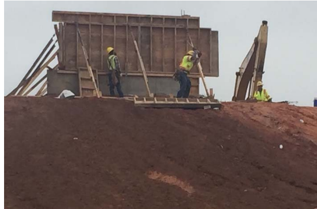
Building forms for CR 431 bridge abutment
