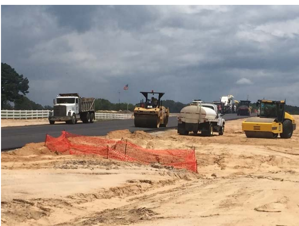
Placement of hot mix asphalt on the western side of realigned FM 849 pavement
