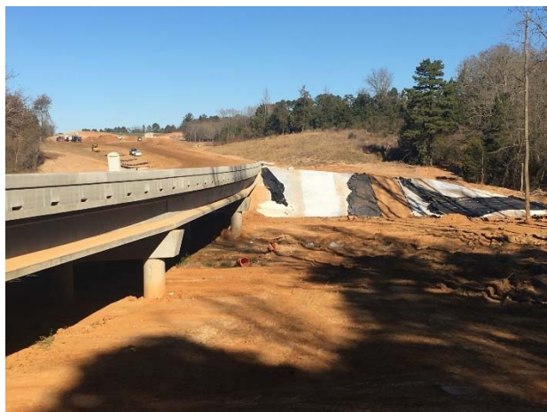
Rip rap construction at Davis Branch bridge abutment
