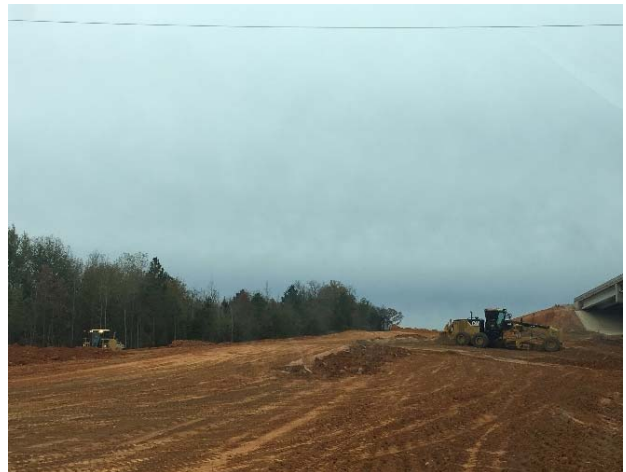
Embankment south of IH 20 for the northbound exit ramp from Toll 49 to IH 20
