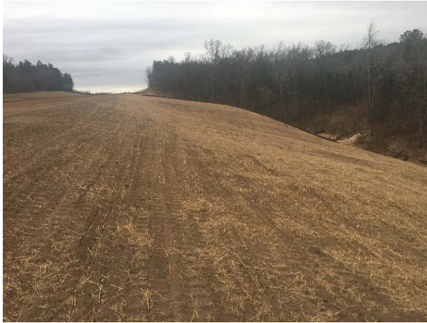
Hay mulch on roadway side slope south of Stevenson Branch near Culvert No. 8
