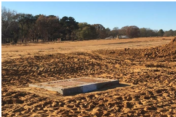
Storm sewer area inlet south of FM 16
