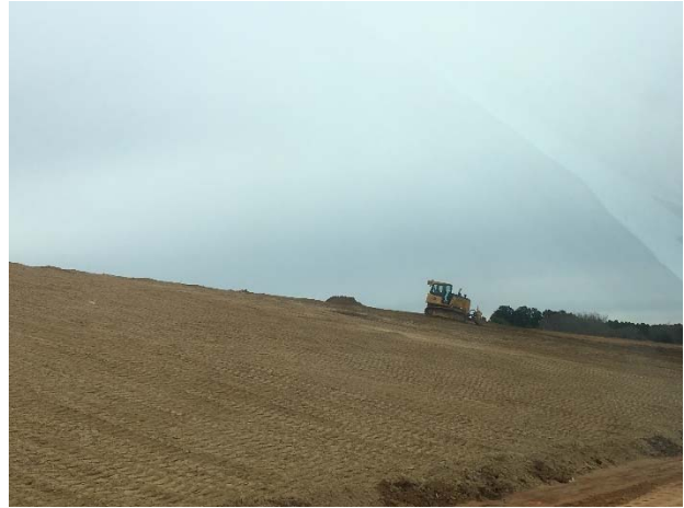
Installing top soil on side slopes south of FM 16
