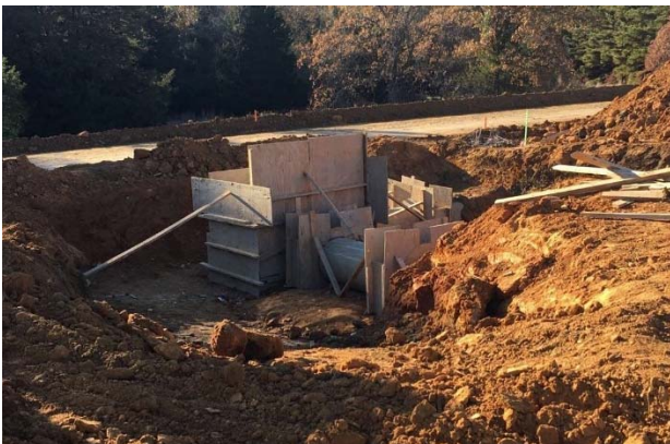
Drop inlet installation for storm sewer south of FM 16
