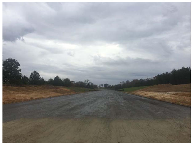
Roadway primed between IH 20 and existing FM 849
