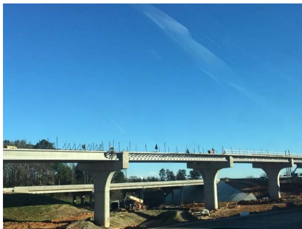
Installing overhang forms at IH 20 mainline overpass
