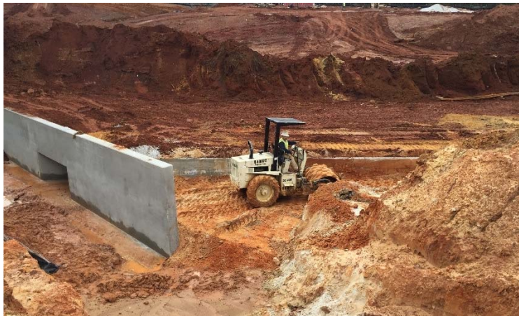
Backfilling at cross culvert #7 headwall (north of FM 16)
