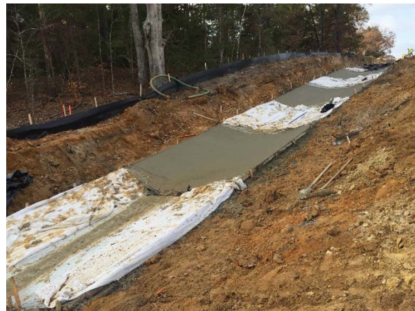
Concrete riprap construction near cross culvert #12 (south of FM 16)
