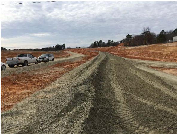
Flexible base grading and compaction south of US 69
