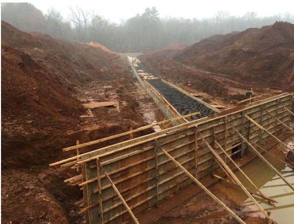
Construction of cross Culvert #7 concrete headwall (north of FM 16)
