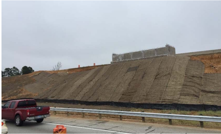
Soil retention blankets at IH 20 northbound ramp bridge abutment
