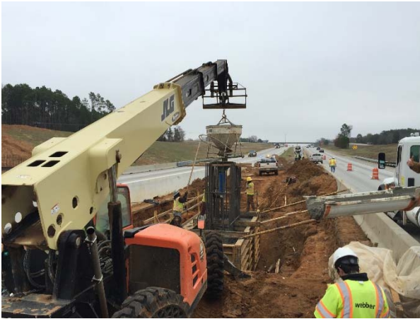
Footing construction for main lane overpass at IH 20
