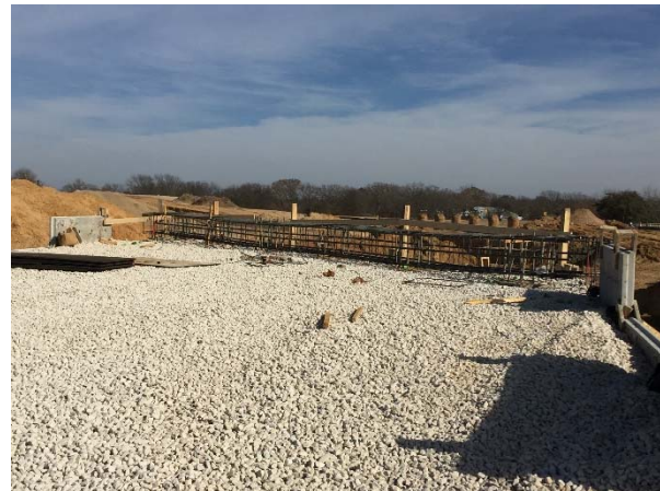
Rebar for cap construction at FM 849 underpass (Abutment No. 4)
