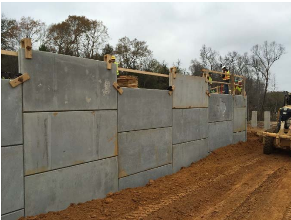
MSE wall construction at Davis Branch Tributary bridge (Abutment No. 4)
