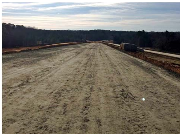
Flexible base installation south of FM 16
