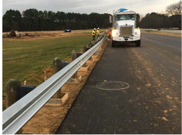
Installation of guardrail and construction of mow strips approaching the FM 849 bridge
