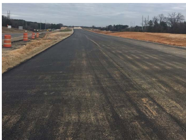
Asphalt paving south of IH 20
