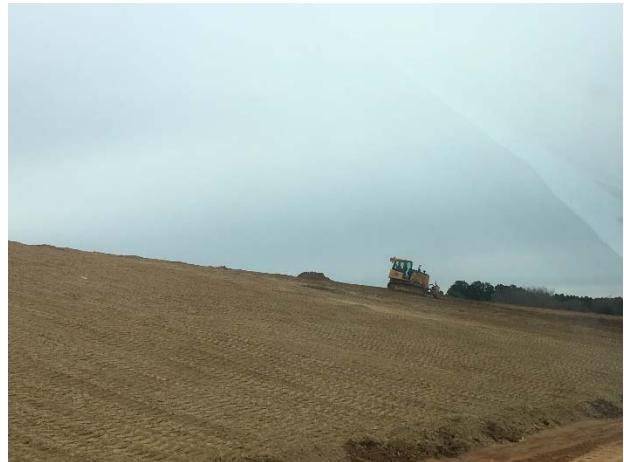
Installation of top soil on side slopes south of FM 16
