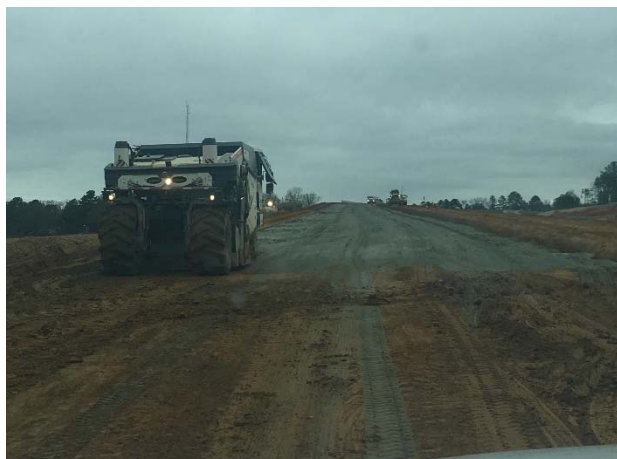
Cement subgrade treatment south of FM 16
