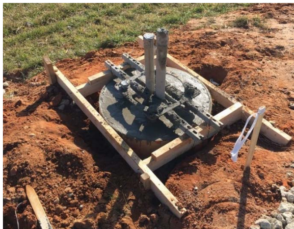
Drilled shaft for main lane gantry north of FM 16
