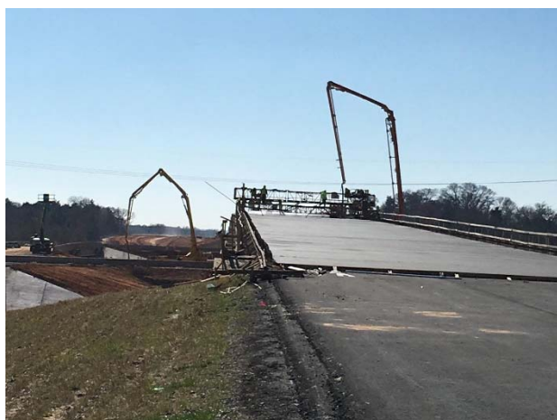
IH 20 main lane overpass bridge deck construction
