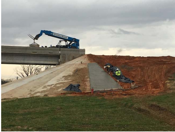
Construction of concrete rip rap at the FM 16 bridge abutment
