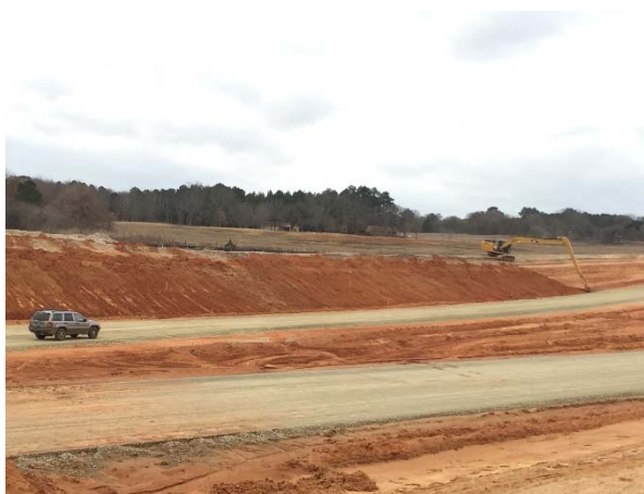
Grading of backslopes between US 69 and CR 4118
