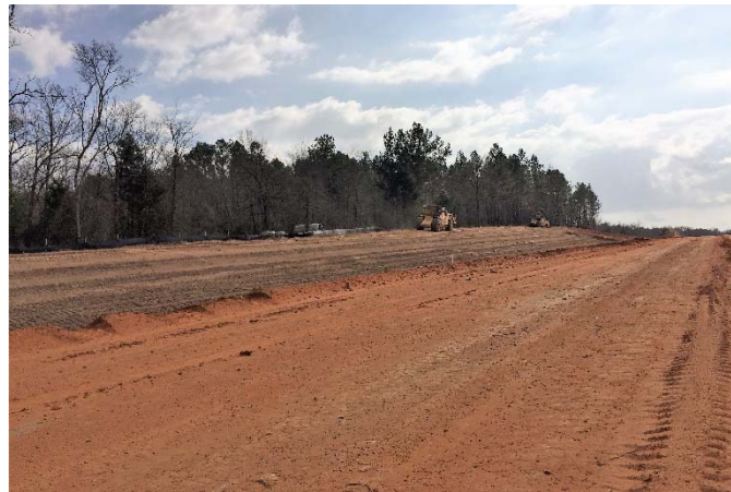
Placement of topsoil on backslopes between US 69 and CR 4118
