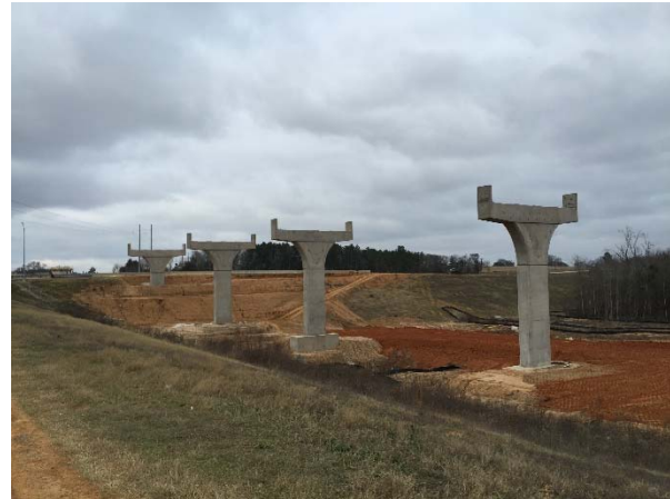
IH 20 main lane overpass bridge bents, southern side of IH 20
