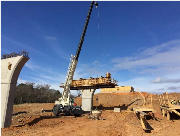
Cap construction for IH 20 main lane overpass, northern side of IH 20
