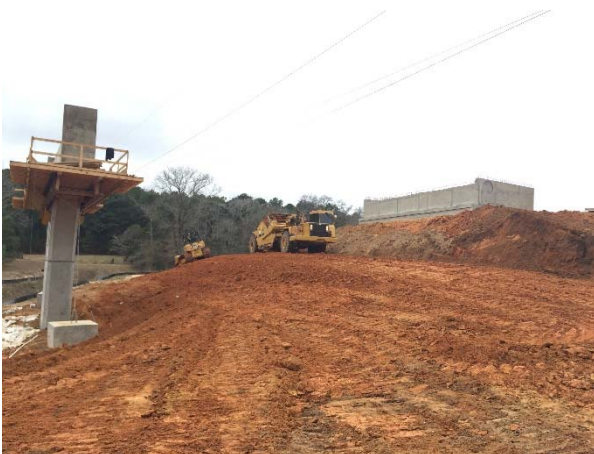
Embankment of IH 20 main lane bridge abutment
