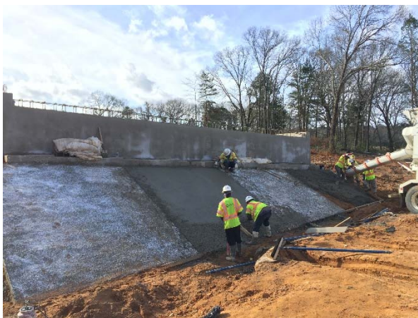
Concrete riprap construction at Davis Branch Bridge abutment No. 4
