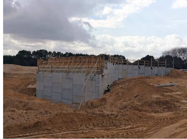
MSE wall construction at FM 849 underpass (Abutment No. 4)
