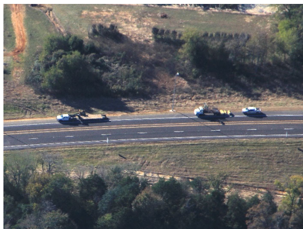
Raised pavement markers repair north of I-20
