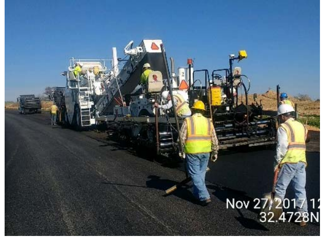
Placement of the first four inches of asphalt for the north bound ramp from IH 20
