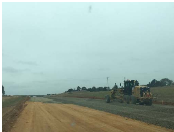
Flex base installation north of FM 849
