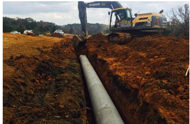
Reinforced concrete pipe south of FM 16
