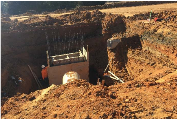
Drop inlets installation south of FM 16
