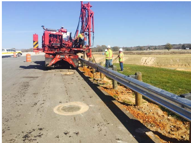
Installation of guardrail on FM 849 bridge approach
