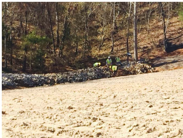
Rock filter dam maintenance at Cross Culvert No. 8, between Stevenson Branch and FM 16
