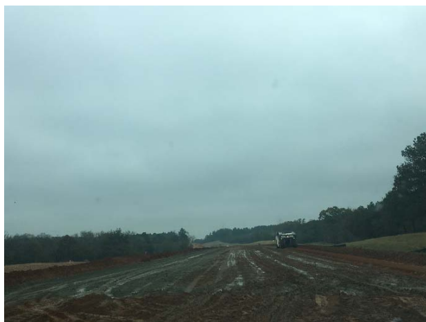
Cement treated subgrade north of FM 16
