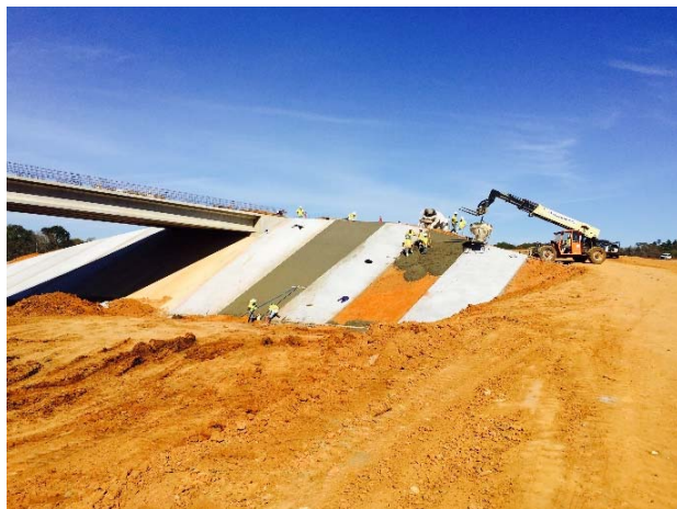
Rip rap installation at Stevenson Branch bridge abutment
