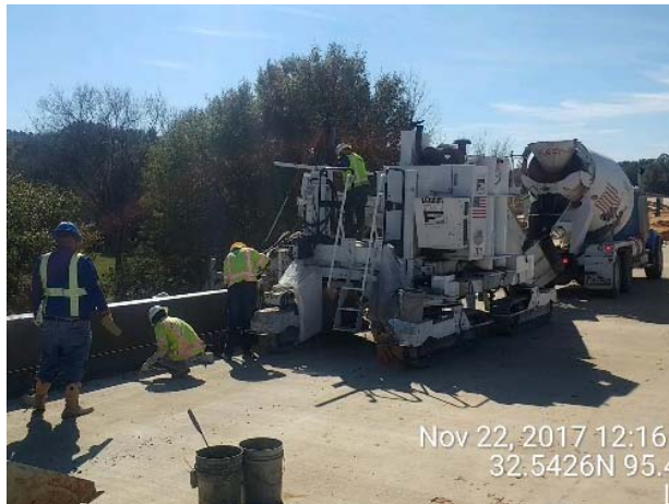
Concrete bridge rail installation on CR 431 bridge
