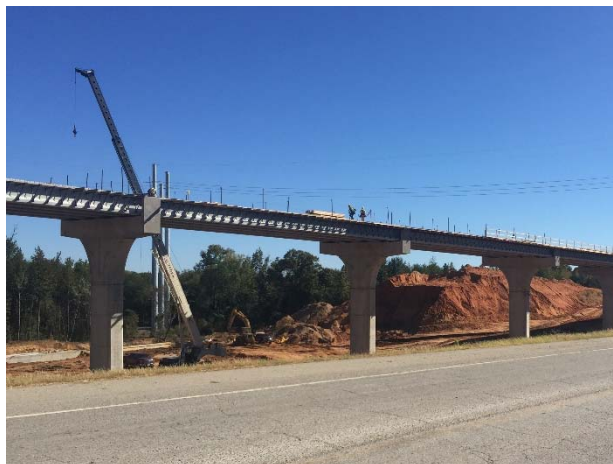
Installing deck panels and overhangs on IH 20
