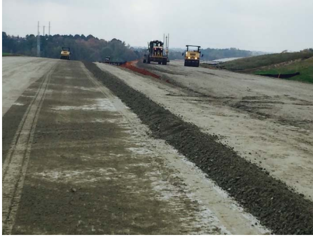
Installation of flex base north of IH 20
