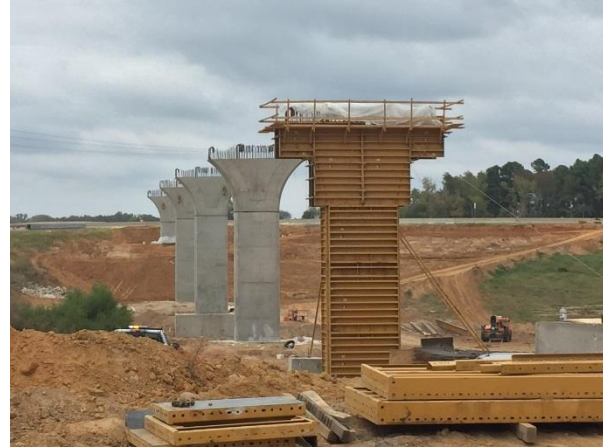
Flared column construction for main lane overpass at IH 20
