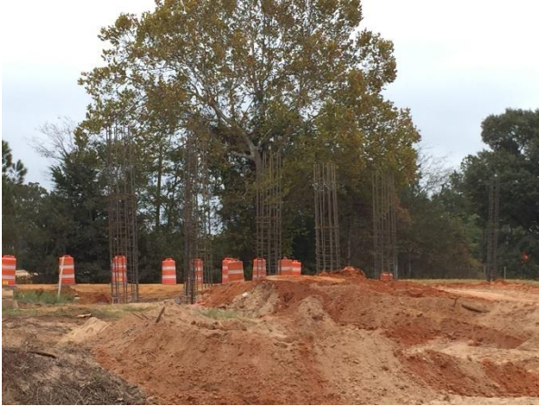
Drill shafts for bridge abutment at FM 16 overpass
