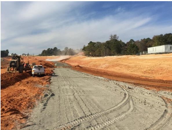
Main lane cement subgrade stabilization south of US 69
