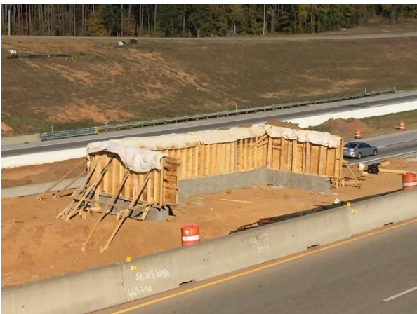
Bridge abutment for main lane overpass at IH 20
