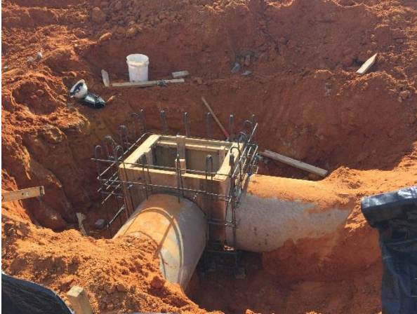
Minor culvert inlet construction at US 69 SB entrance ramp
