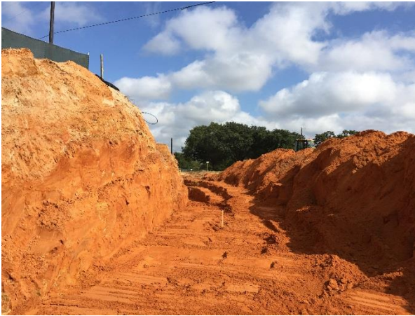
Excavation for temporary drainage (at future US 69 southbound entrance ramp)
