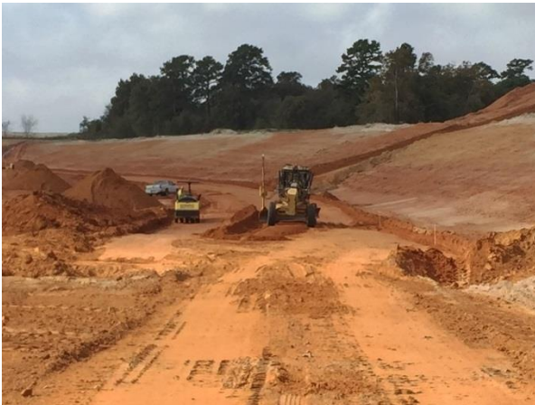
Final grading for roadway subgrade south of US 69
