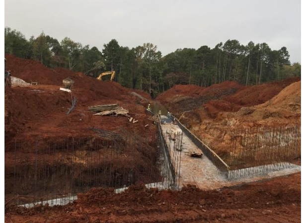
Cross Culvert #7 concrete box culvert construction (north of FM 16)
