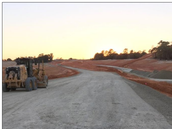
Flexible base at Toll 49 main lane and US 69 southbound entrance ramp
