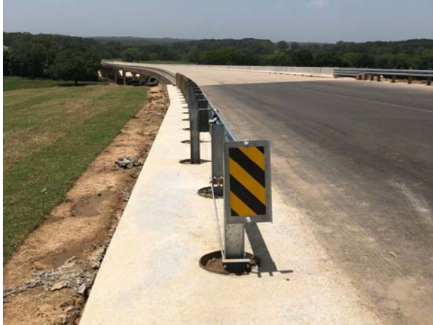
Guardrail installed on CR 431 bridge
