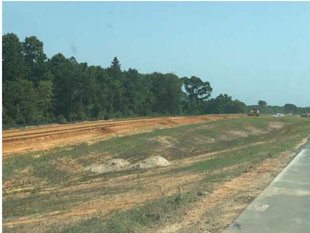
Cement treatment for northbound ramp
