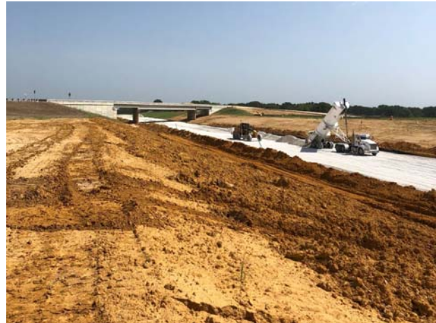
Placement of drainable pavement layer at FM 849
