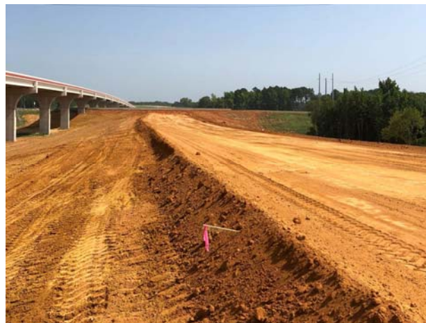
Embankment completed south of IH 20 on northbound ramp
