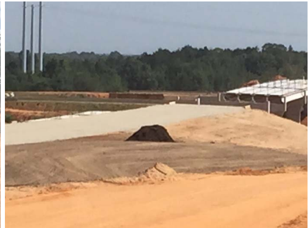
Flexible base for Toll 49 main lanes north of IH 20 bridge
