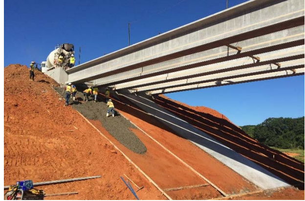
Placement of concrete rip rap under the Stevenson Branch bridge
