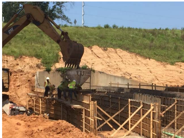
Concrete pour for Culvert No. 19 side walls at Long Brake Tributary
