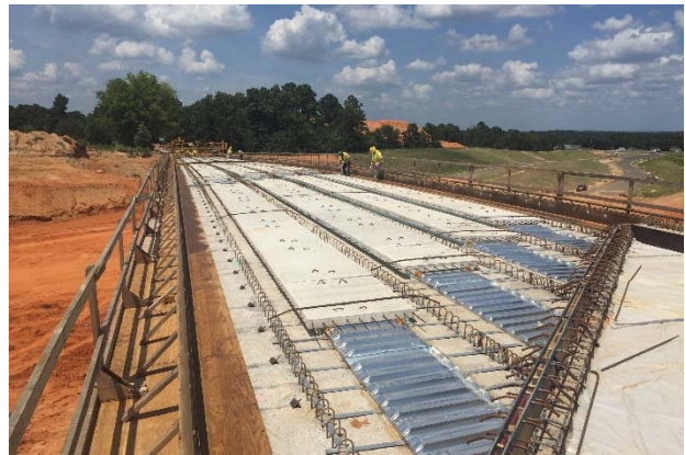
Permanent metal decking on the CR 431 bridge
