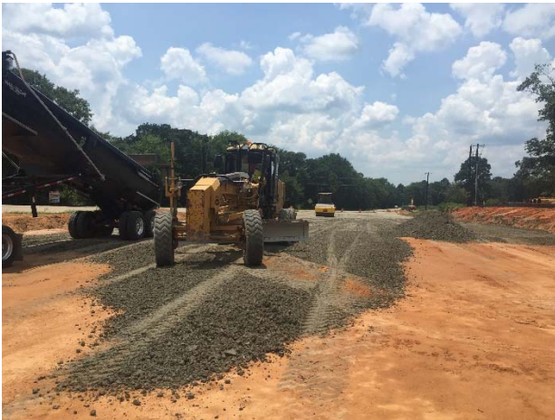
Flexible base placement at FM 16
