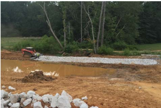
Rock filter dam maintenance and repair near Culvert No. 14
