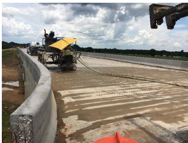
Surface grooving of concrete bridge deck at the FM 849 bridge
