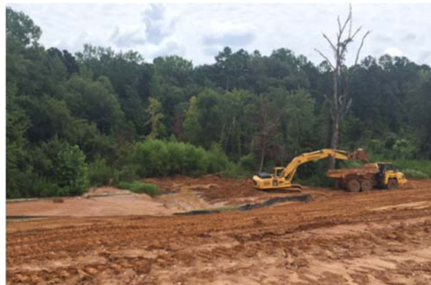
Sediment removal at Culvert No. 15 crossing
