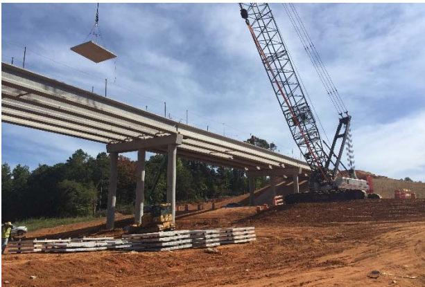
Concrete deck panel placement at the CR 431 bridge
