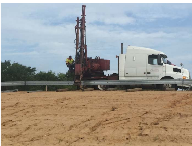
Installation of metal beam guard fence at the approach of the FM 849 bridge
