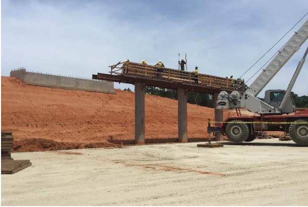
Building forms for the bent cap at FM 16 bridge
