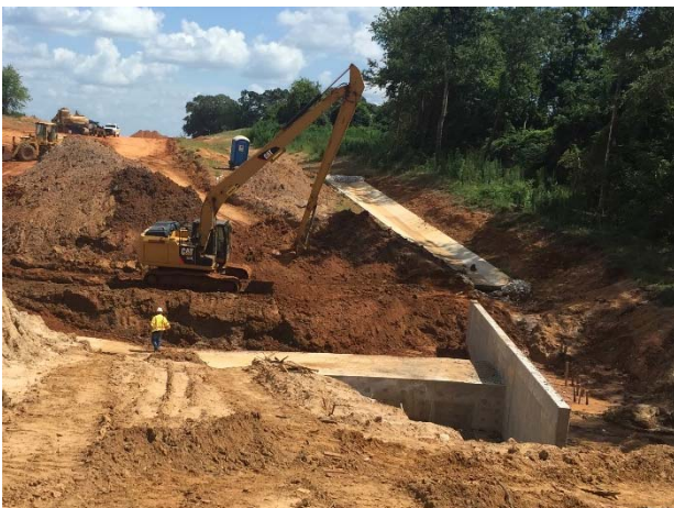
Backfill at Cross Culvert No. 16 south of FM 849
