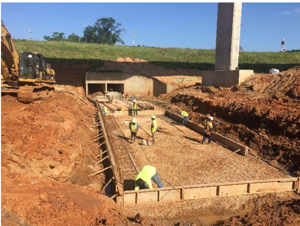
Culvert No. 19 footing forms north of IH 20 at Long Brake Tributary
