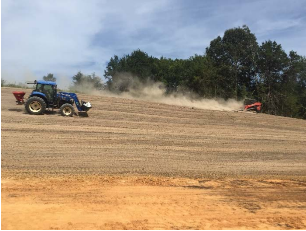
Permanent seeding on backslopes between Davis Branch and Davis Branch Tributary
