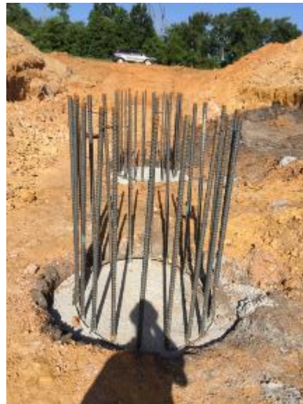
Drill shaft work at the future IH 20 overpass
