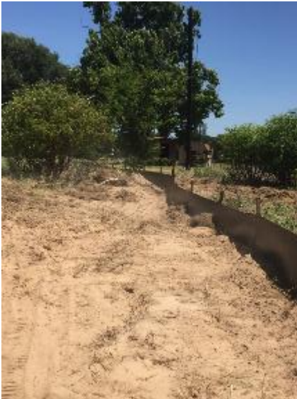
Silt fence installation near IH 20
