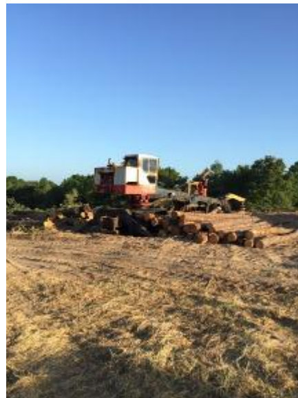
Clearing and grubbing near US 69
