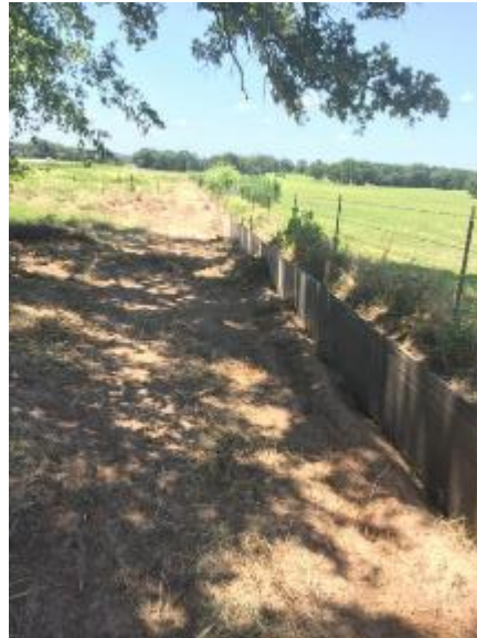
Silt fence installation near SH 110
