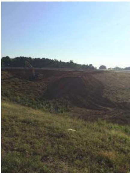
Clearing and grubbing near IH 20
