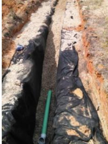
Underdrain installation at the future IH 20 southbound ramp
