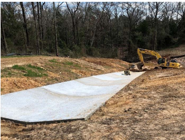
Concrete rip rap flume near Culvert No.16, south of FM 849
