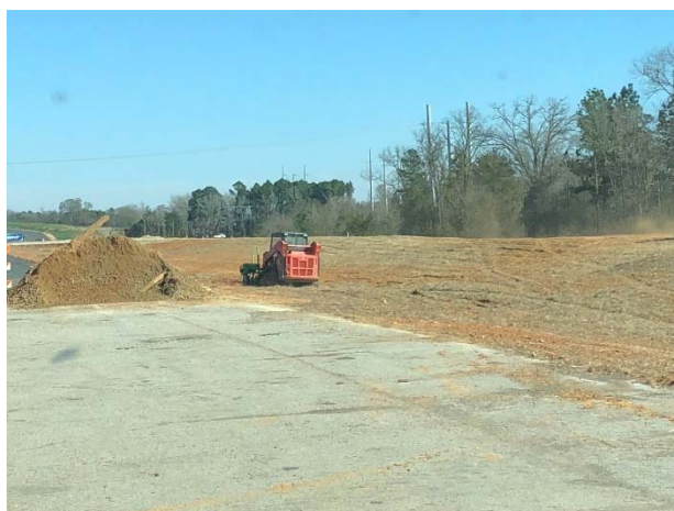
Topsoil and seeding south of existing FM 849
