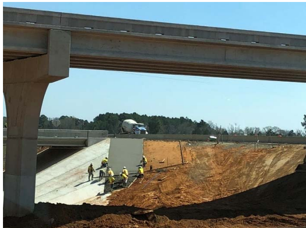
Concrete rip rap construction at the Northbound Ramp Bridge abutment at IH 20
