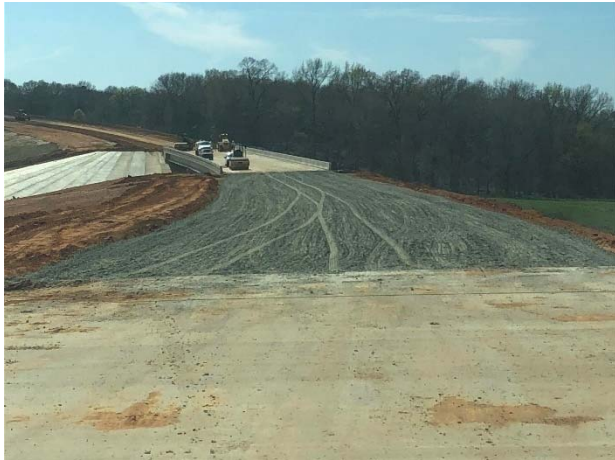
Flexible base installation between the CR 431 and Stevenson Branch bridges
