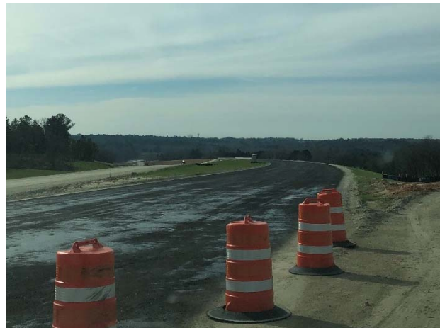
Primed flexible base north of FM 16 at the ramp tie-ins
