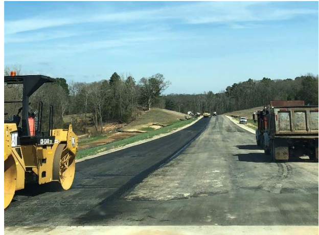
Asphalt paving south of Davis Branch Bridge
