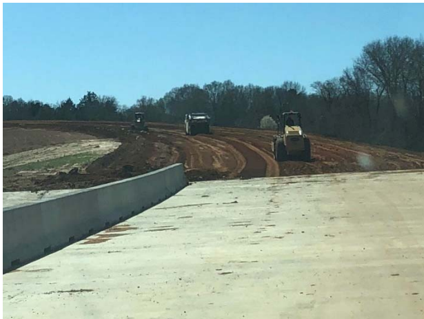
Preparing for cement treatment of the subgrade south of Stevenson Branch
