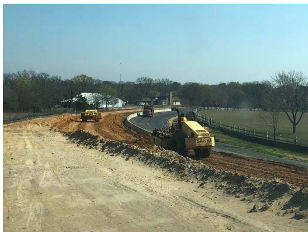
Embankment at FM 849 tie-ins
