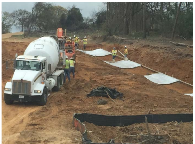
Concrete riprap construction near future cross Culvert No. 16 south of FM 849
