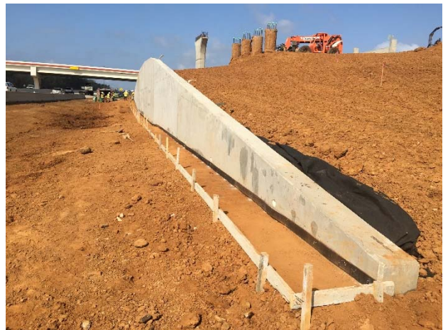
Cast-in-place retaining wall #5 at IH 20 northbound ramp overpass
