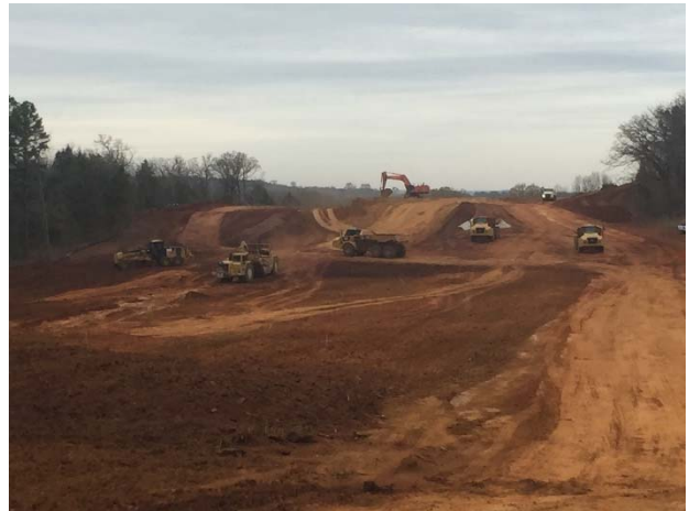
Excavation between Stevenson Branch and FM 16
