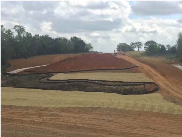
Soil retention blankets near future cross culvert No. 16 south of FM 849
