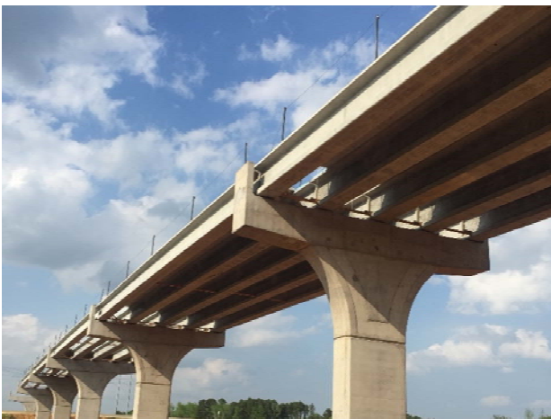
Deck panels at the IH 20 main lane overpass bridge
