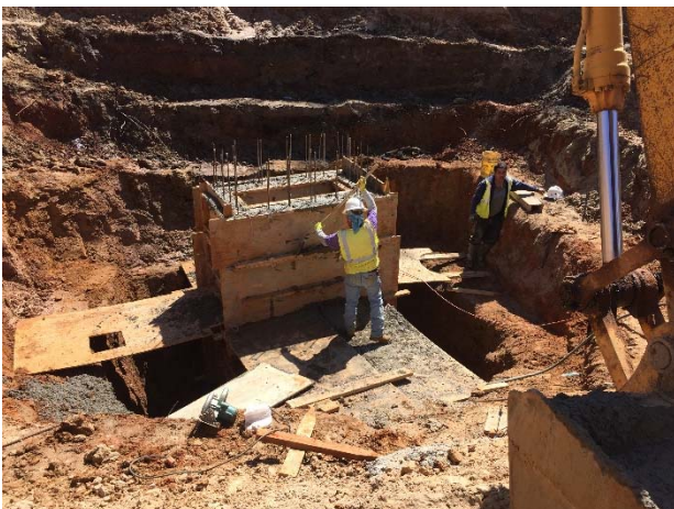
Drop intel at Culvert No. 15 near Davis Branch Tributary
