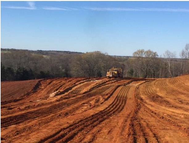
Compaction near Stevenson Branch
