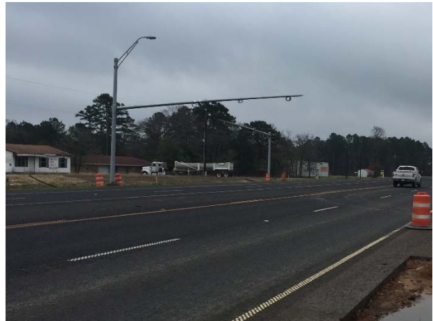
Signal pole installation at intersection with US 69
