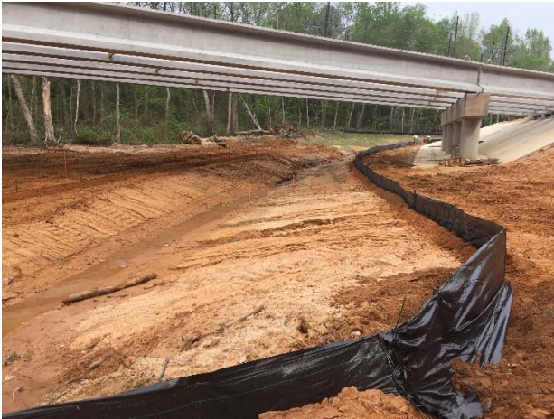
Bridge beams and silt fence at Davis Branch Tributary bridge
