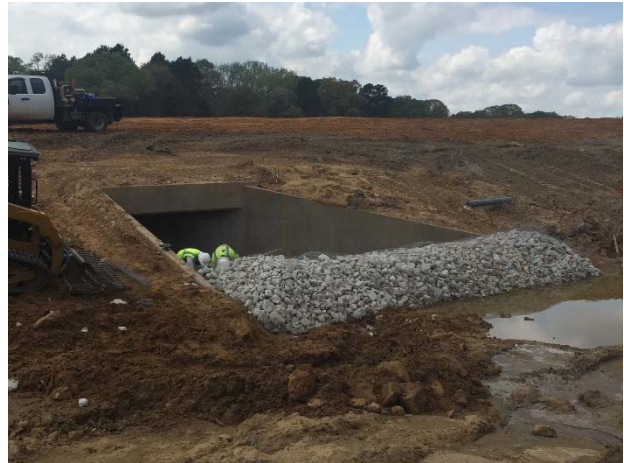
Rock filter dam at cross culvert No. 12 just south of FM 16
