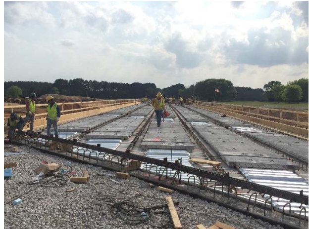
Metal decking and paneling at the FM 849 bridge
