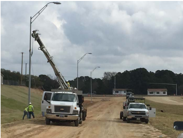
Light pole installation along just south of US 69
