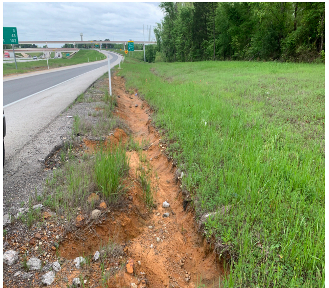
Figure 6: Erosion and Edge Drop-Off EB IH 20 Frontage
