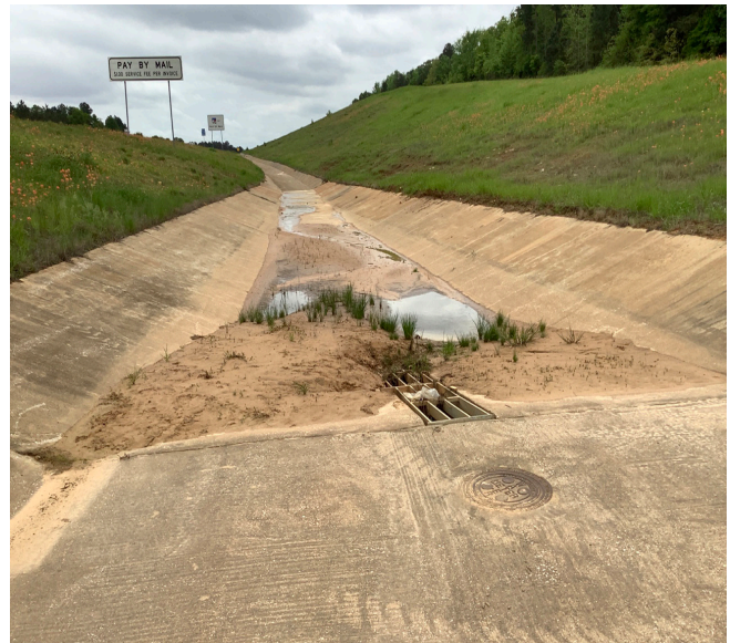
Figure 13: Hazmat Trap Silted Up
