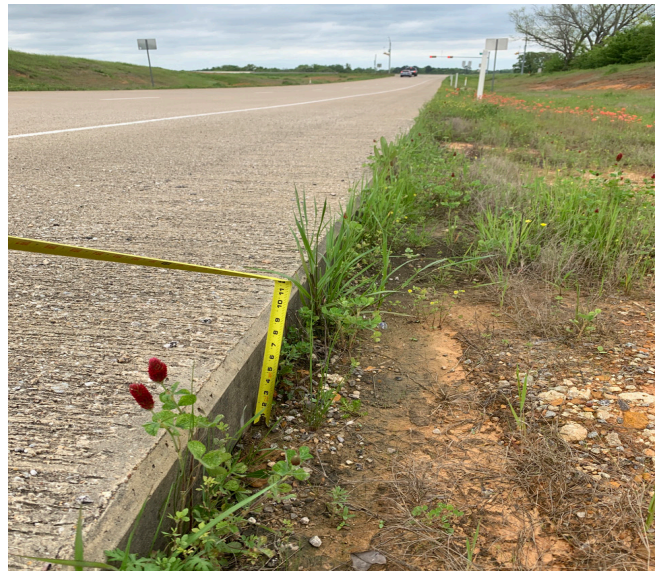
Figure 5: Edge Drop-Off NB SH 64 Off-Ramp
