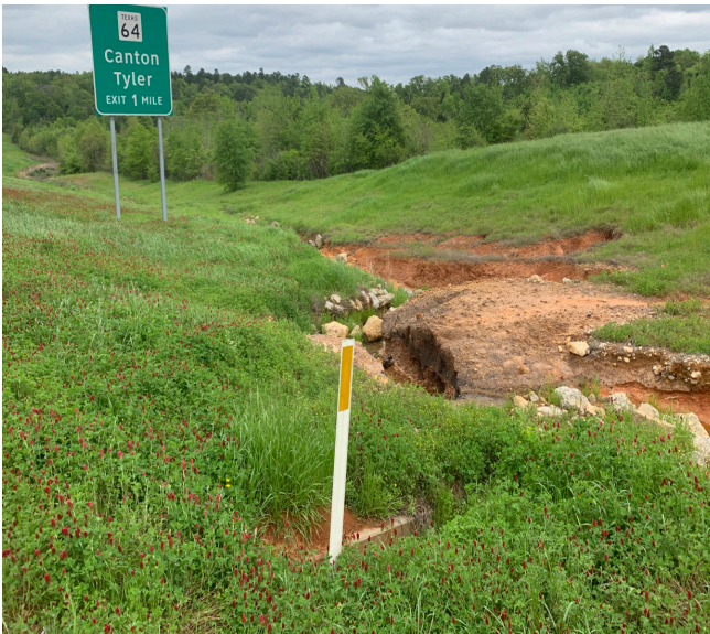
Figure 16: Ditch Erosion
