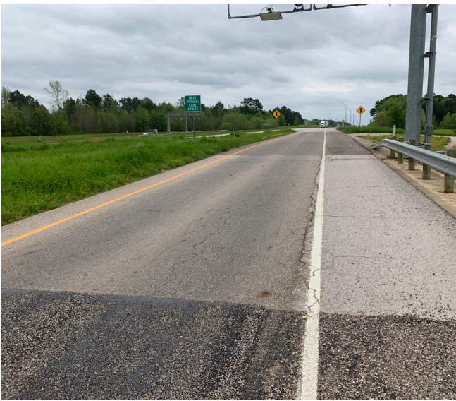
Figure 2: Pavement Cracking on SB SH 64 On-Ramp
