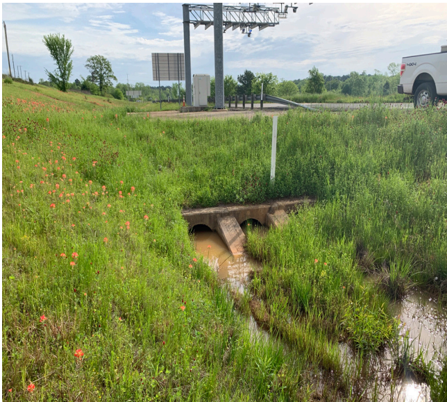
Figure 12: Structure Silted Up
