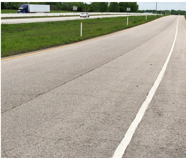
Figure 4: Pavement Cracking EB IH 20 Frontage
