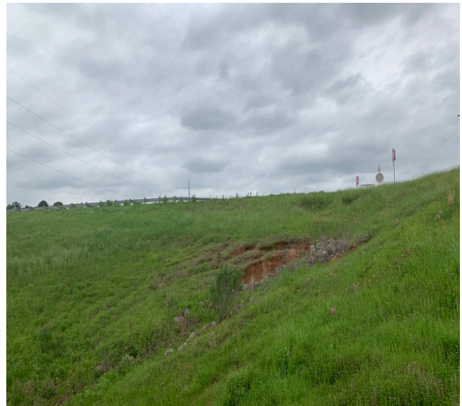
Figure 14: Slope Erosion
