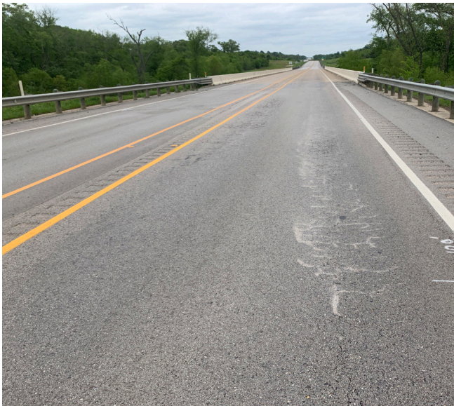
Figure 3: Pavement Cracking on NB Mainlane
