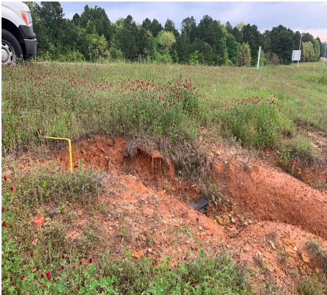
Figure 15: Slope Erosion
