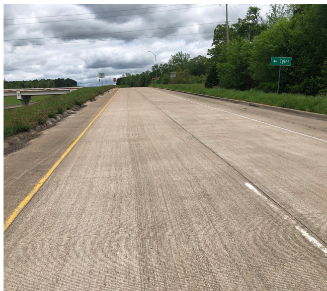
Figure 9: Faded Striping
