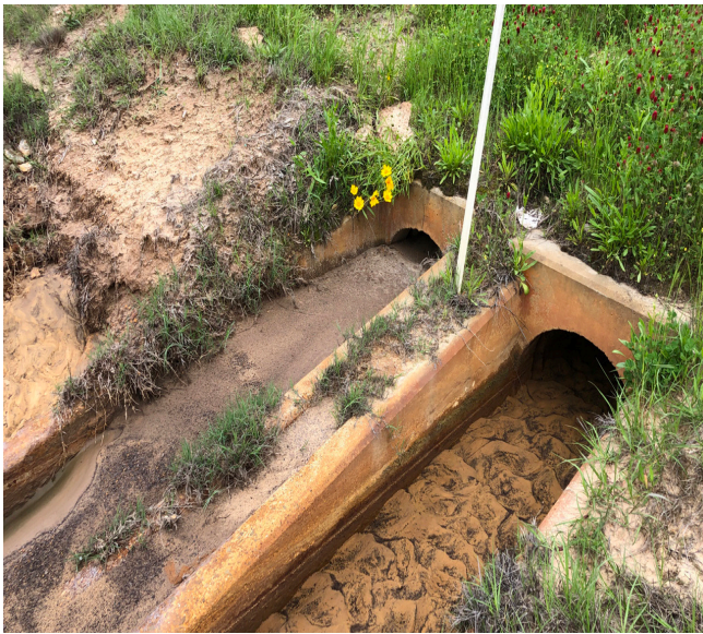
Figure 11: Culvert Partially Blocked
