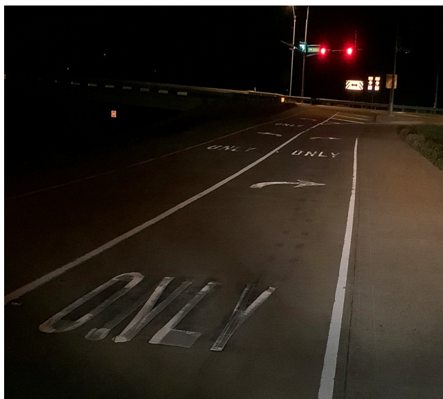
Figure 10: Faded Striping
