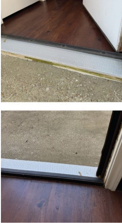
Transition at emergency exit is higher than the ¼" or ½" max allowed by TAS on interior and exterior sides (below left and middle)
