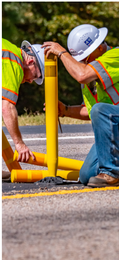
Installation of new electronic delineators
