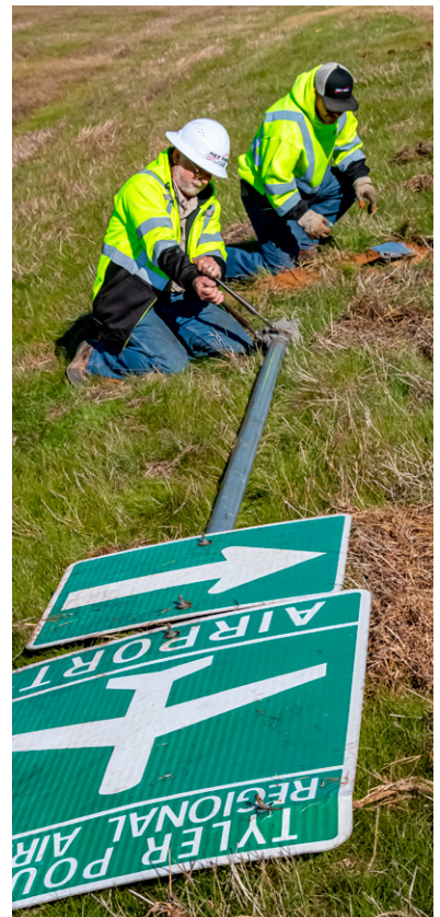
Installation & maintenance of permanent signage
