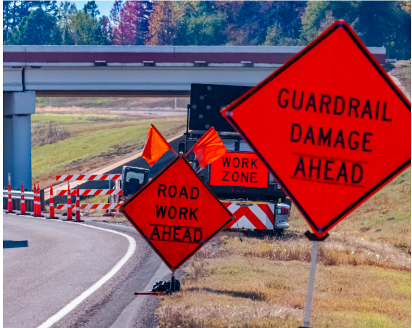
On-going road safety maintenance
