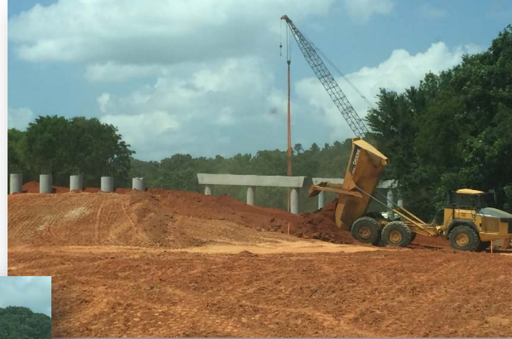
Earthwork: embankment.
