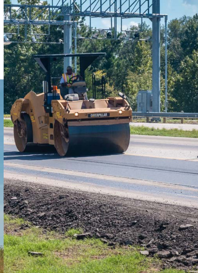
Steel drum and pneumatic rollers compacting new pavement inlay.
