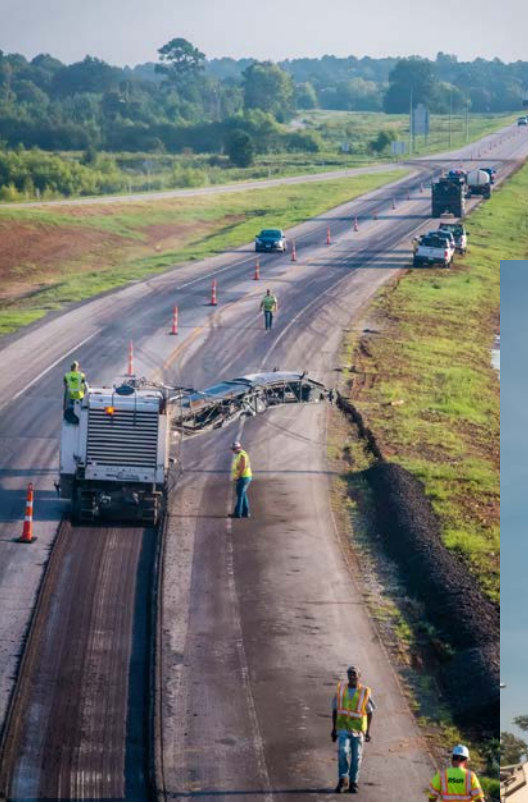
Depositing milled pavement along the shoulder.
