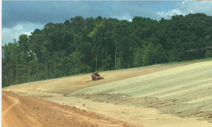
Erosion Controls: topsoil and seeding.
