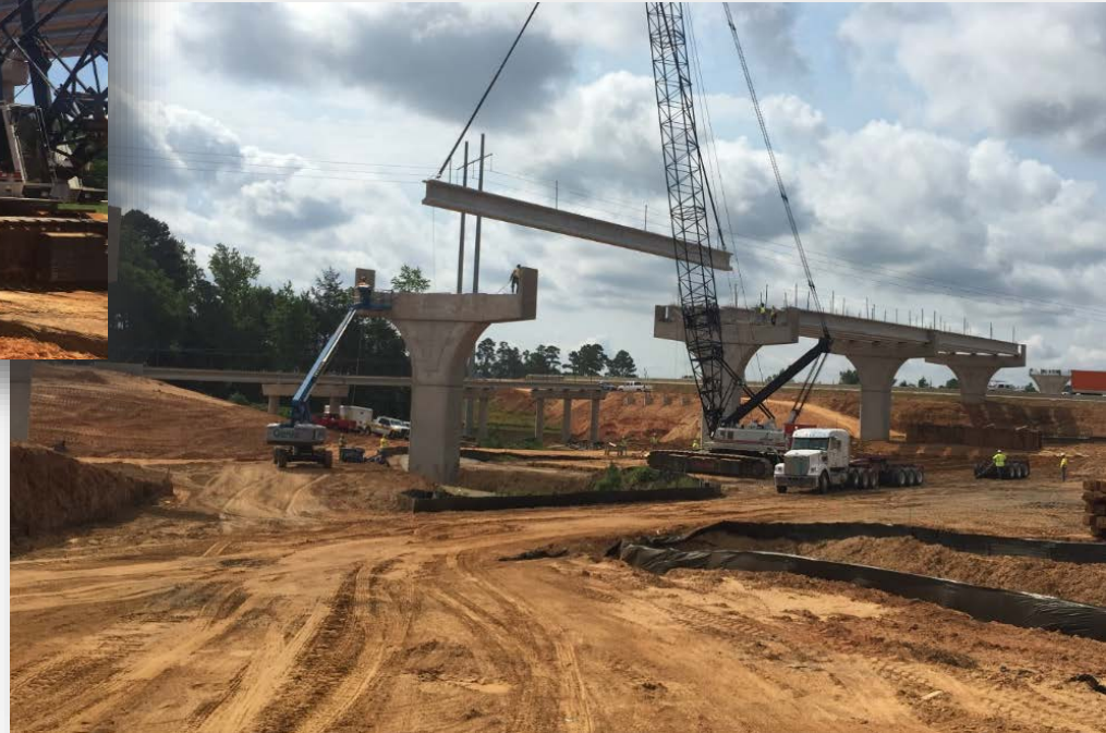
Bridges – I20 main lane and long brake tributary bridge beams.
