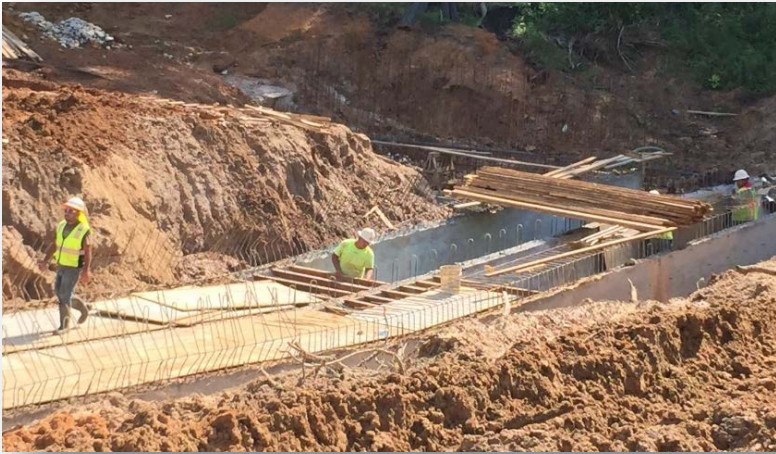
Drainage: culvert construction.
