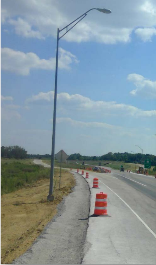
Widening – adding flexible base.
