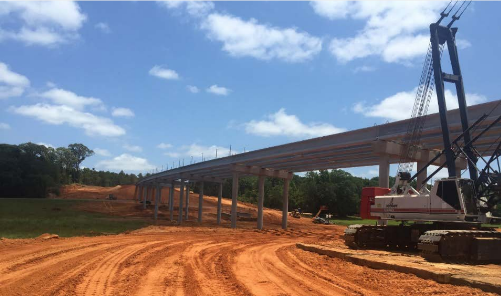
Bridges: beam placement.
