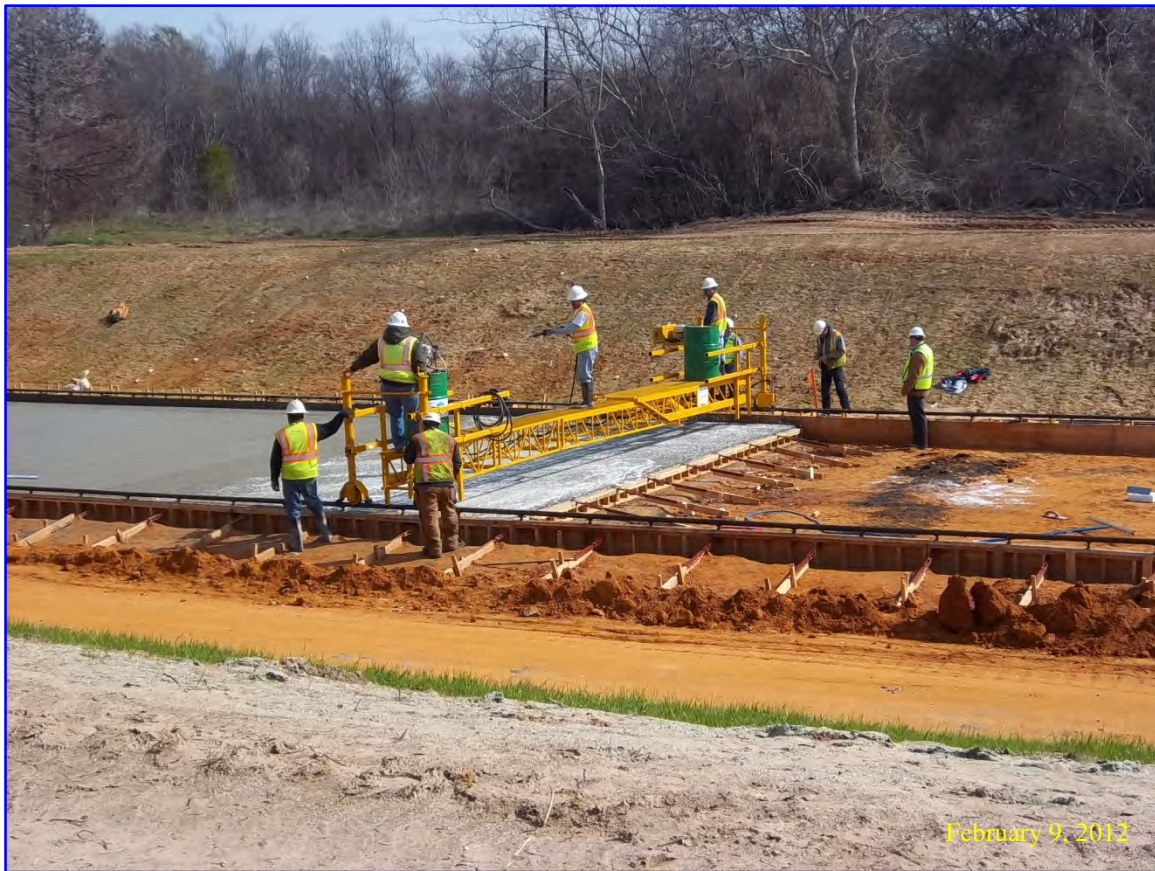
SH 64 Concrete Ramp Curing
