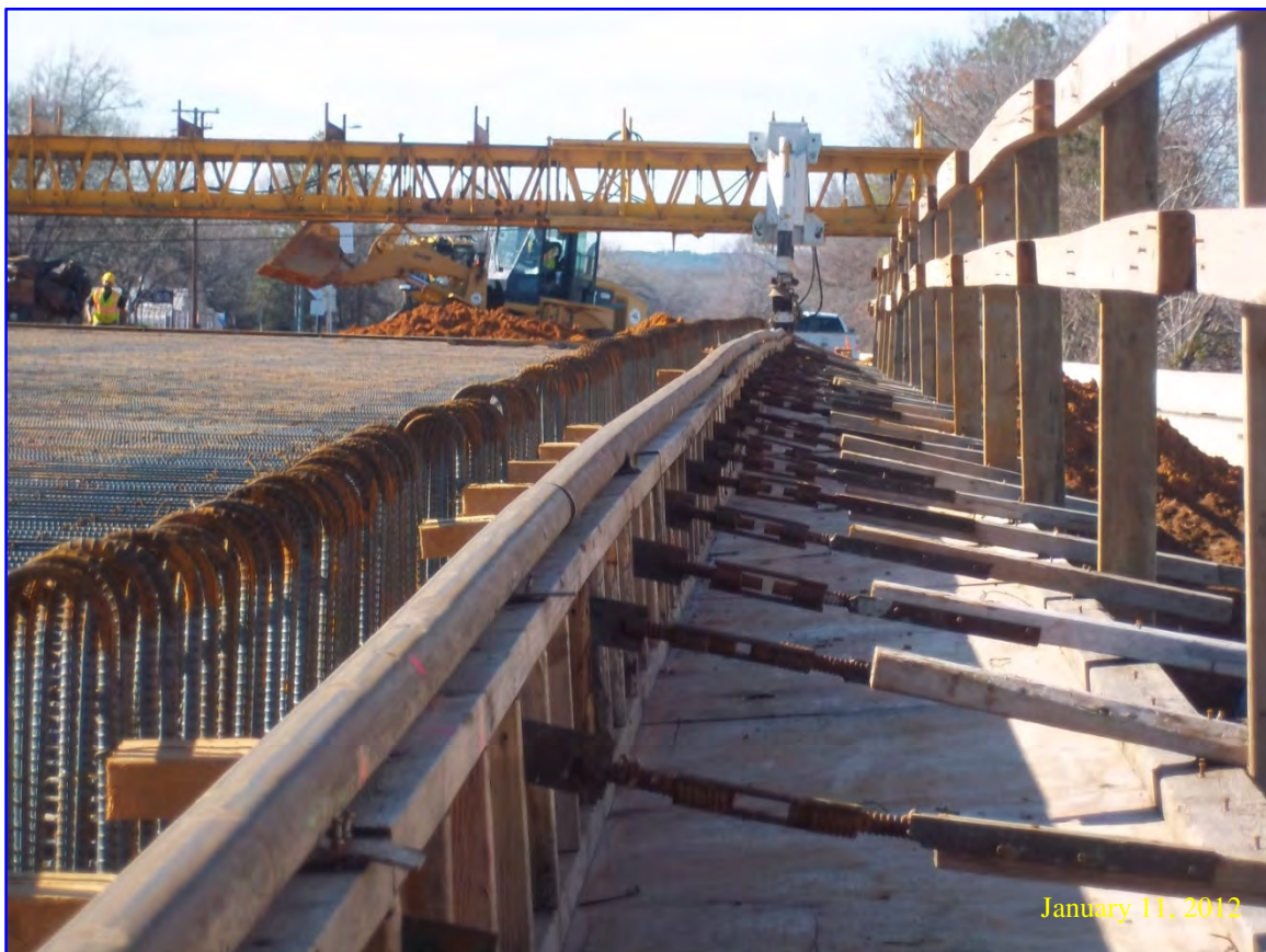
SH 64 Bridge Deck Steel and Screed
