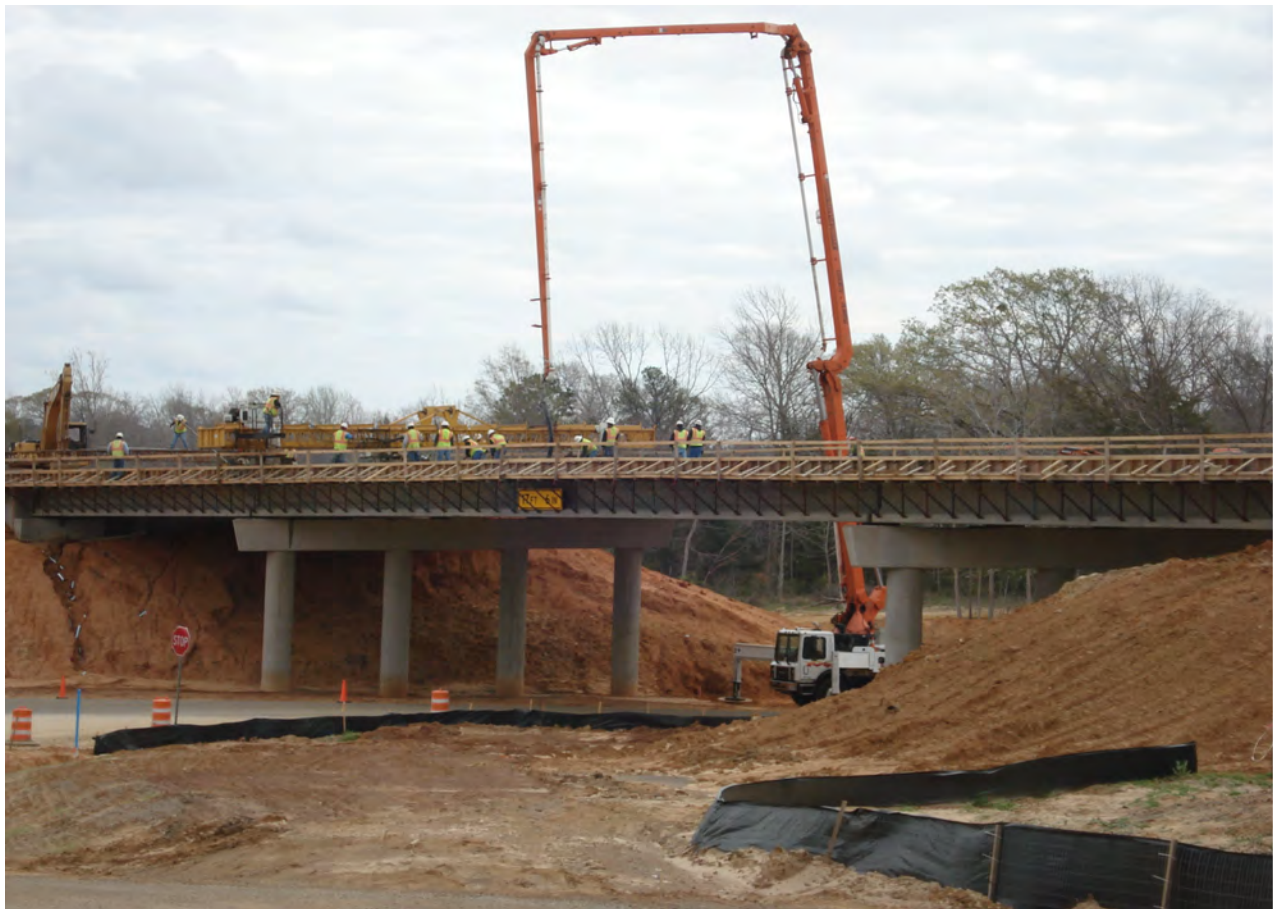
Bridge Deck Construction at SH 724
