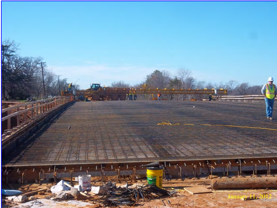
SH 64 Bridge Deck Steel and Screed
