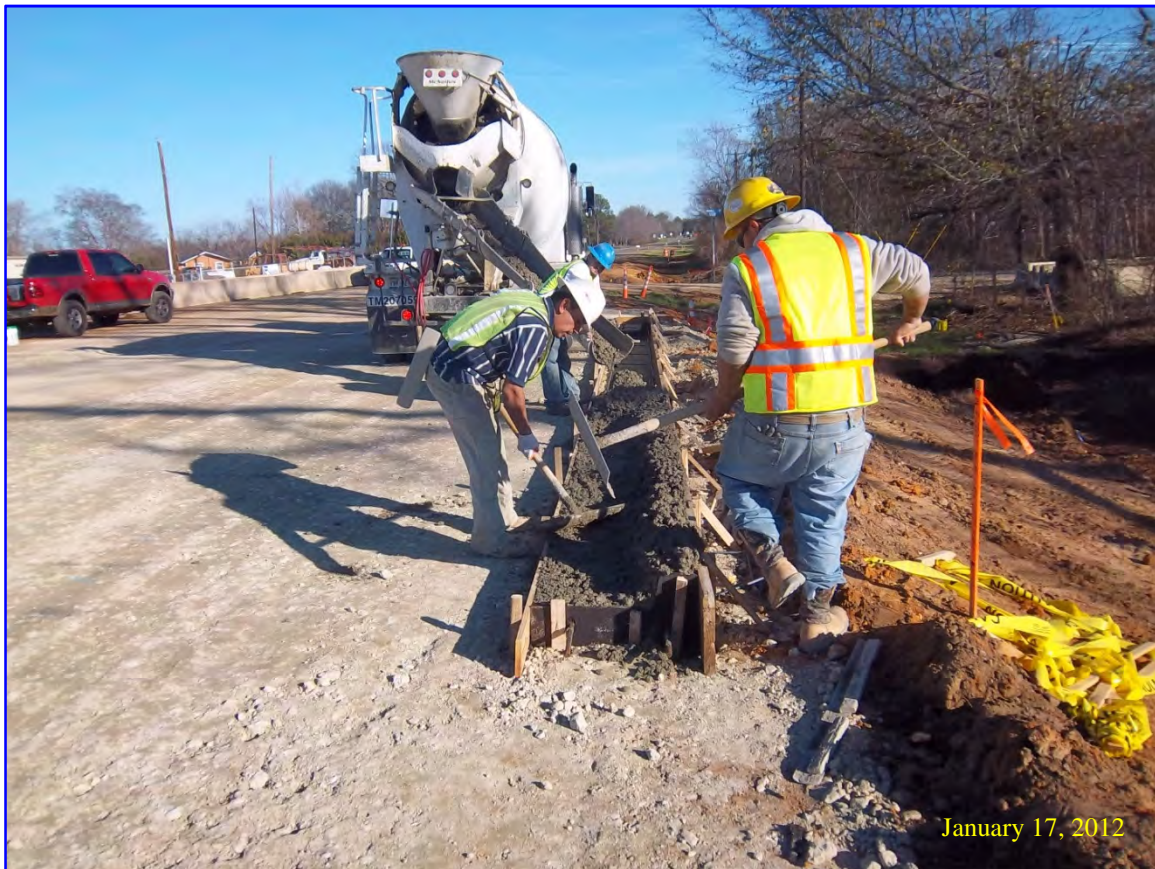
Concrete Curb for SH 64
