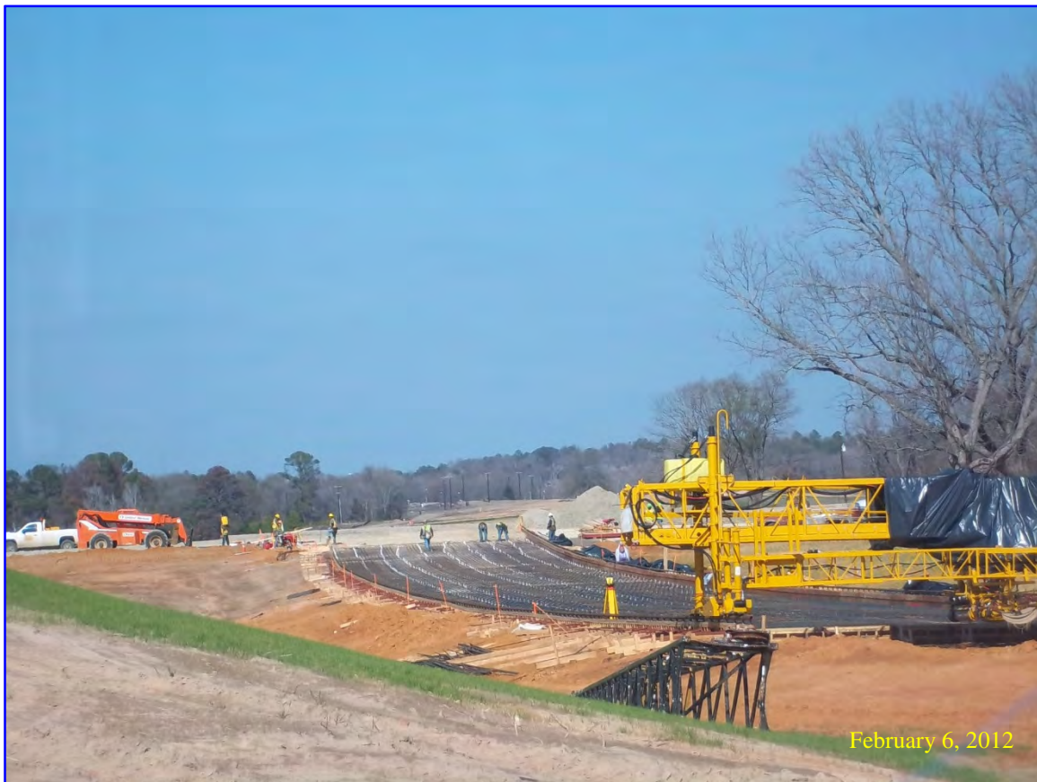
SH 64 Off Ramp Concrete Pavement Preparation
