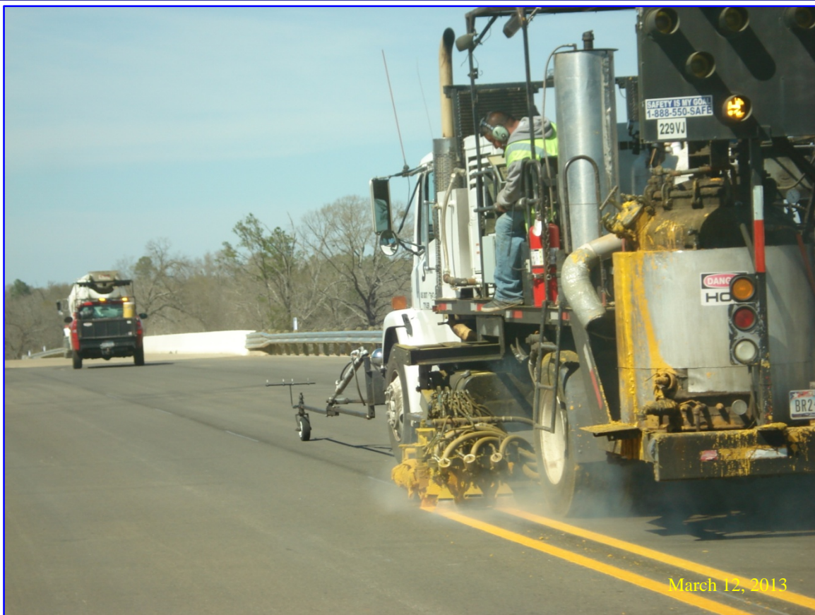
Striping Truck Striping Segment 3B of Toll 49 South of Prairie Creek
