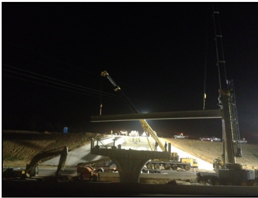
Figure 3: Nighttime Bridge Girder Installation at Toll 49 and I-20.
