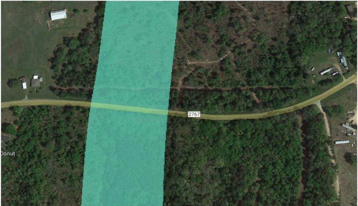
Figure 8a: 2019 aerial view of Development #8 prior to development (FM 2767) within Teal Adjusted route.
