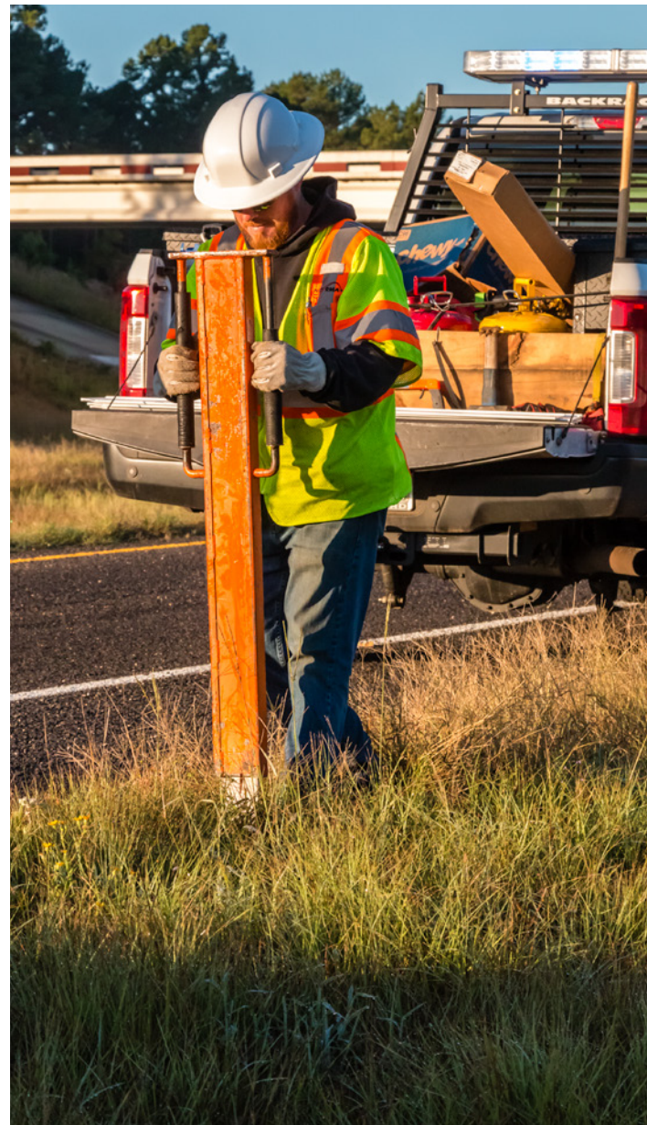
A NET RMA maintenance team member uses a driver to install a new delineator.
