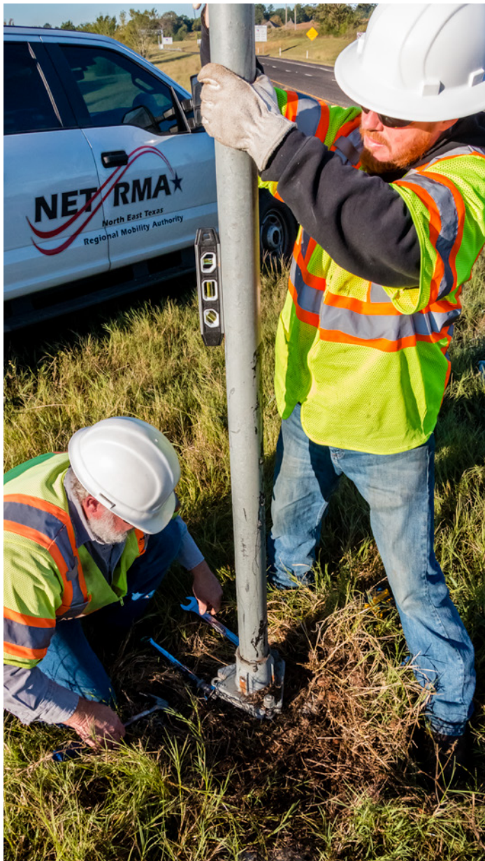
The NET RMA maintenance team ensures that signs are secure and level.
